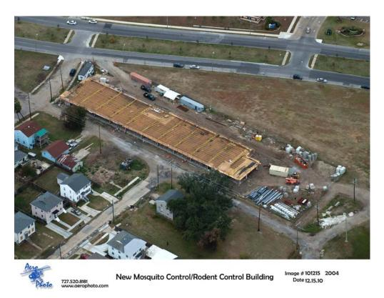
Figure 47. Second floor was framed to prepare for the pouring of the second floor.
