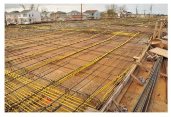
Figure 46. The cables were visible for pre-tensioning the slab for the second floor on 12/9/2010
