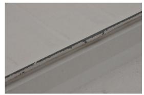
Figure 32. Paint scraped off the ridges of the roof panels caused by careless installation.
