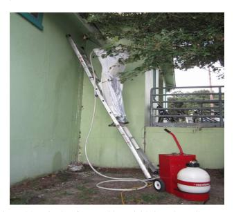
Figure 34. Injecting foam and insecticide into the wall at Stallings playground.
