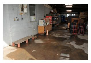
Figure 8. The waterline showed that approximately six to eight inches of water entered the middleshop.
