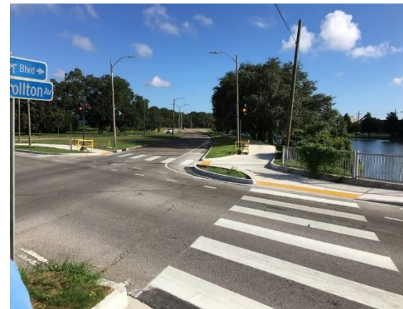
Figure 8. Completed installation of curb ramps and high visibility
