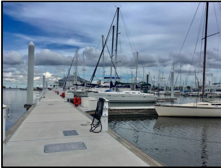
Figure 6: New Floating Docks and Slips
