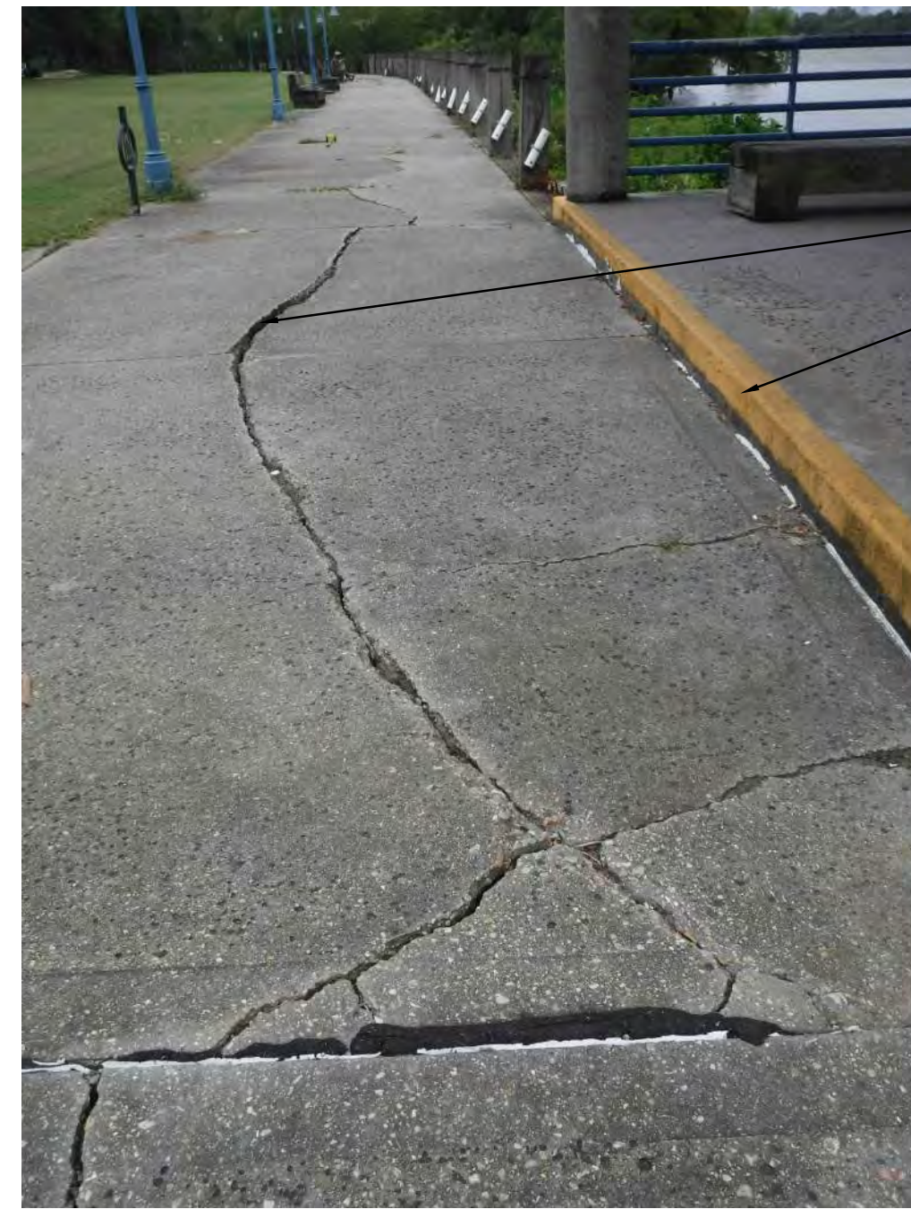
TOPS OF TIMBER BOLLARDS ARE ROTTEN, TYP. SOME ARE LOOSE TIMBER BULKHEAD SUBSIDING DOWN BANK SLOPE, TYPICAL CONDITION MISSING BOLLARD CRACK ALONG SIDEWALK
