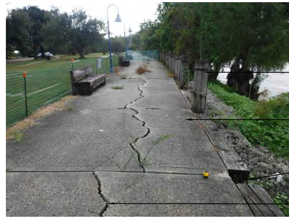
TOPS OF TIMBER BOLLARDS ARE ROTTEN, TYP. SOME ARE LOOSE TIMBER BULKHEAD SUBSIDING DOWN BANK SLOPE, TYPICAL CONDITION MISSING BOLLARD CRACK ALONG SIDEWALK
