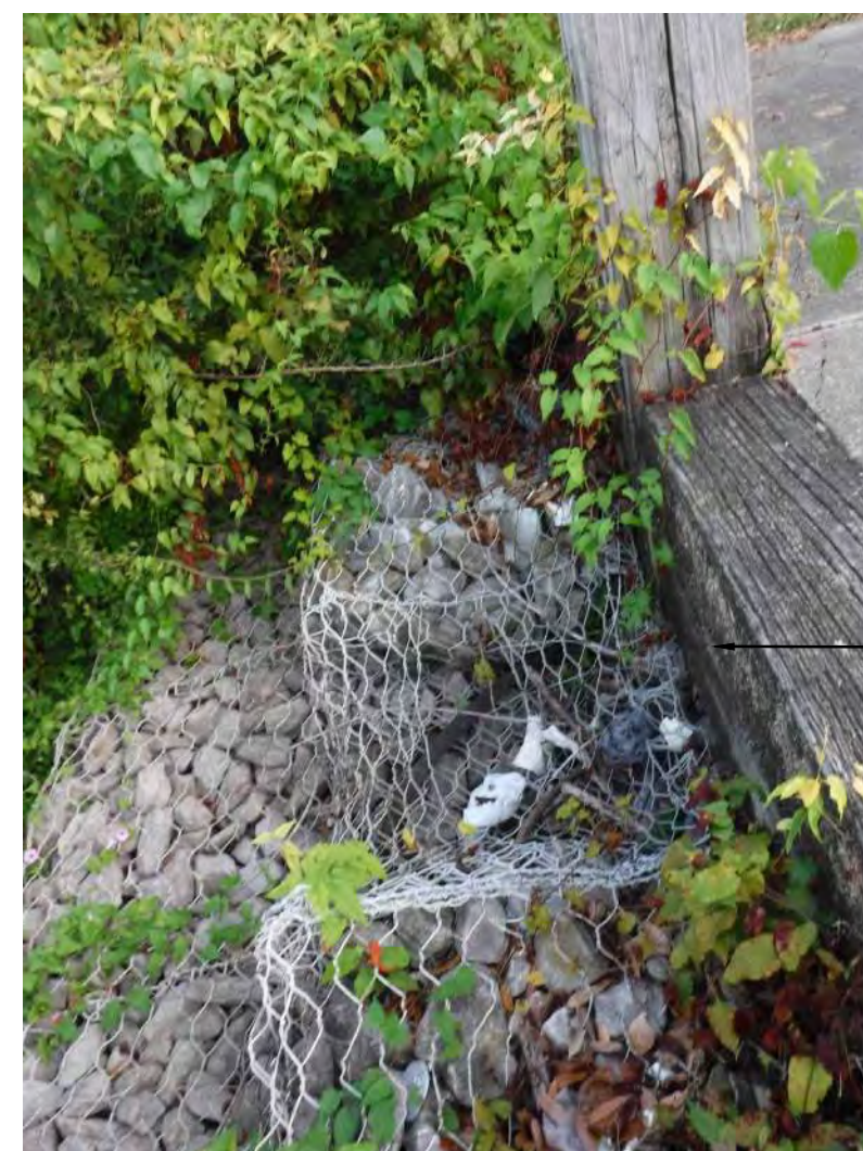
EXAMPLE OF EMPTIED OR DAMAGED GABION BASKETS
