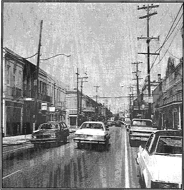
Telephone and utility lines along Magazine Street near Jackson Avenue.
