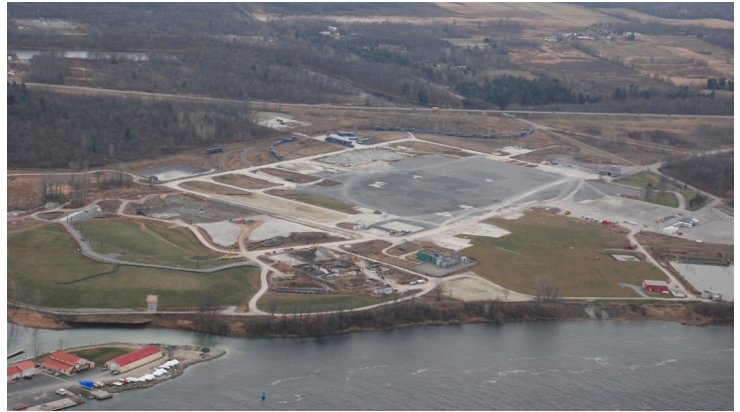
View of building slabs at the GM Massena Superfund site
