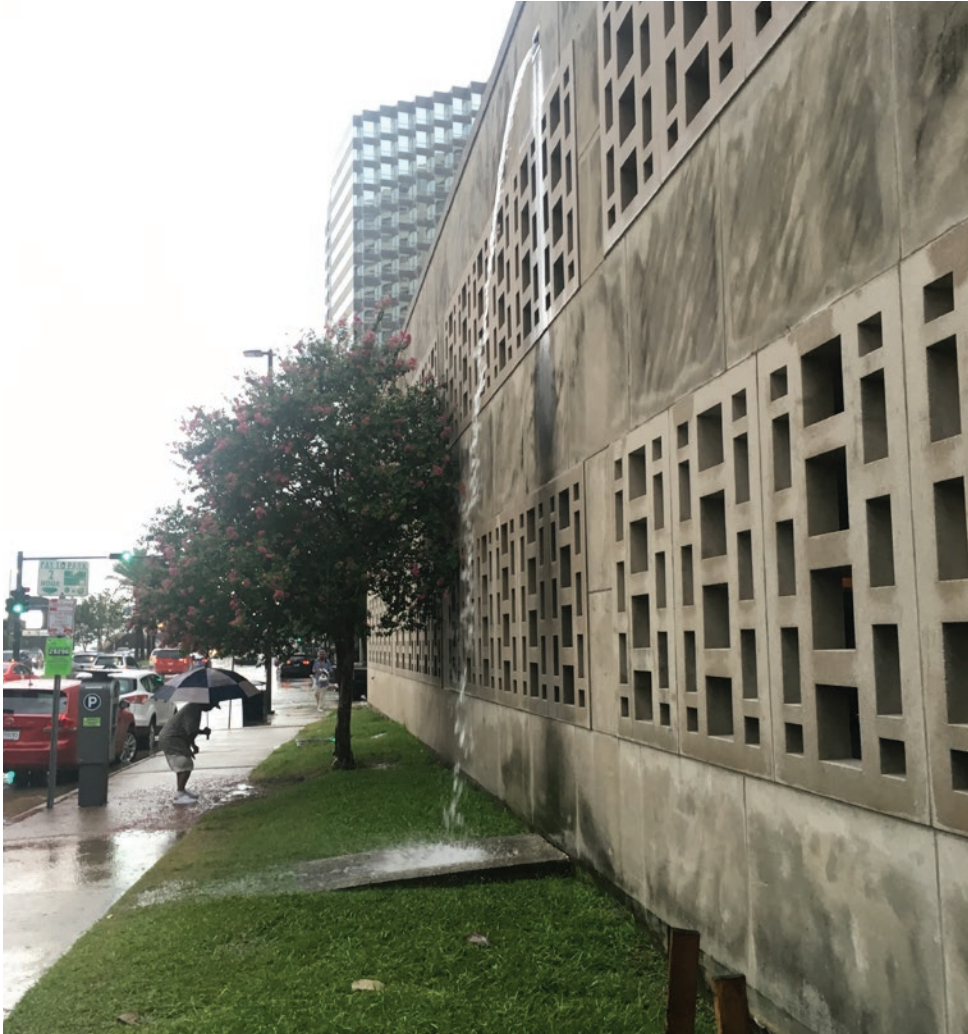
POYDRAS STREET: Water pouring from scupper
