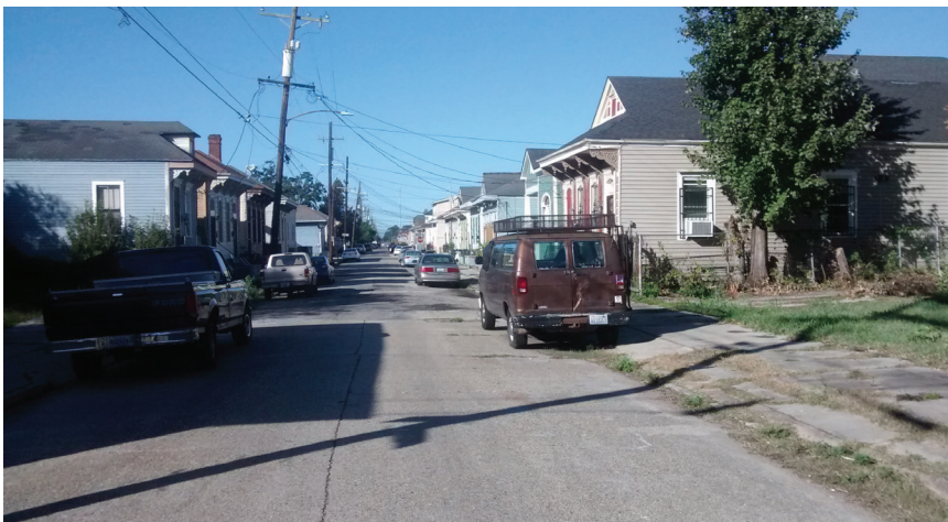
Many of the narrow historic streets in St. Roch are pavement from stoop to stoop.
