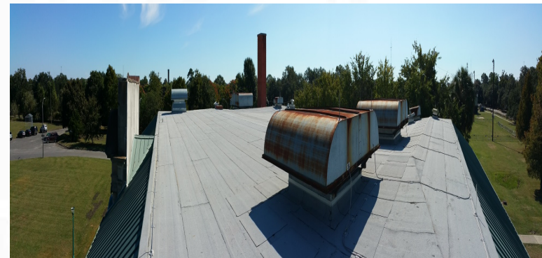
Behrman Gym Roof
