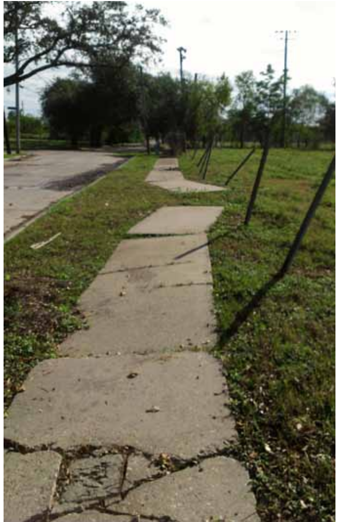
Sidewalks that surround the park site are cracked and inconsistent
