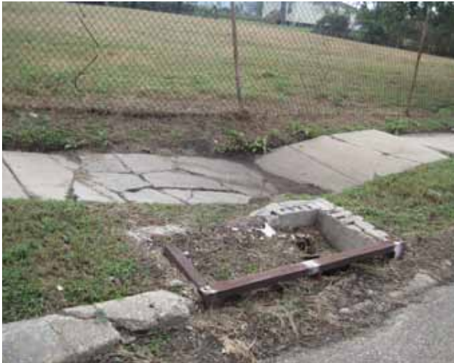
The drains along streets are broken and not functional
