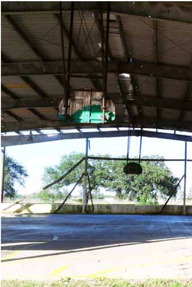
Cracked basketball court and unsafe overhead structure
