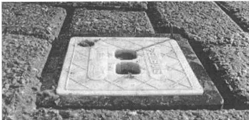
Figure 5 Example of urban groundwater observation well
