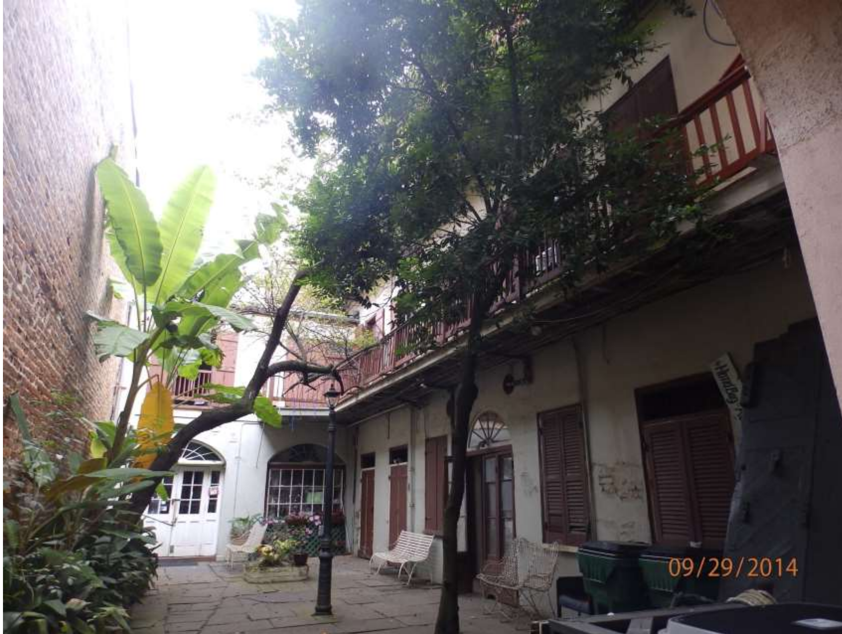
622-624 Royal, existing courtyard
