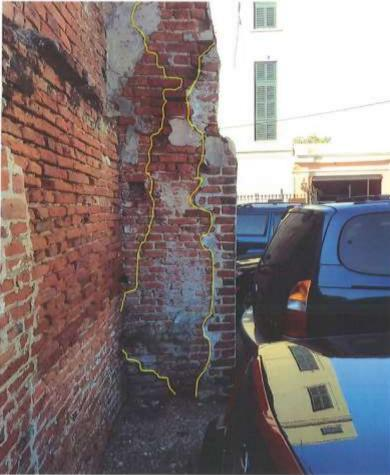
Photo #6-View of cracked section of southwest wall
