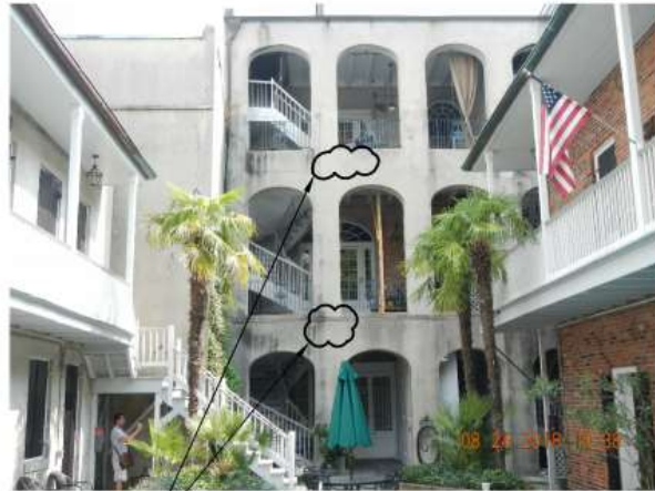
SCOPE OF WORK AREA ON INTERIOR
