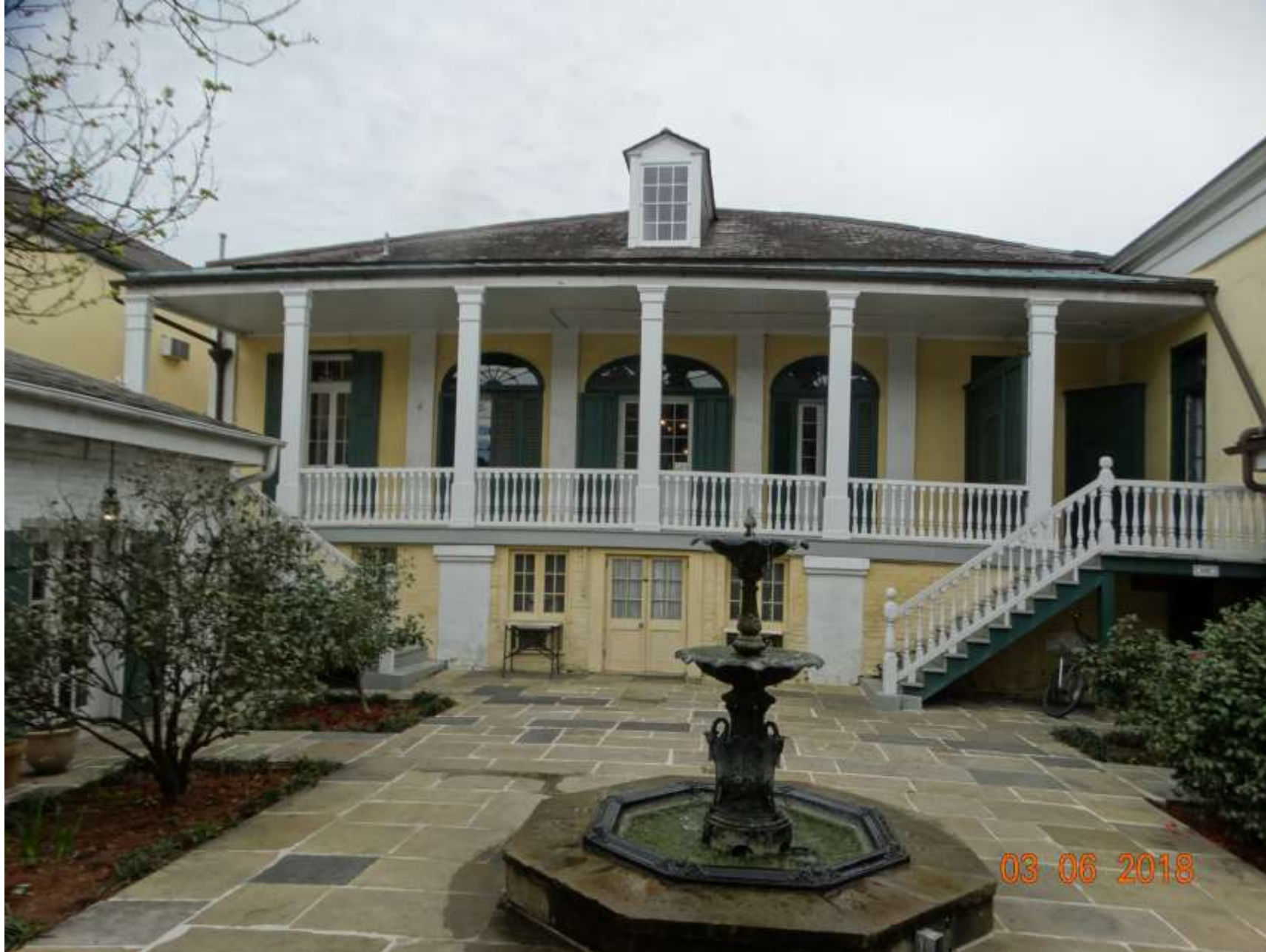
1113 Chartres – Courtyard & Rear Building
