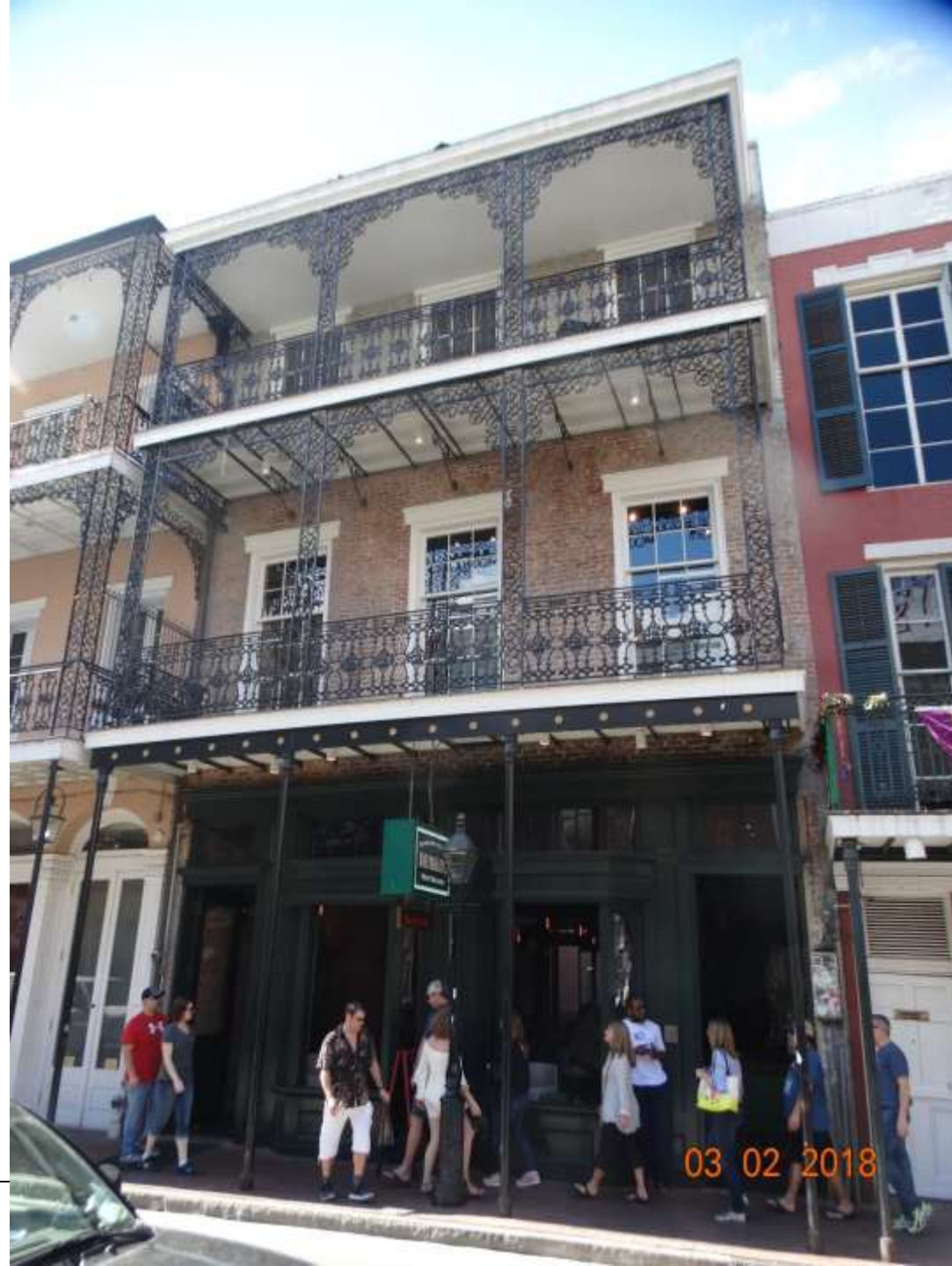
217 Bourbon – After Renovation VCC Architectural Committee
