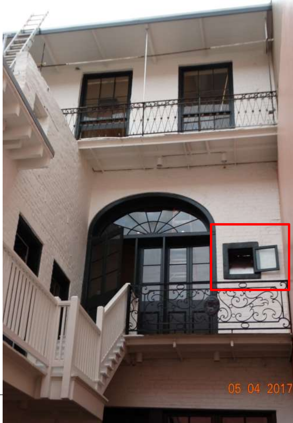
217 Bourbon – Atypical Window VCC Architectural Committee
