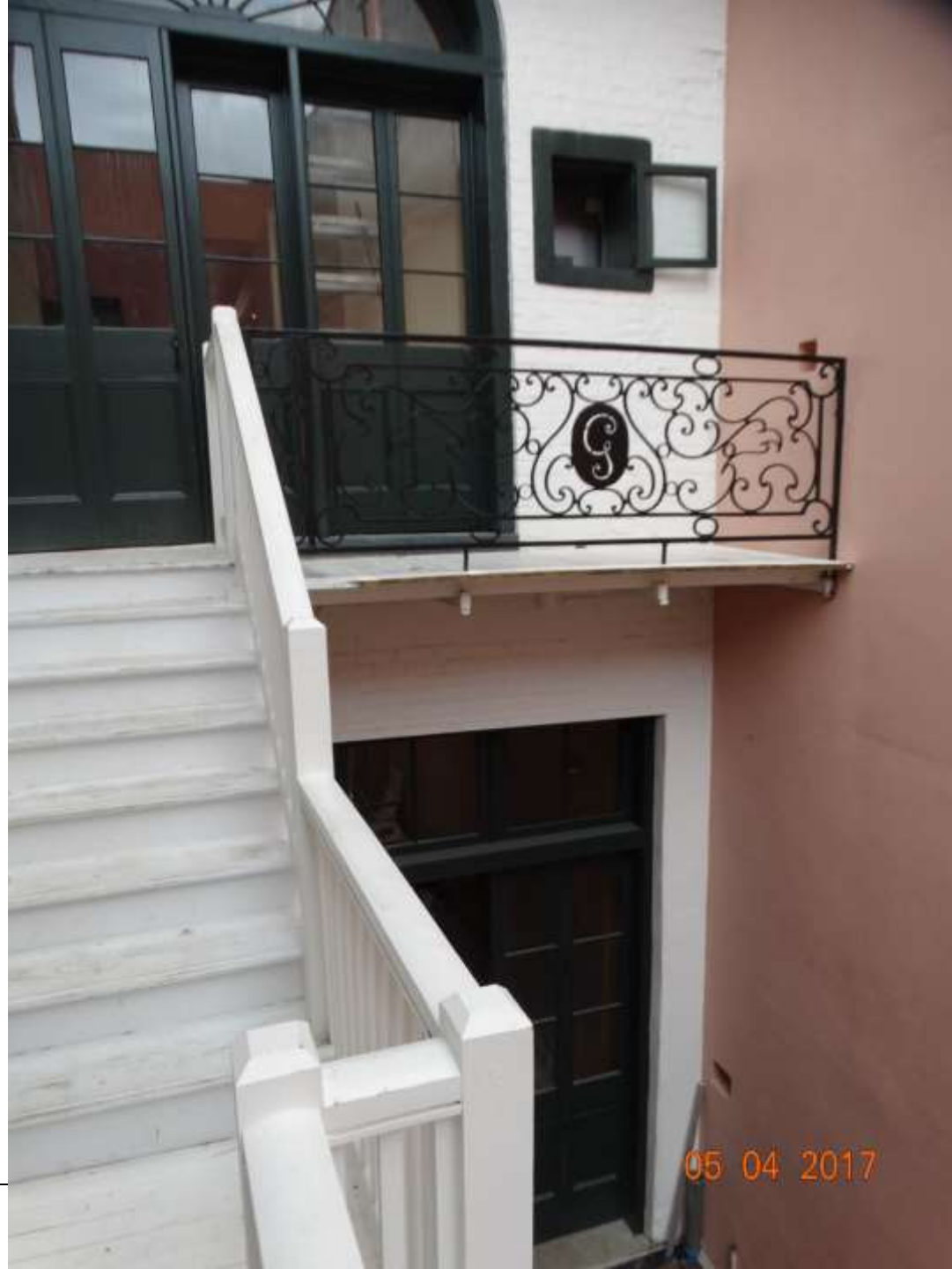
217 Bourbon – Atypical Window VCC Architectural Committee
