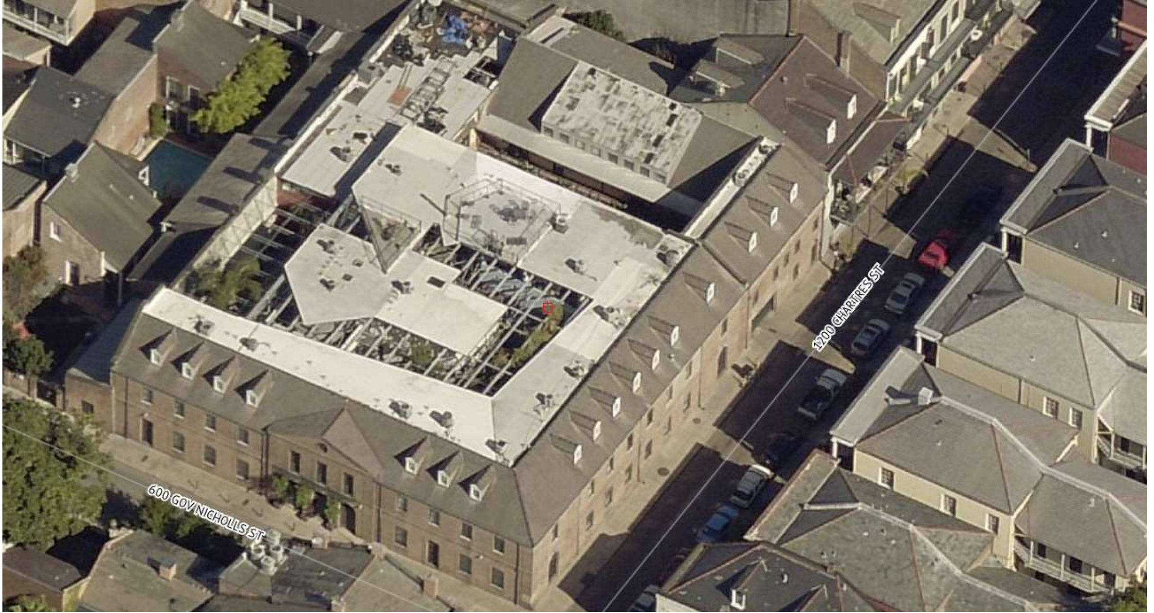
1201 Chartres – Previously existing roof deck
