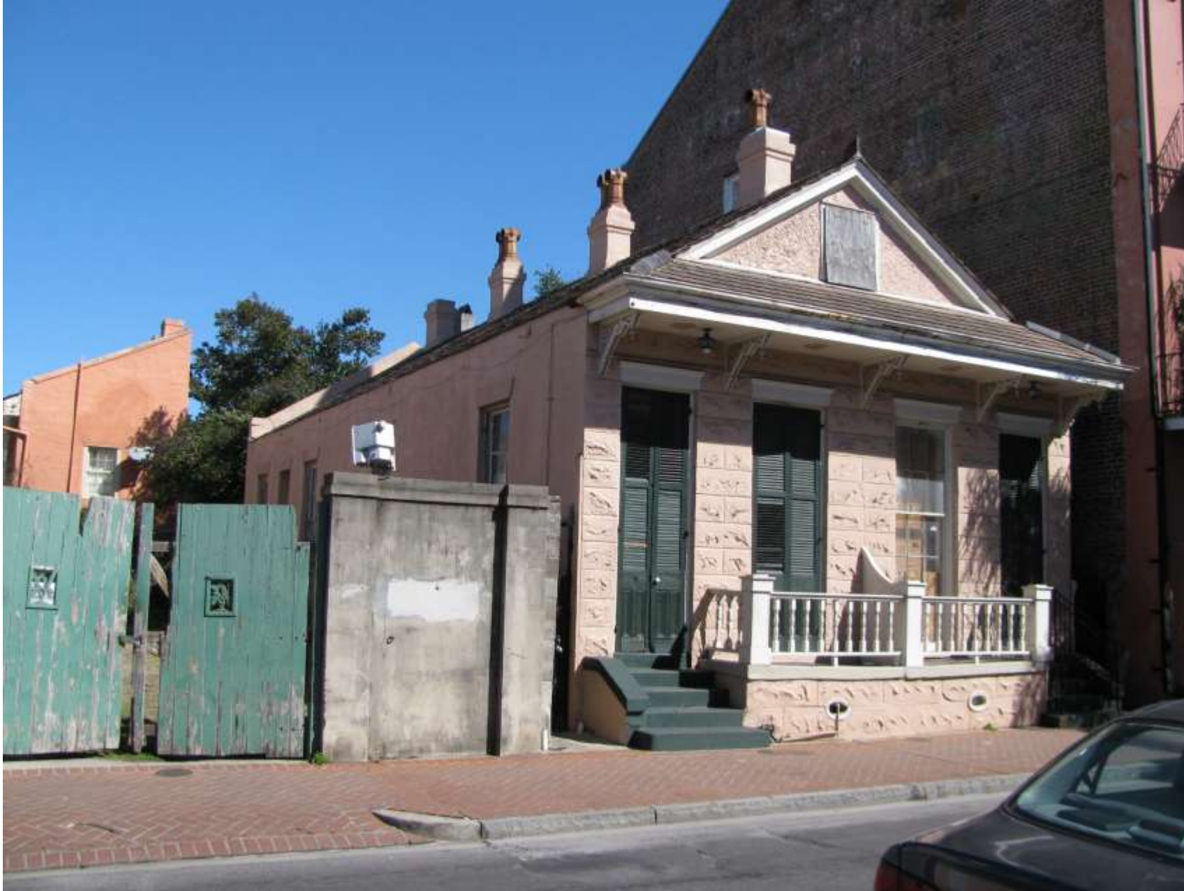
933 Toulouse– 2009 – rails on riverside steps
