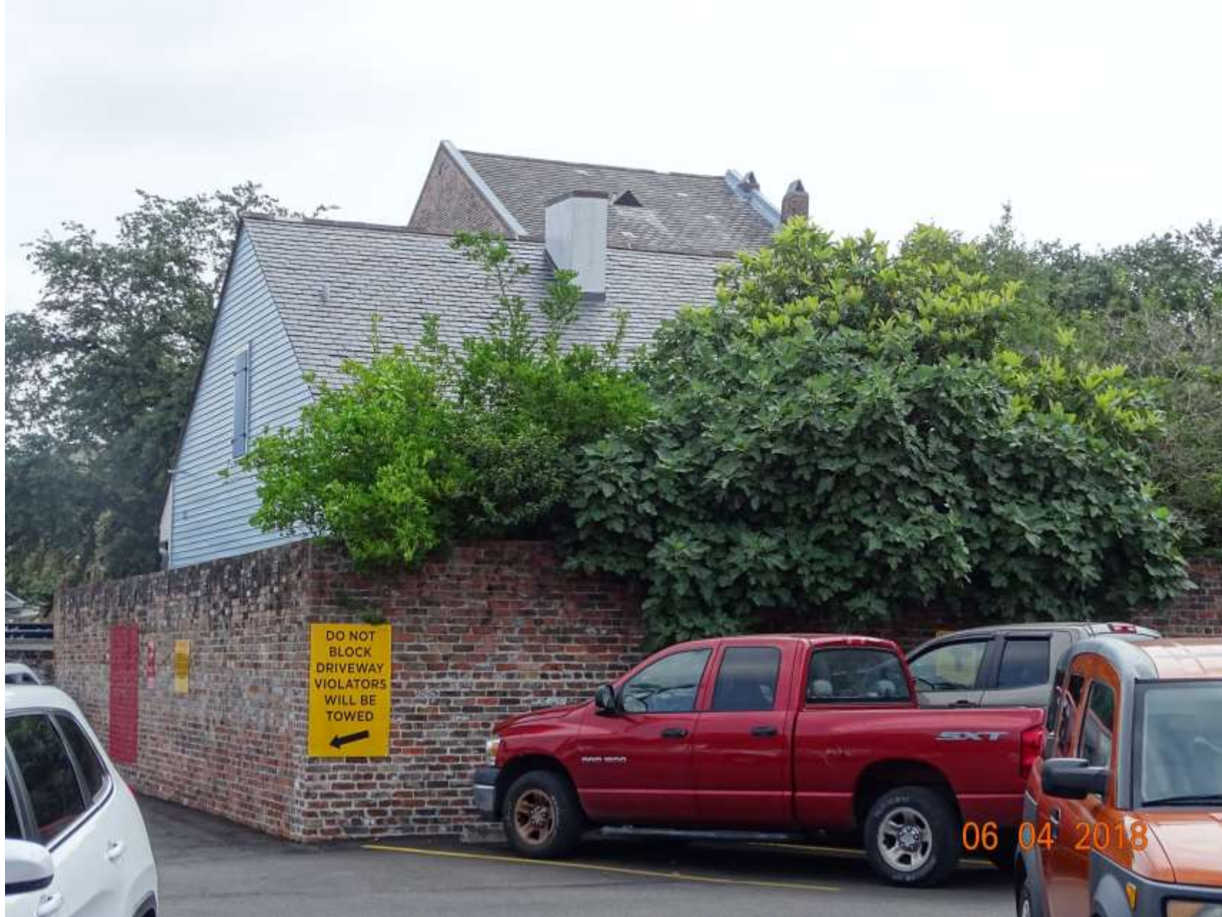
1026 St. Louis – Rear from Parking Lot
