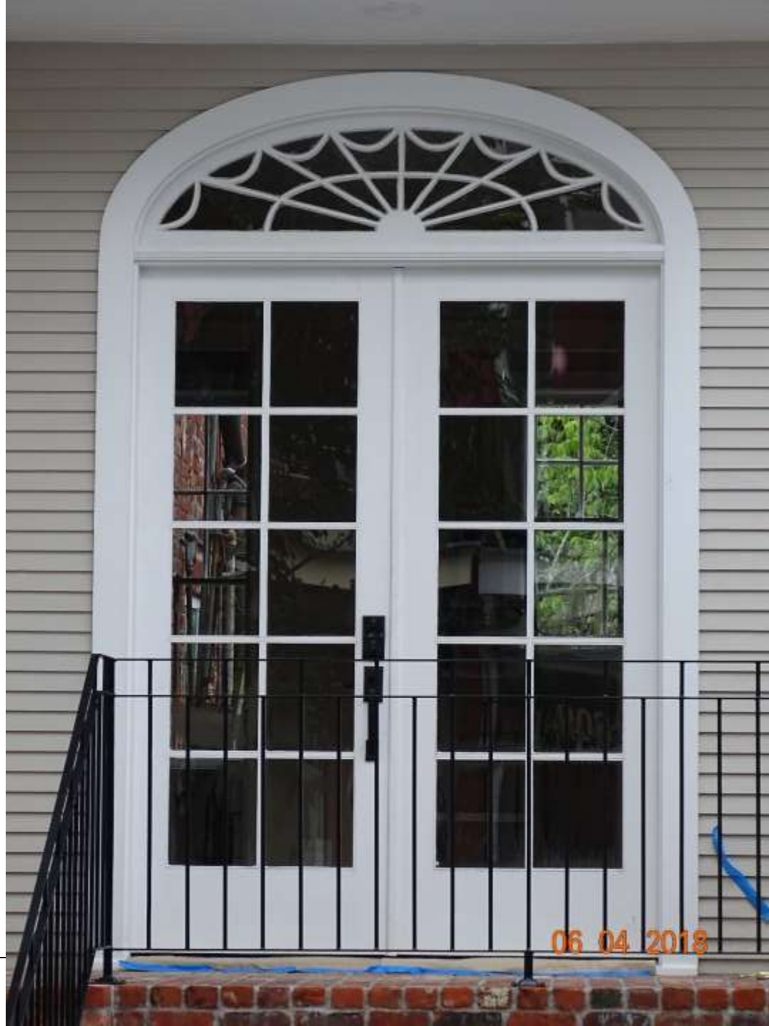
816 Burgundy – As Built Conditions VCC Architectural Committee
