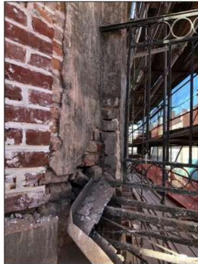
Existing Balcony Connection Condition
