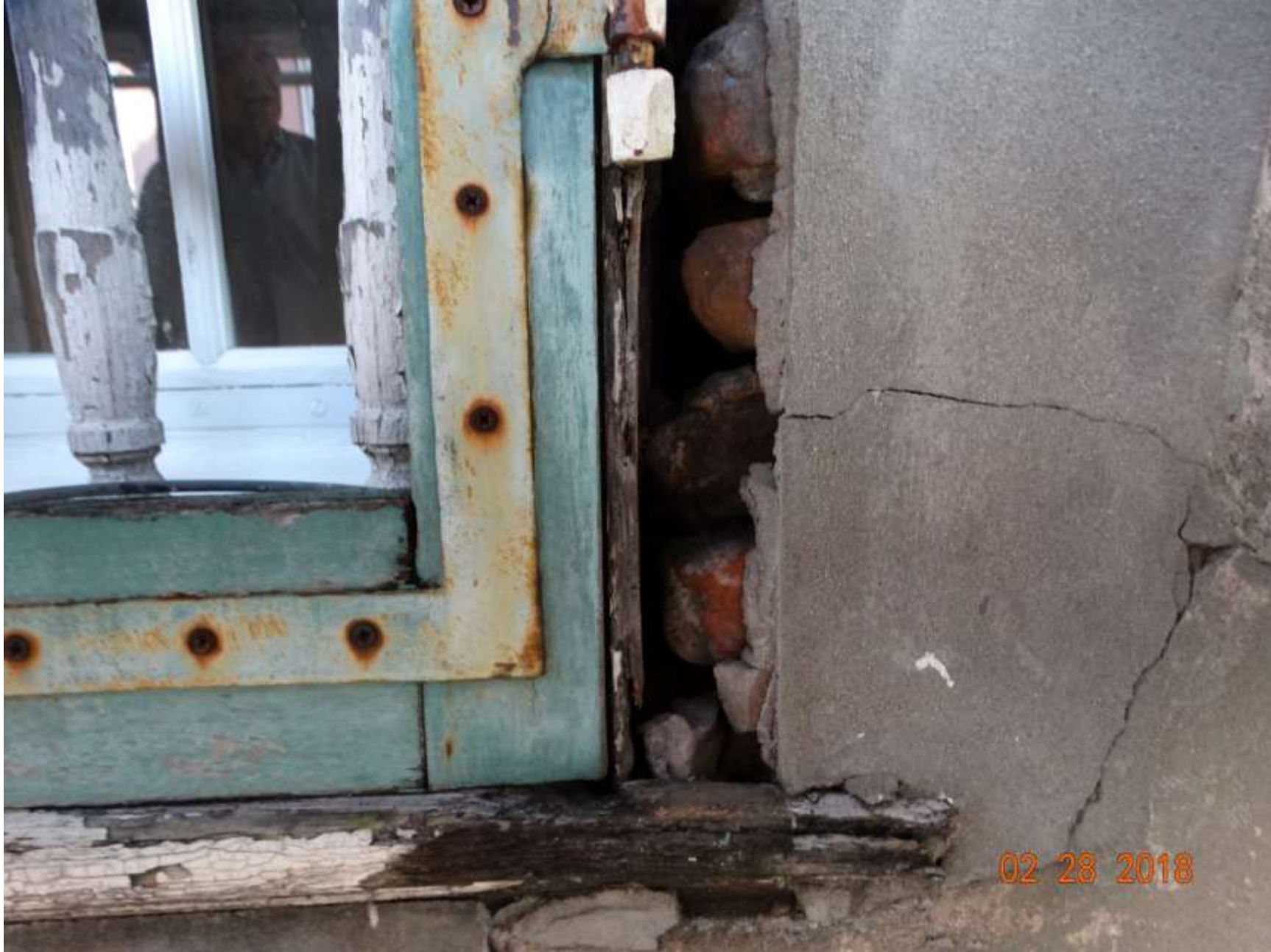
636-40 Royal – Previously Existing Condition
