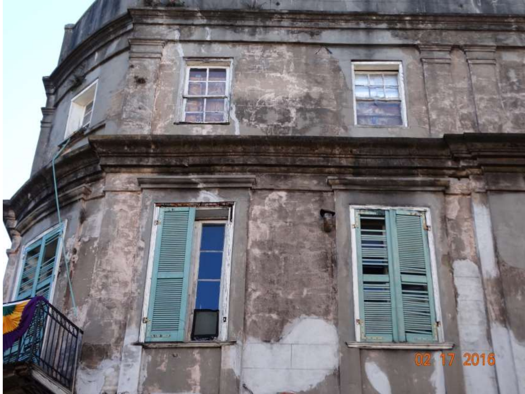
636-40 Royal – Previously Existing Condition
