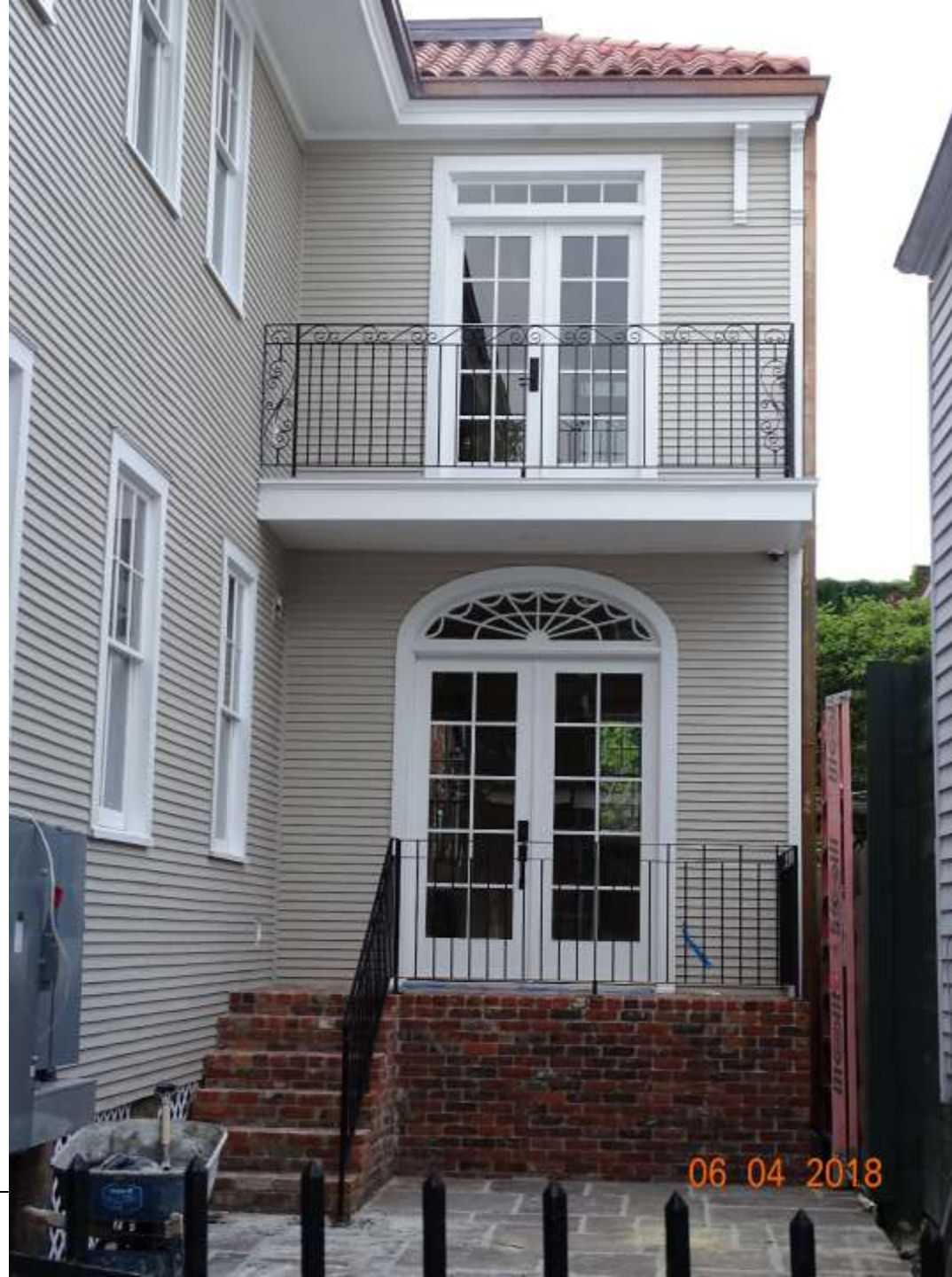
816 Burgundy – As Built Conditions VCC Architectural Committee
