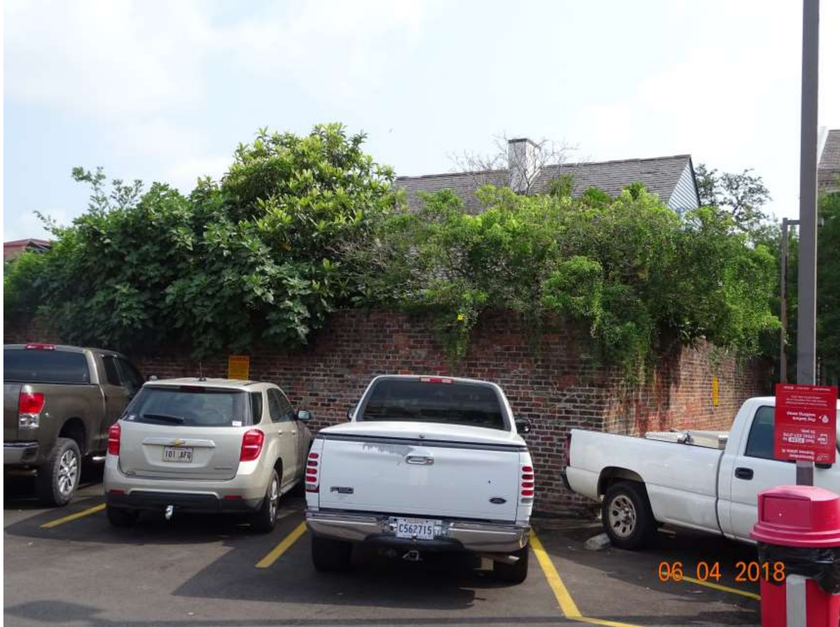
1026 St. Louis – Rear from Parking Lot
