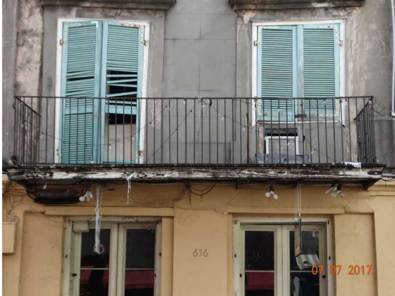
636-40 Royal – Previously Existing Condition
