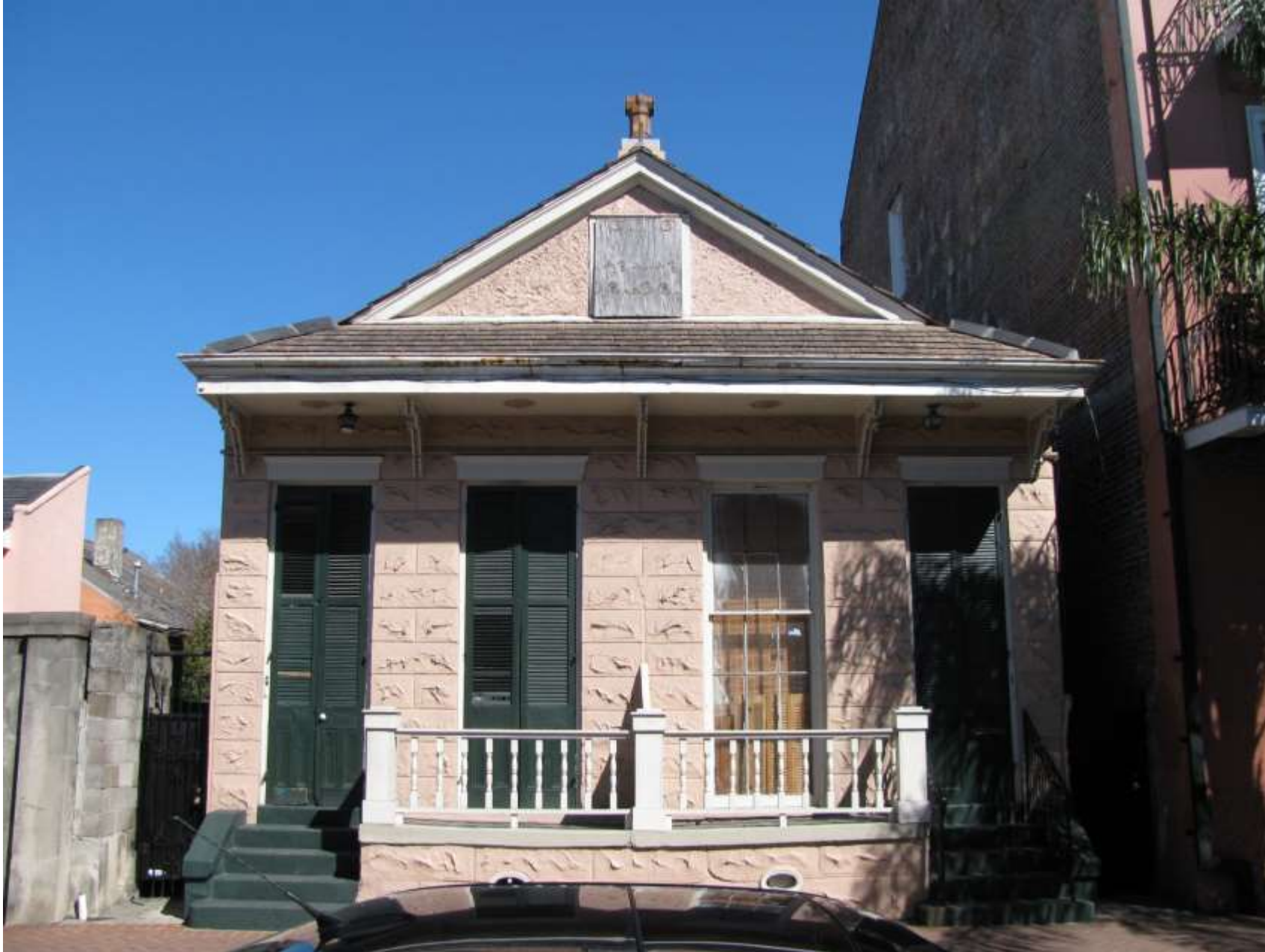
933 Toulouse – 2009 – rails on riverside steps
