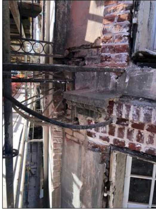
Existing Balcony Connection Condition
