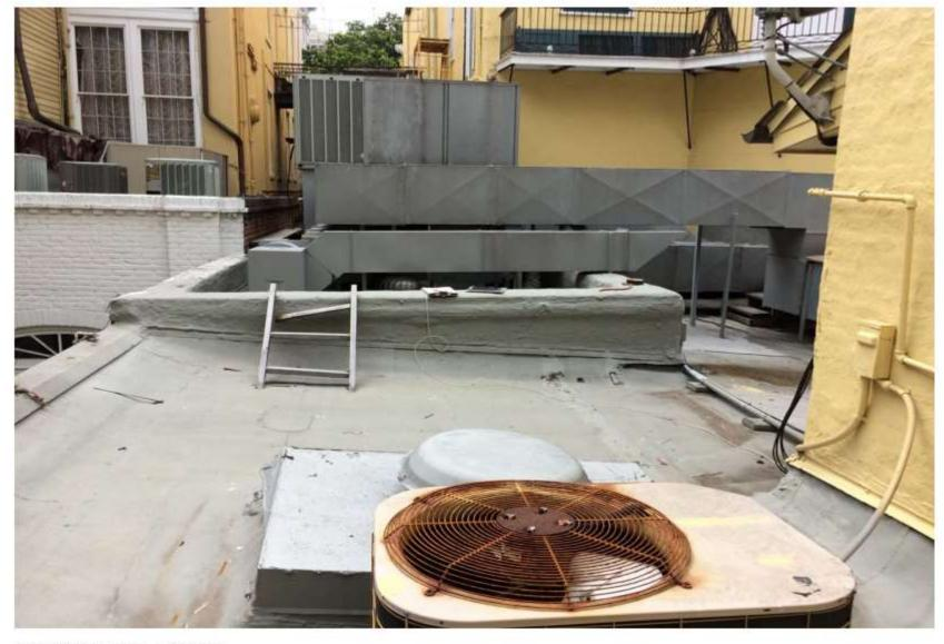
PROPOSED LOCATION FOR RELOCATED #1 AND #2 EQUIPMENT (BETWEEN EXISTING FAN AND PARAPET BEYOND)
