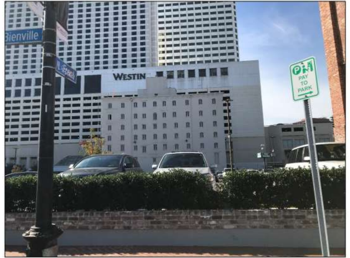
4. View from Bienville Street, looking towards the Bienville St. facade
