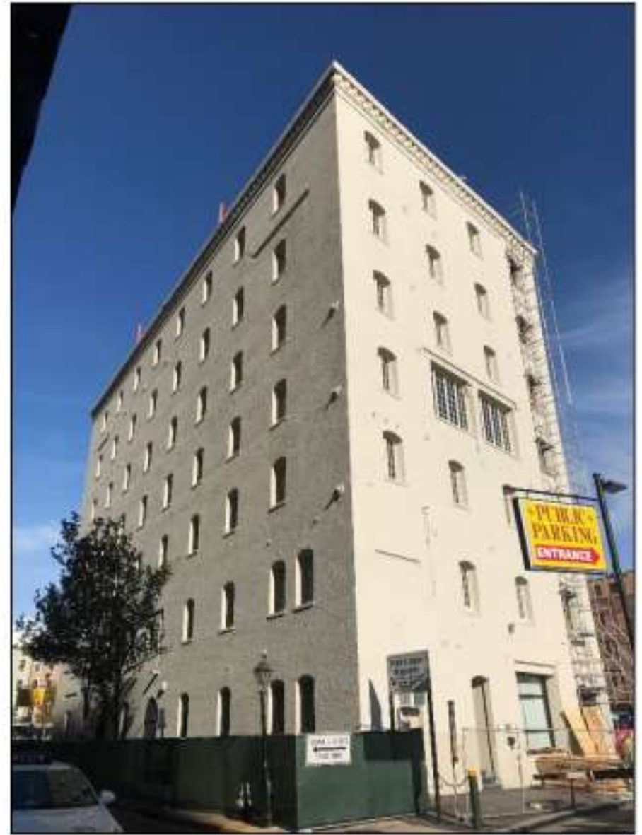
2. View from Iberville Street, towards Riverfront facade
