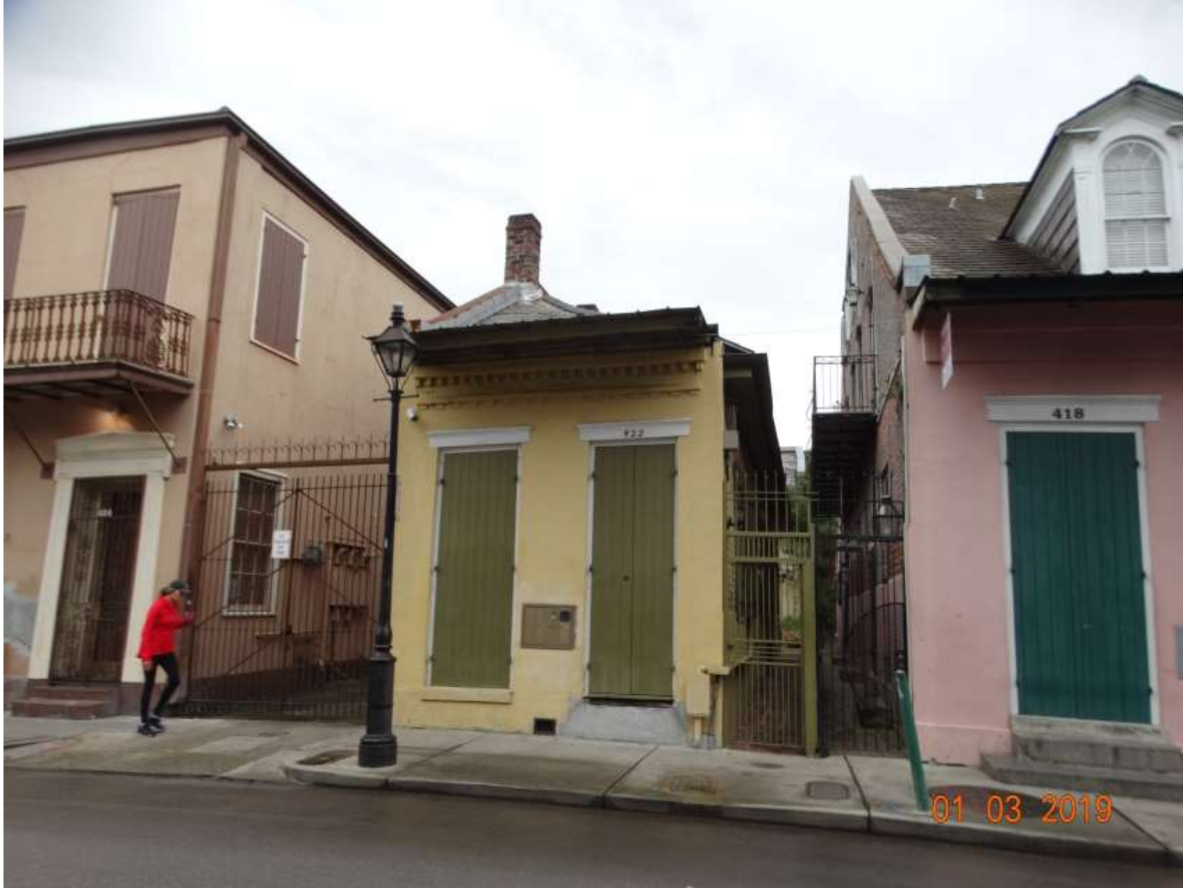
422 Burgundy – Existing Conditions
