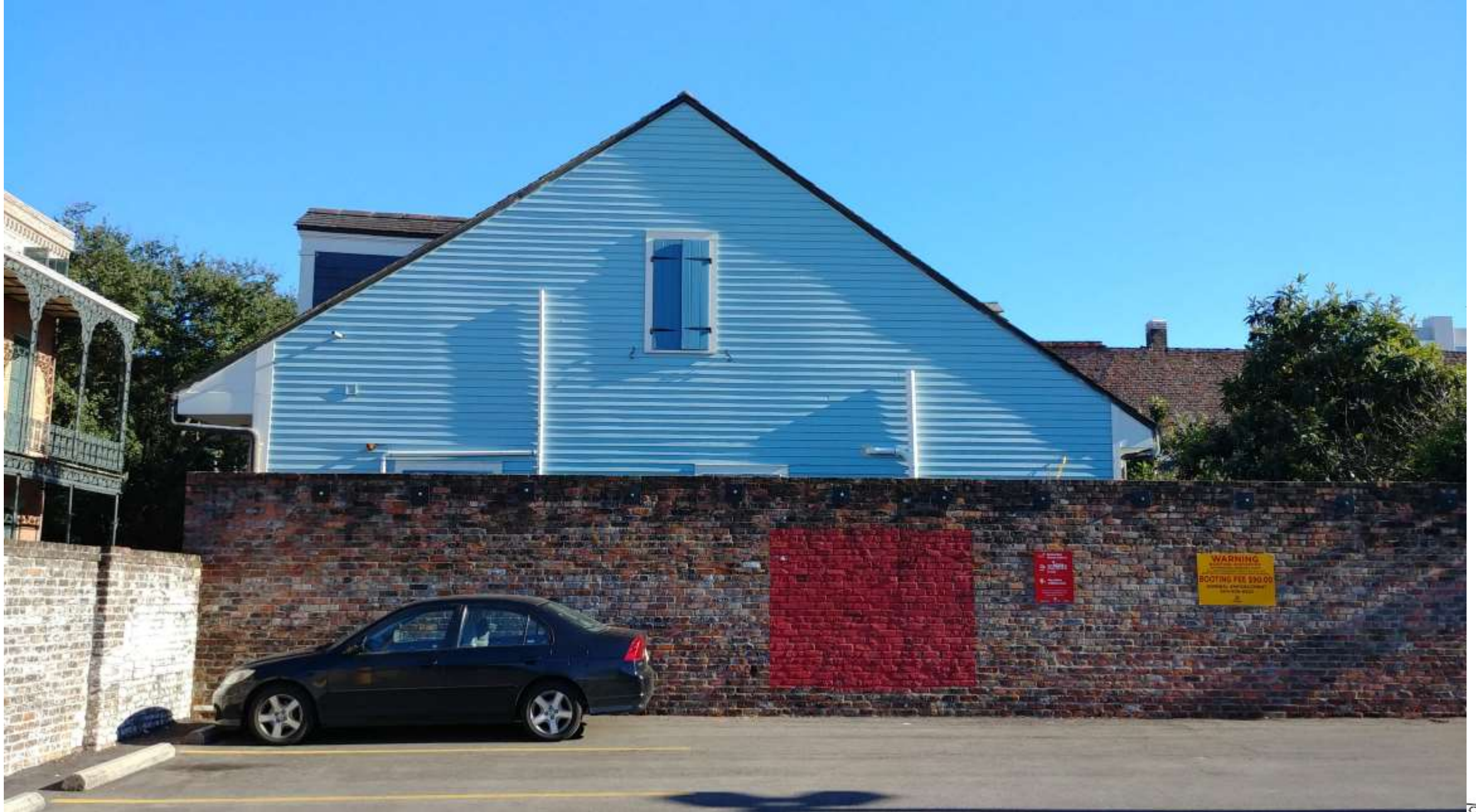
1026 St. Louis – From N. Rampart – As-built Condition
