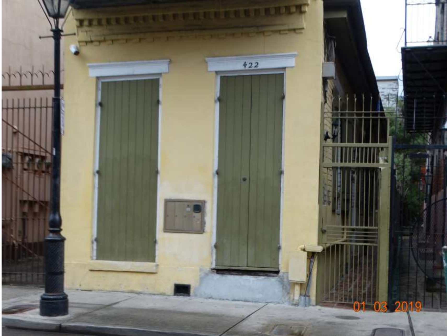
422 Burgundy – Existing Conditions
