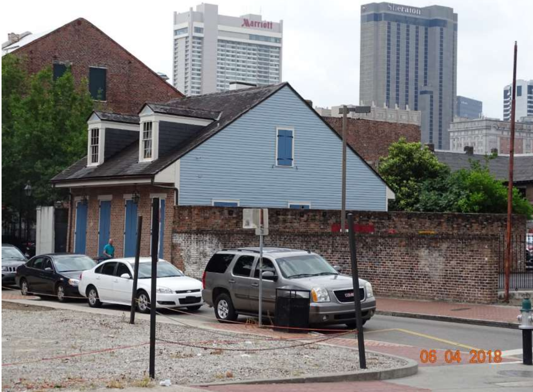
1026 St. Louis – From N. Rampart – Before Pipe Installation
