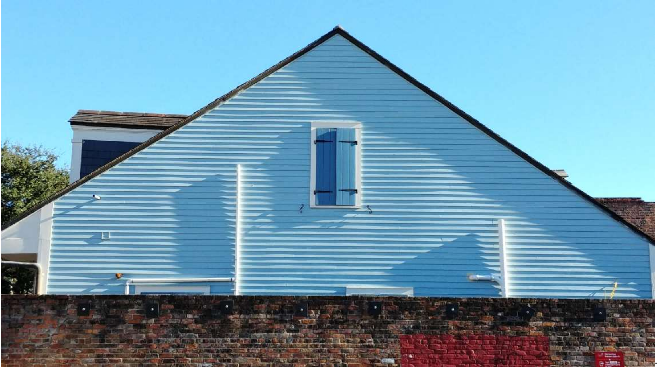
1026 St. Louis – From N. Rampart – As-built Condition
