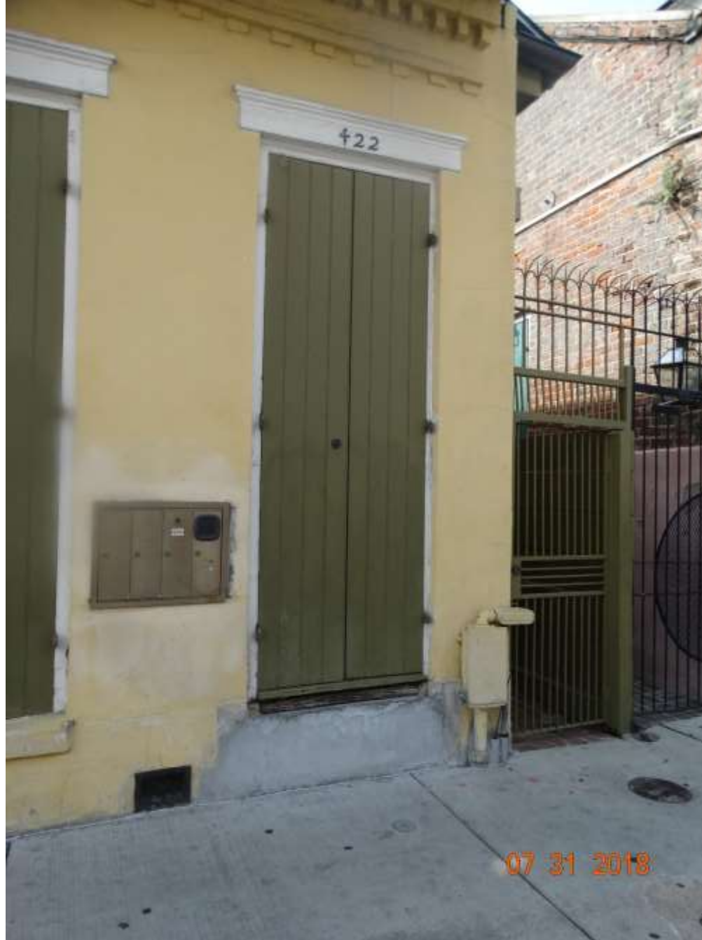
422 Burgundy – Existing Conditions
