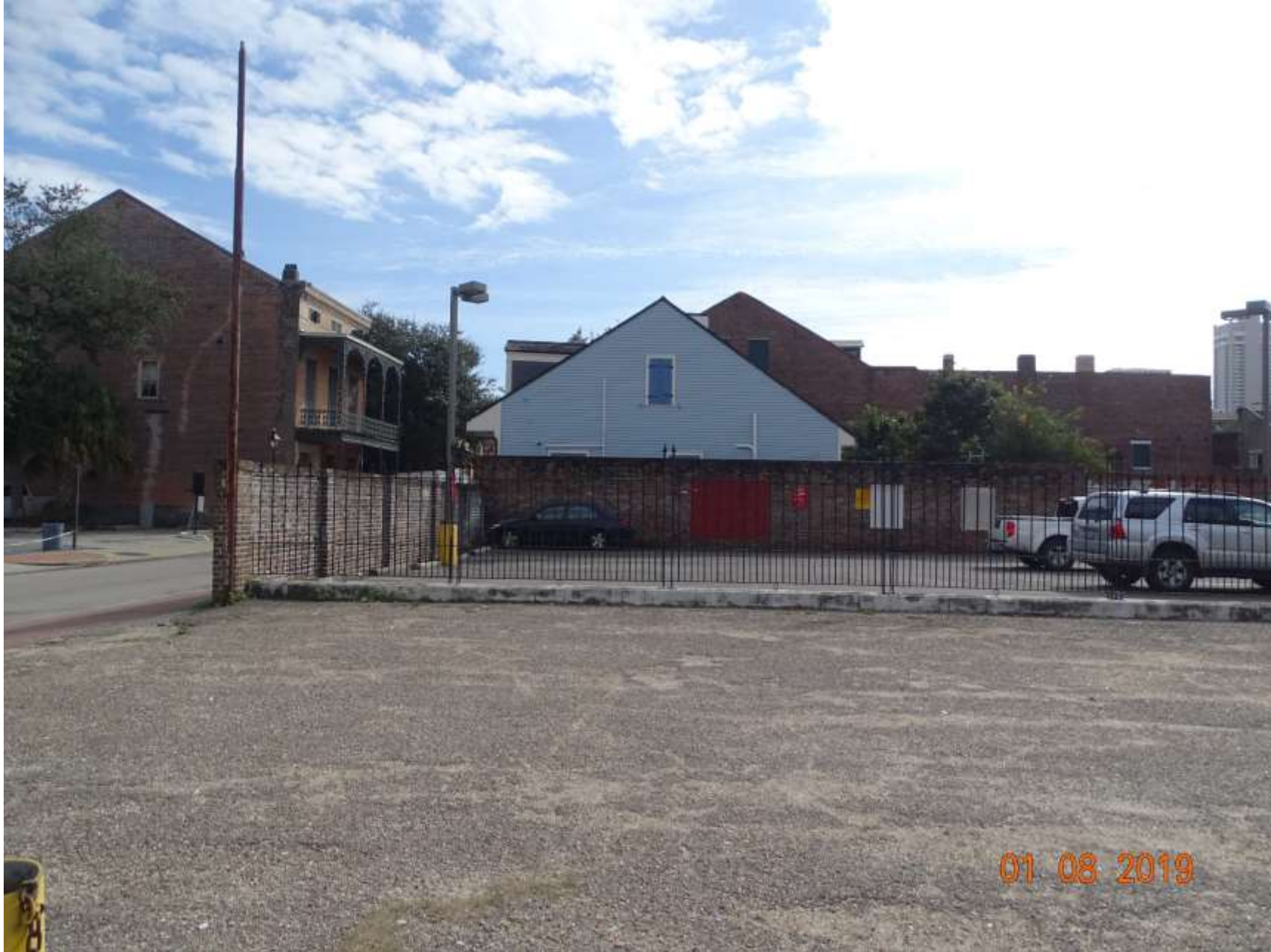
1026 St. Louis – From N. Rampart – As-built Condition
