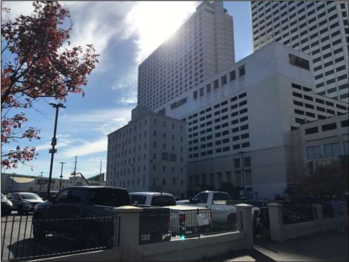
5. View from N. Peters Street, towards the N. Peters and Bienville St facades
