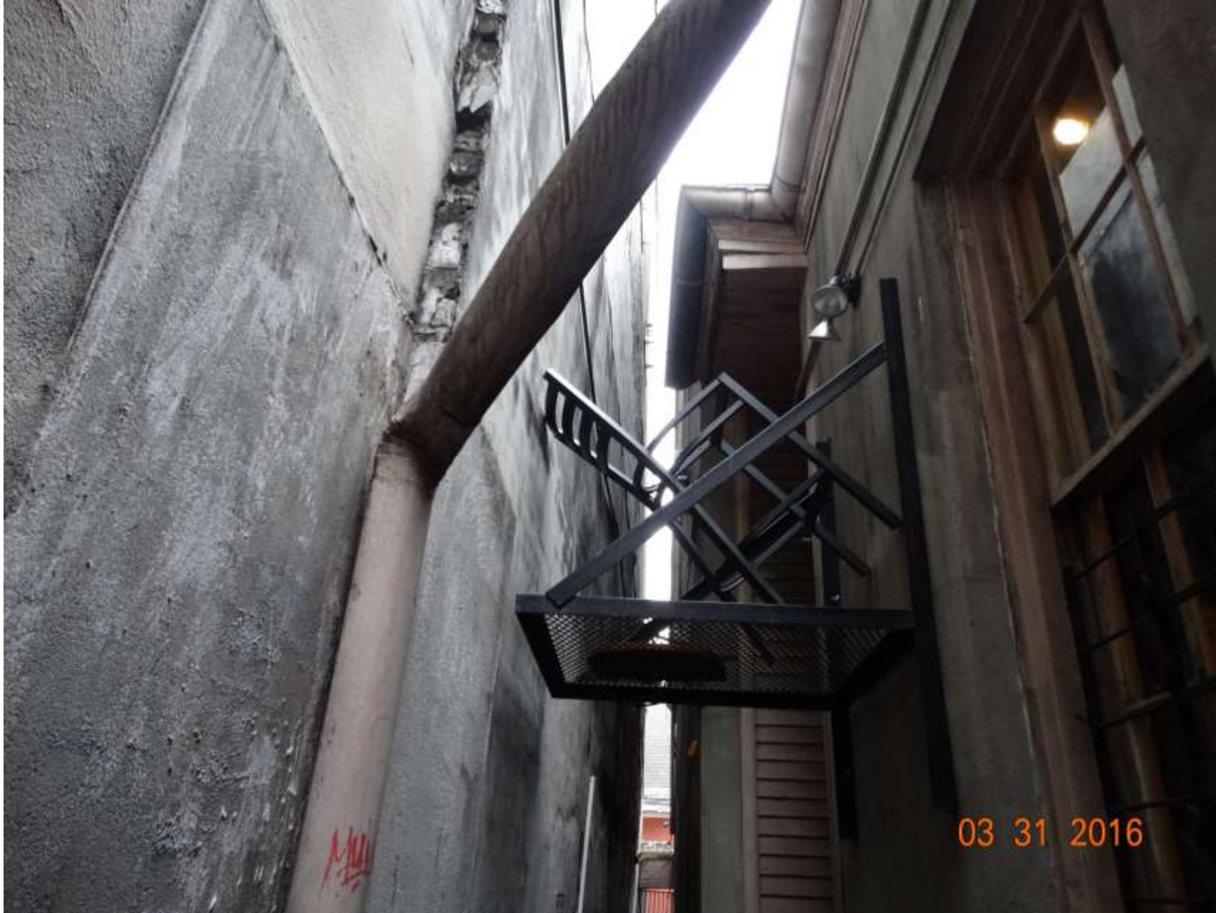
417-19 Bourbon – Third, unused rack
