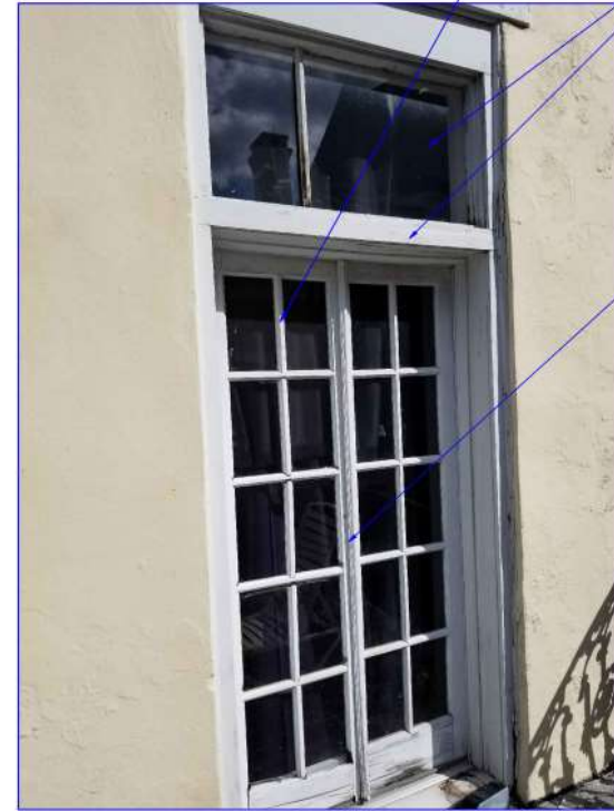
1 DOOR EXTERIOR PHOTO (TYP. EXISTING) NTS
