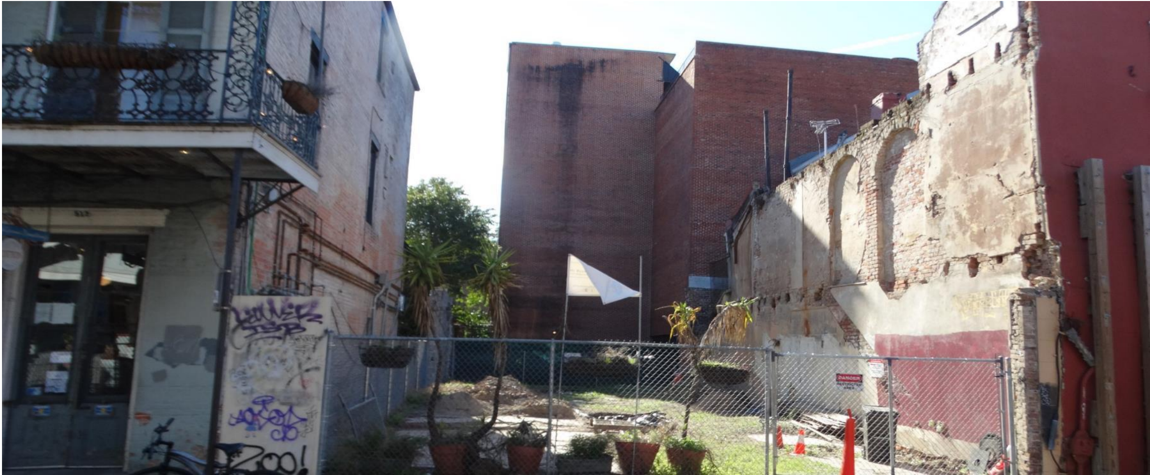
808 Royal – Existing Conditions
