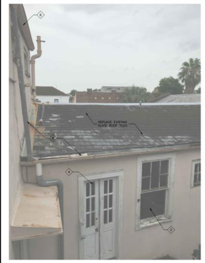
4 PHOTO - ANNEX BUILDING 2ND FLOOR SCALE: 1/8" = 1'-0"
