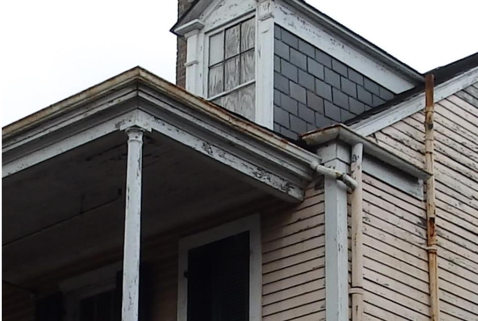
822 Barracks – 2014 – Previously existing gutters and downspout
