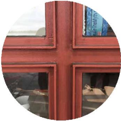
EXISTING PAINTED STEEL
