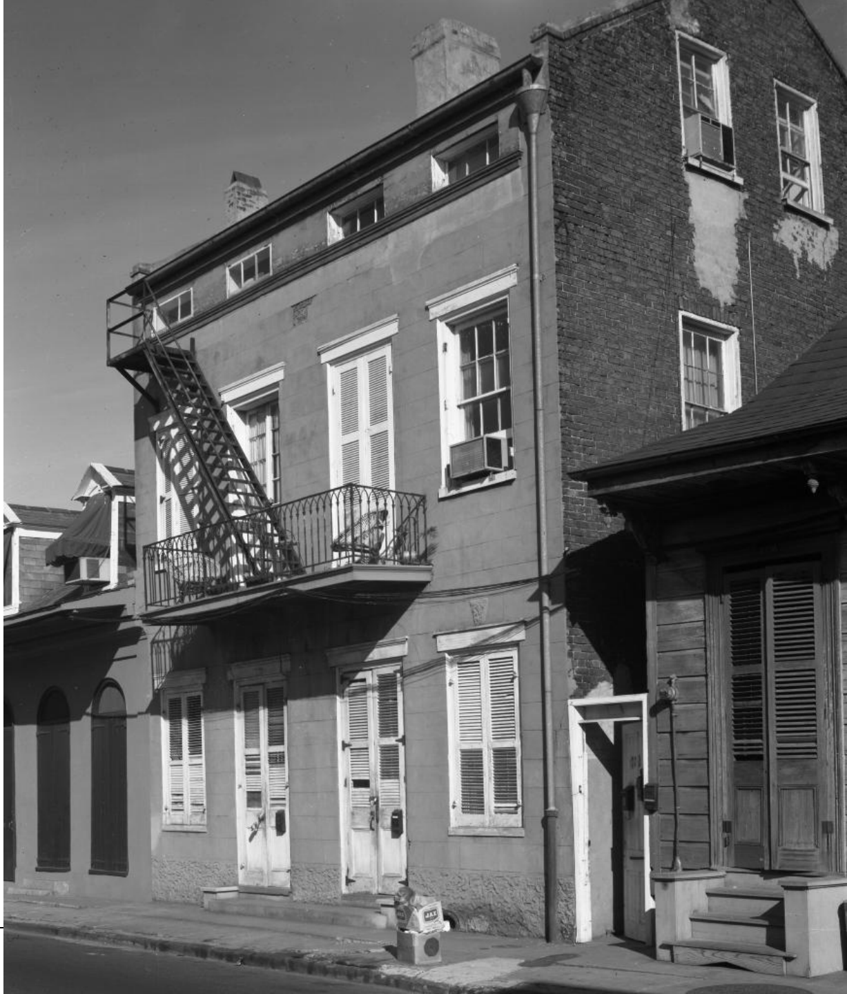
1008 Dauphine VCC Architectural Committee
