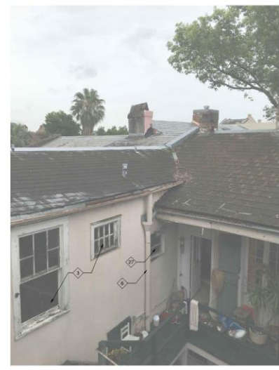
5 PHOTO - ANNEX BUILDING 2ND FLOOR SCALE: 1/8" = 1'-0"
