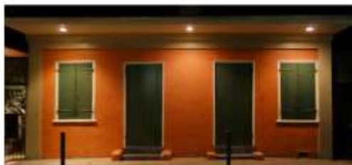
BOURBON ELEVATION (4) SOFFIT RECESSED CANS CENTERED ON (4) DOOR OPENINGS
