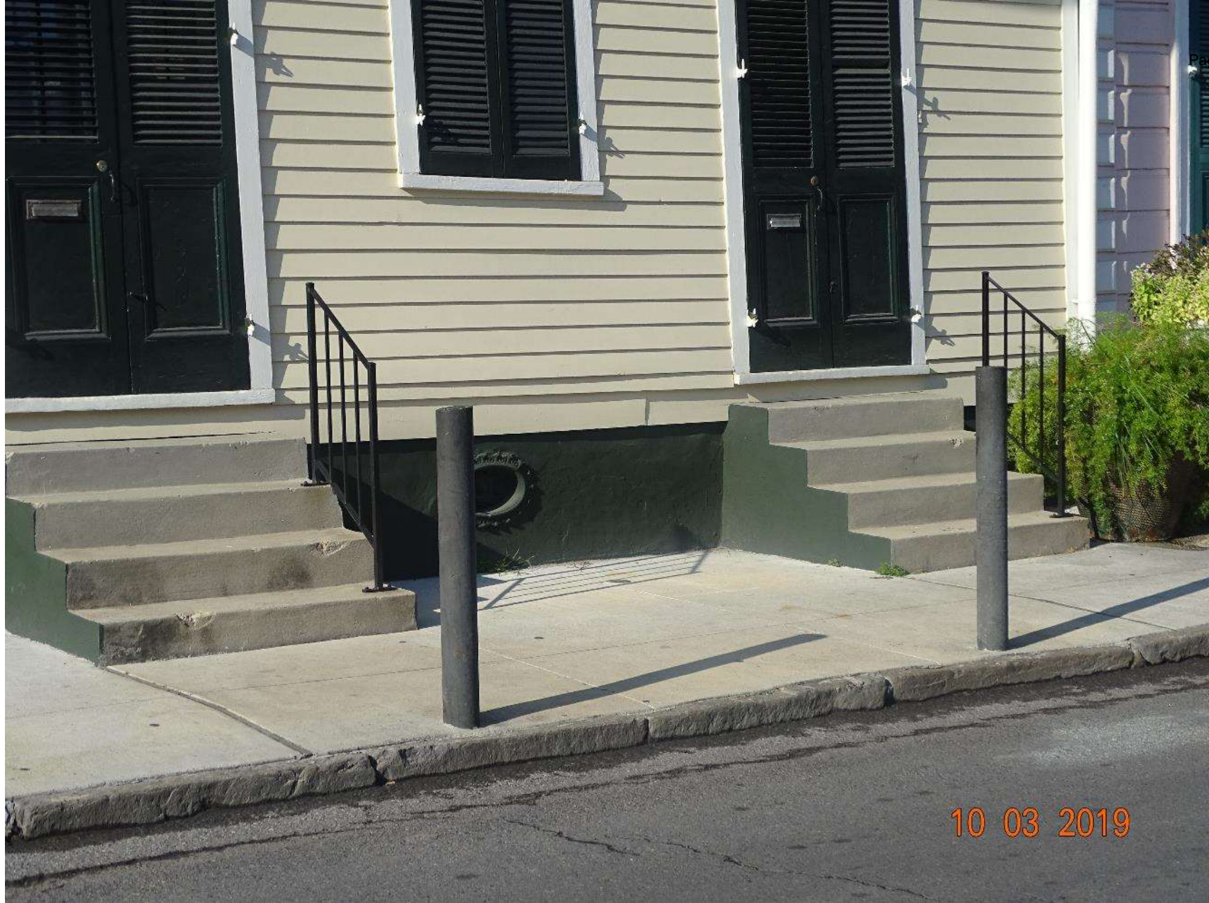
1000 Orleans – Existing Railings on Orleans Elevation
