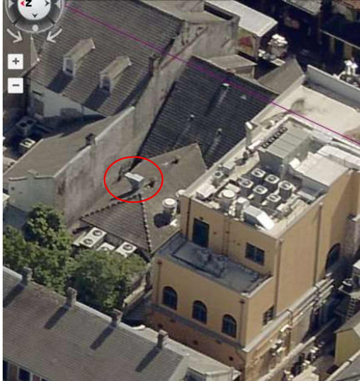
417-19 Bourbon – Previously Existing Air Intake
