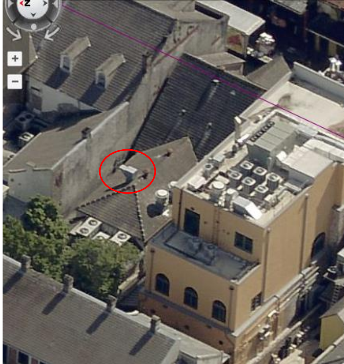
417-19 Bourbon – Previously Existing Air Intake
