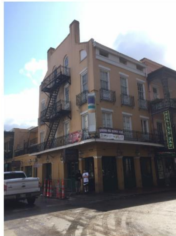
ROOF VISIBILITY ON BOURBON STREET FROM CORNER OF BOURBON AND IBERVILLE STREETS
