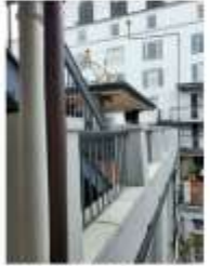
3 STORY WALL AT POOL DECK
