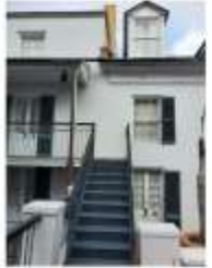
STAIR AT BALCONY ADJOINING POOL DECK
