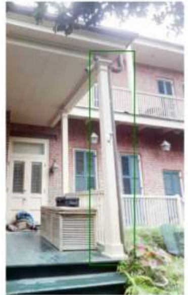
③ PHOTO - EXISTING REAR PORCH COLUMN NTS
