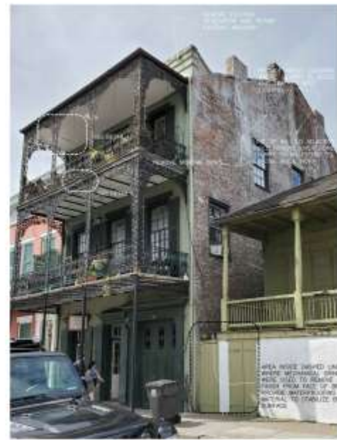
2 NORTH WALL PHOTOGRAPH EXISTING CONDITIONS SCALE: 1/4"
