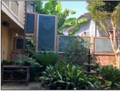
7 SIDE YARD FENCE AT REAR STRUCTURE
