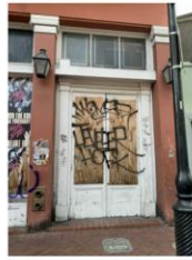
EXISTING STOREFRONT SWING DOORS
