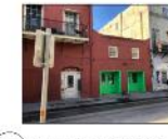
N) DUMAINE STREET [14][8] VEGETATION / WIRING / CONDUIT
