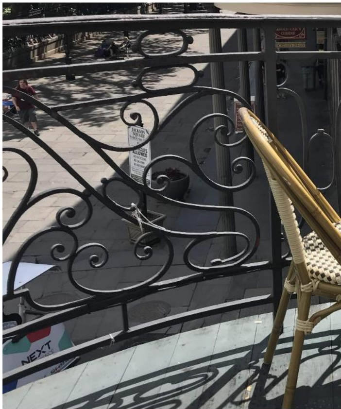
EXISTING CURVED CORNER RAILING
