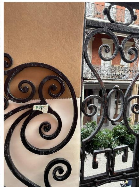
SAMPLE 2- 1/2" SQ. BAR WITH BUTTON SCROLLWORK AND EXISTING 1/2" SQ. RAILING
