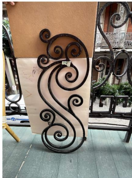
SAMPLE 2- 1/2" SQ. BAR WITH BUTTON SCROLLWORK AND EXISTING 1/2" SQ. RAILING
