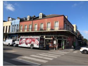
Q) DECATUR STREET [2][4][7][10][11][12] ROOF MATERIAL / PAINT / LIGHTING / WALLS / ROOF TILE / RIDGES / CAPS / TRIM
