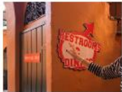
SIZE AND LOCATION OF EXISTING VINYL SIGN TO BE HUNG FROM SPINDLES IN SAME LOCATION OF STAIR ABOVE USING MOVABLE TEMPORARY ATTACHMENTS. NO ALTERATIONS TO EXISTING WALL.
