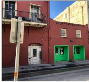
B) DUMAINE STREET [8][14] VEGETATION / WIRING / CONDUIT
