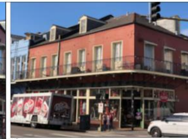
S) DECATUR/DUMAINE STREET [2][4][7][10][11][12] ROOF MATERIAL / PAINT / LIGHTING / WALLS / ROOF TILE / RIDGES / CAPS / TRIM
