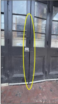
THESE PHOTOS SHOW THE CURRENT CONDITION OF THE FRONT DOOR WITH GAPS, HOLES AND UNSTABLE FROM THE BOTTOM & TOP.
