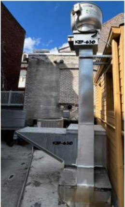
⑤ BLDG 630 - KITCHEN HOOD EXHAUST & SUPPLY FANS
