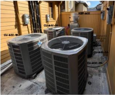
⑦ BLDG 632-4) A/C COND UNITS, HOOD EXHAUST FAN & COOLER COMP
