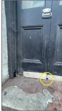
THESE PHOTOS SHOW THE CURRENT CONDITION OF THE FRONT DOOR WITH GAPS, HOLES AND UNSTABLE FROM THE BOTTOM & TOP.
