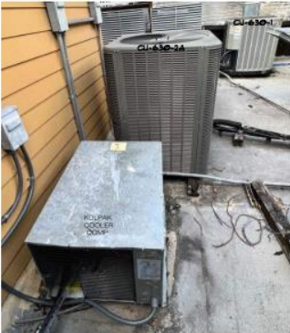
⑥ BLDG 630 - WALK-IN COOLER COMP & A/C COND UNITS
