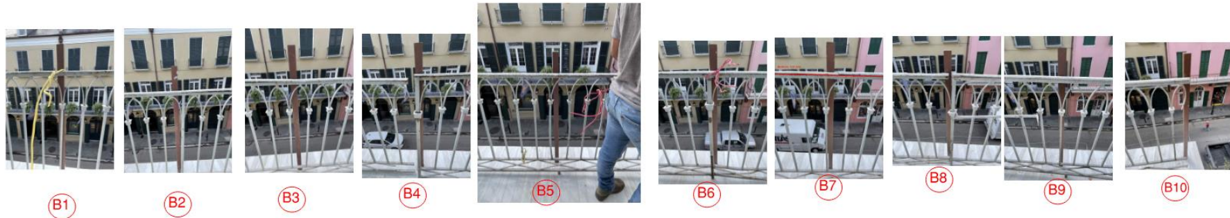
THIRD FLOOR BALCONY ROUGH MOCK UP THE EXISTING RAILINGS TO NEW POSTS
