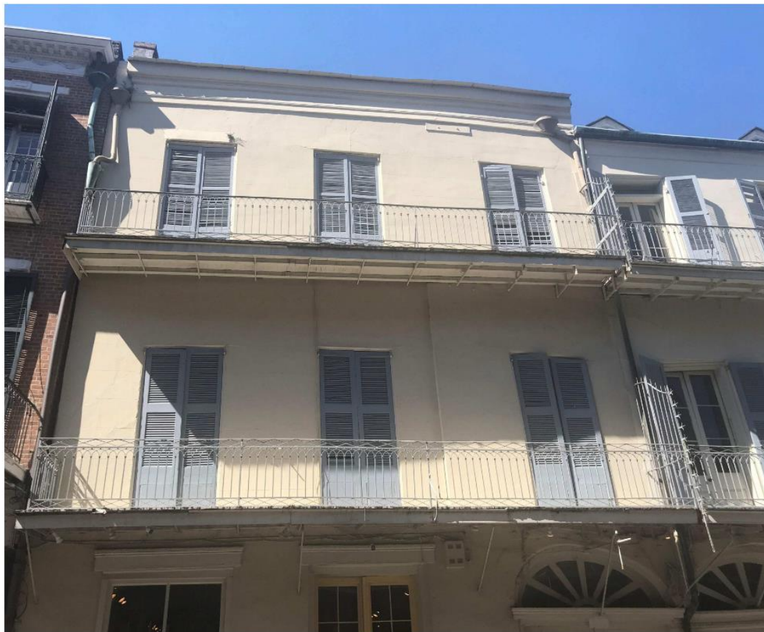
EXISTING BALCONY CONDITION
