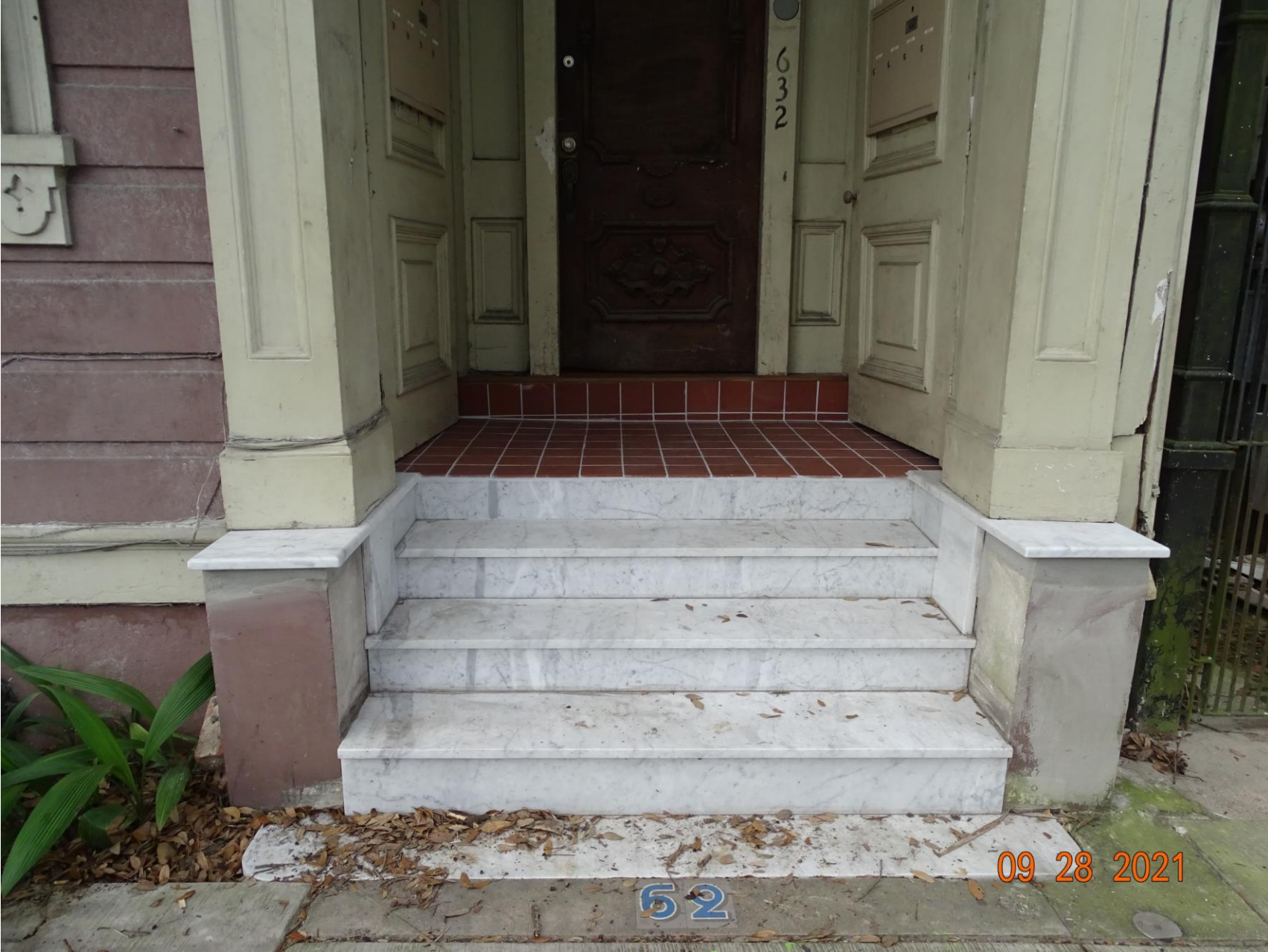
632 Esplanade – Replacement Steps
