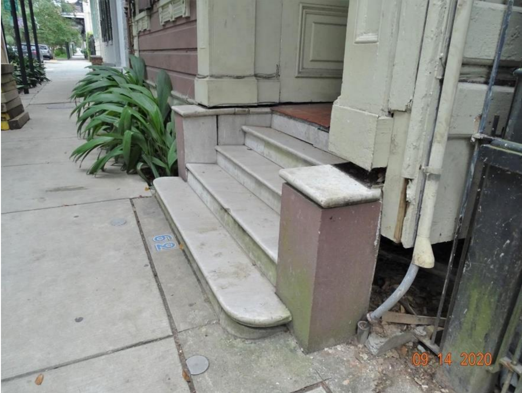
632 Esplanade – Previously existing steps
