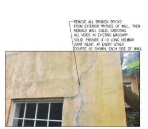
4 DETAIL-REPAIR OF MASONRY WALLS 1/4"=1'-0"
