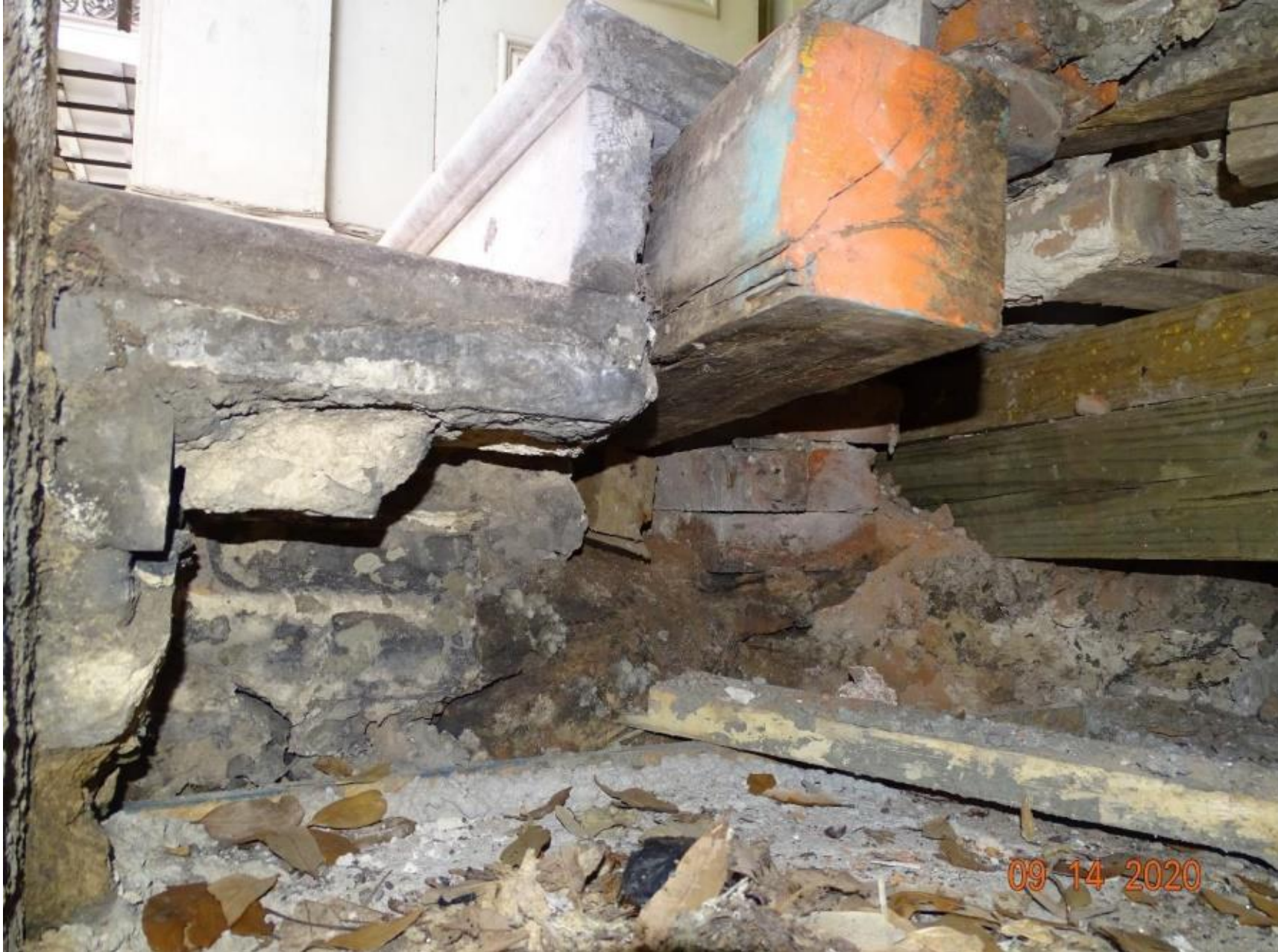
632 Esplanade – Previously existing steps
