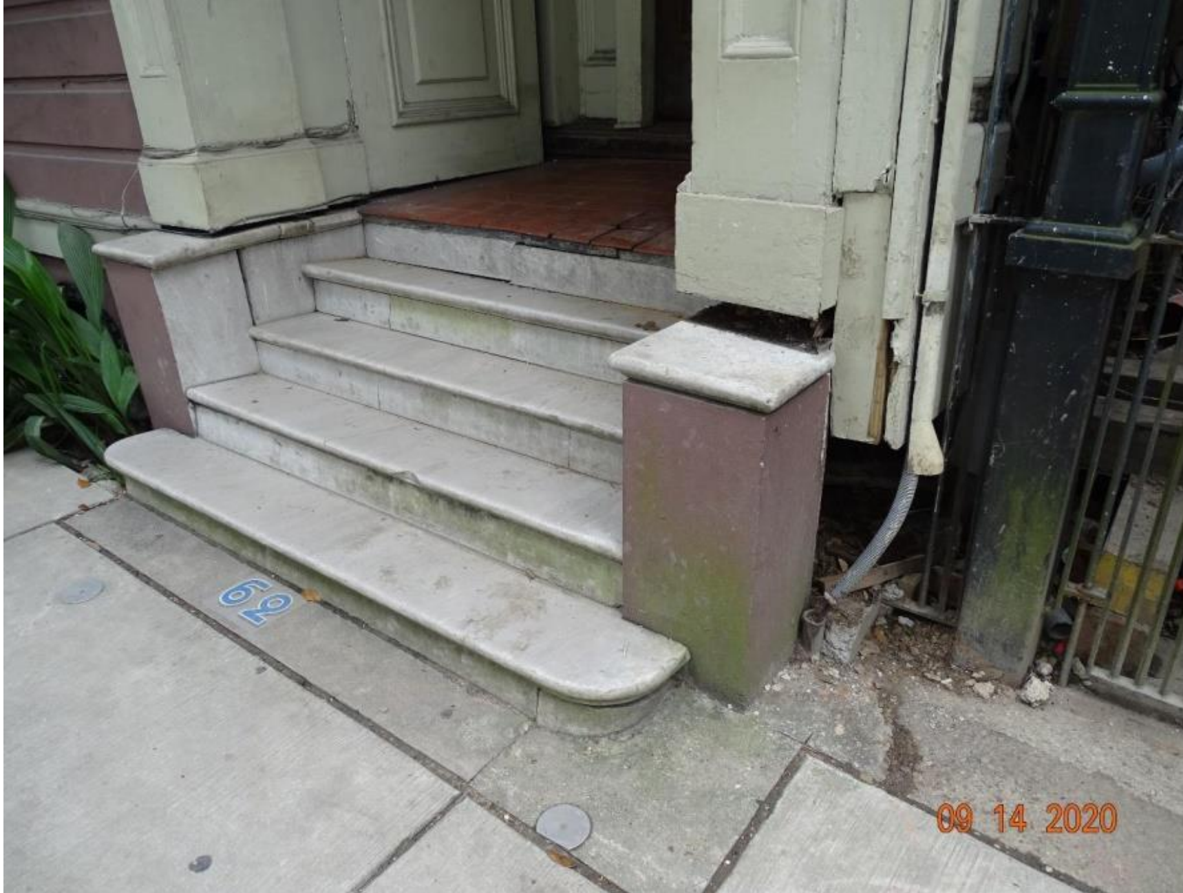
632 Esplanade – Previously existing steps
