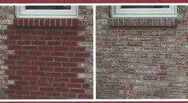
A potassium silicate tint (right) was created to successfully blend the mismatched repair work (left) with the original surrounding brick.
