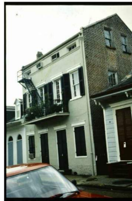
VCC Library Photo of 1008 Dauphine, 1991 This image shows square/stepped trim at the bottom of the frieze band, which we believe is closer to the historic condition.
