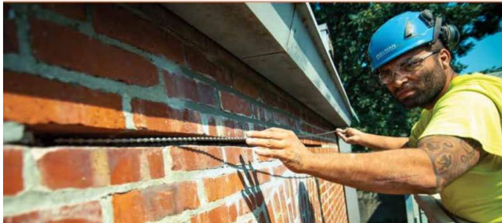
HELICAL BEAMING TO REINFORCE ROUGH OPENINGS
