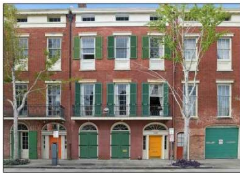
Julia Row, NOLA Greek Revival Frieze Band Windows with stepped/square and dentil trim elements
