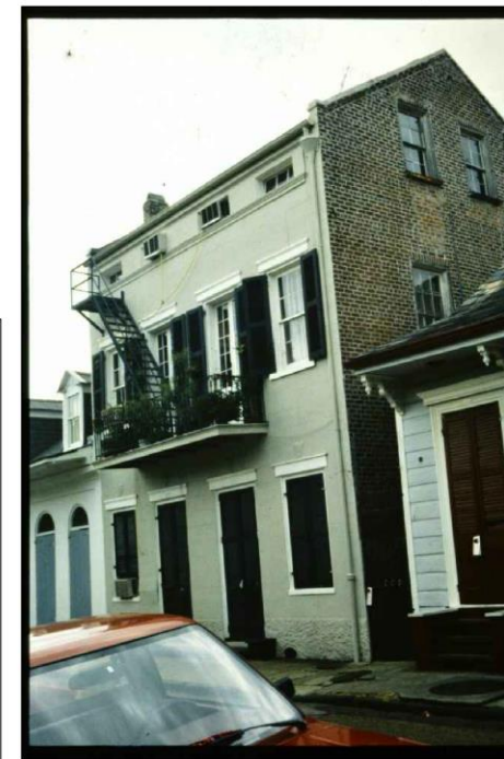
VCC Library Photo of 1008 Dauphine, 1991 This image shows square/stepped trim at the bottom of the frieze band, which we believe is closer to the historic condition.
