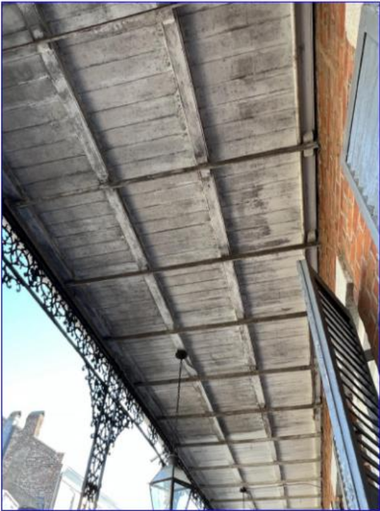
REFERENCE PHOTO OF PORCH CEILING.
