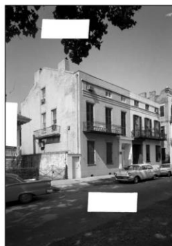
810 Esplanade, NOLA Greek Revival Frieze Band Windows with stepped/square trim elements
