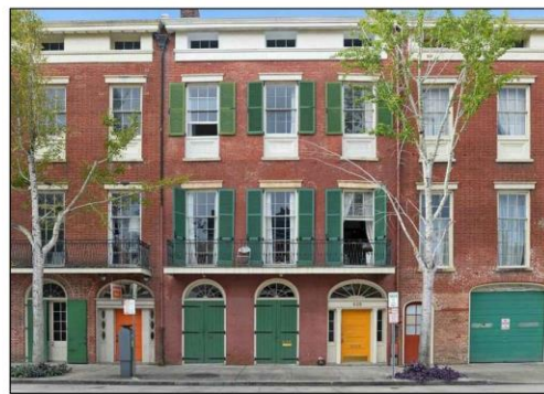
Julia Row, NOLA Greek Revival Frieze Band Windows with stepped/square and dentil trim elements
