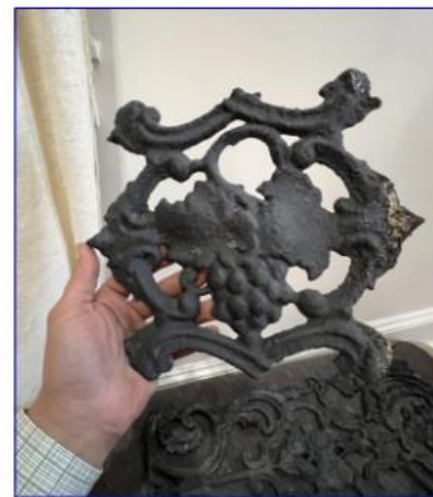
REFERENCE PHOTO 5.3 IRON PIECE FOR THE MID PART. REPAIR NO.2
