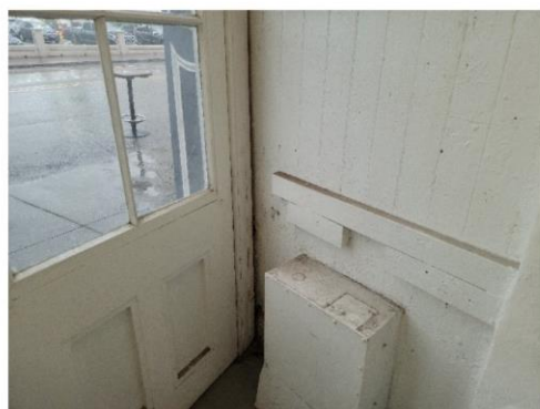
Another view of the left front corner on the first floor
