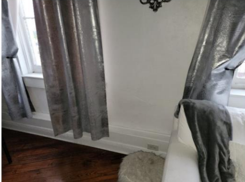
Another view of the front wall in Unit No. 4
