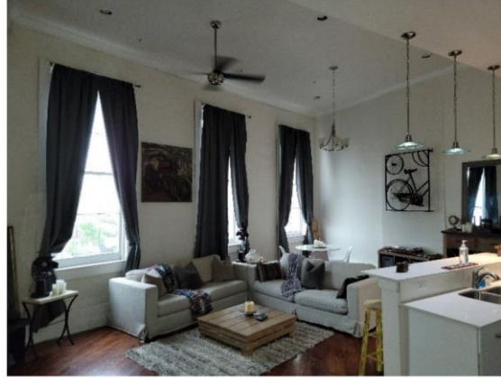
Overview of the inside of the front wall in Unit No. 1 on the left side of the second floor
