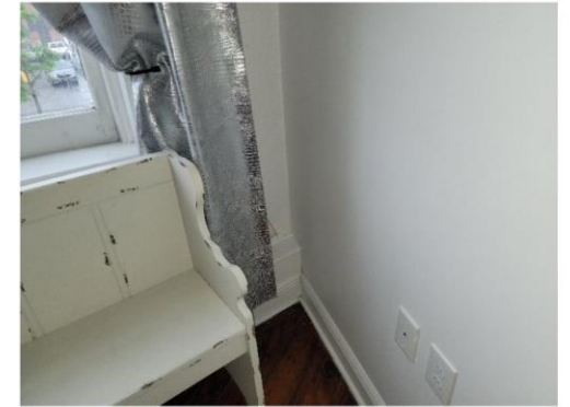
View of the left front corner of Unit No. 4
