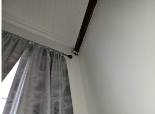
Another view of the left front corner of Unit No. 4
