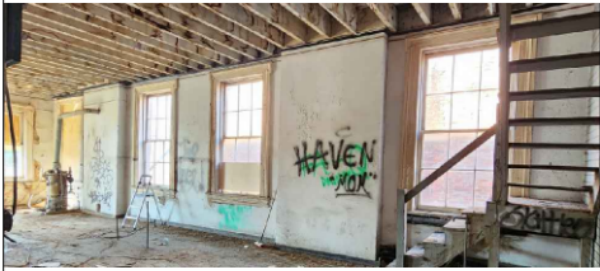
3RD FLOOR - SIDE WINDOWS- QTY 4 EACH FLOOR
