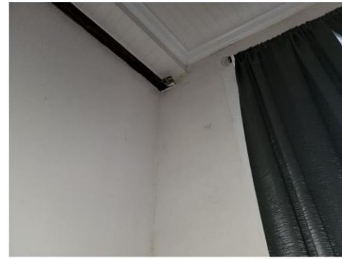
View of the right front corner of Unit No. 1
