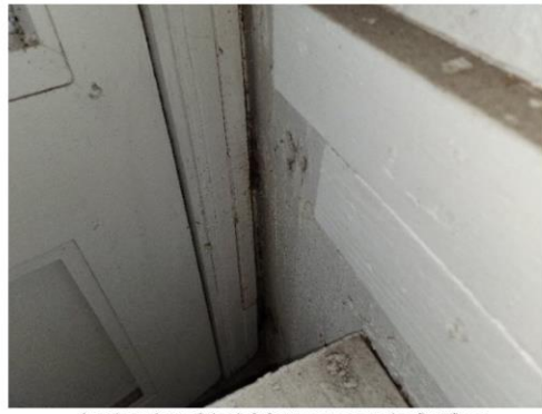
Another view of the left front corner on the first floor
