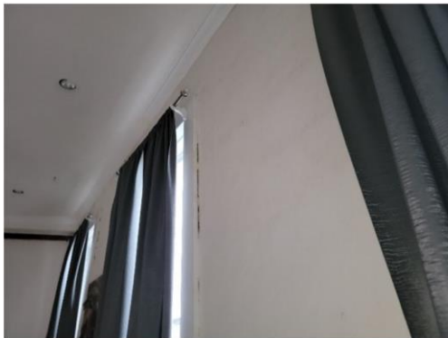
Another view of the separations between the trim and the front wall of Unit No. 1
