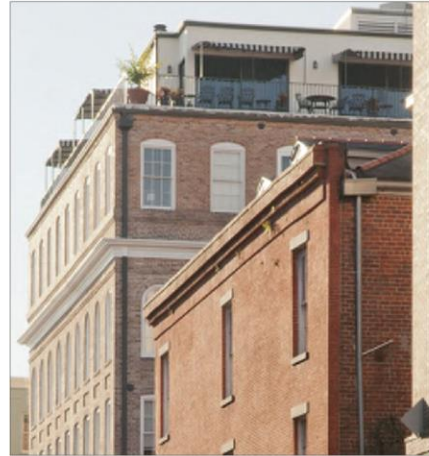
This rooftop addition is set back from the building corner on both sides and has a flat roof without permanent projecting overhangs. The metal railing is nominally visible to pedestrians.
