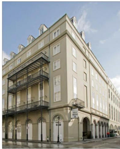
A first floor remnant of the old St. Louis Hotel remains to the right. In 1960, a larger hotel was constructed, incorporating the remnant, with compatible arched ground floor openings and storefront cornice.
