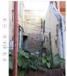
7 BOWING @ MASONRY WALL SCALE: NOT TO SCALE
