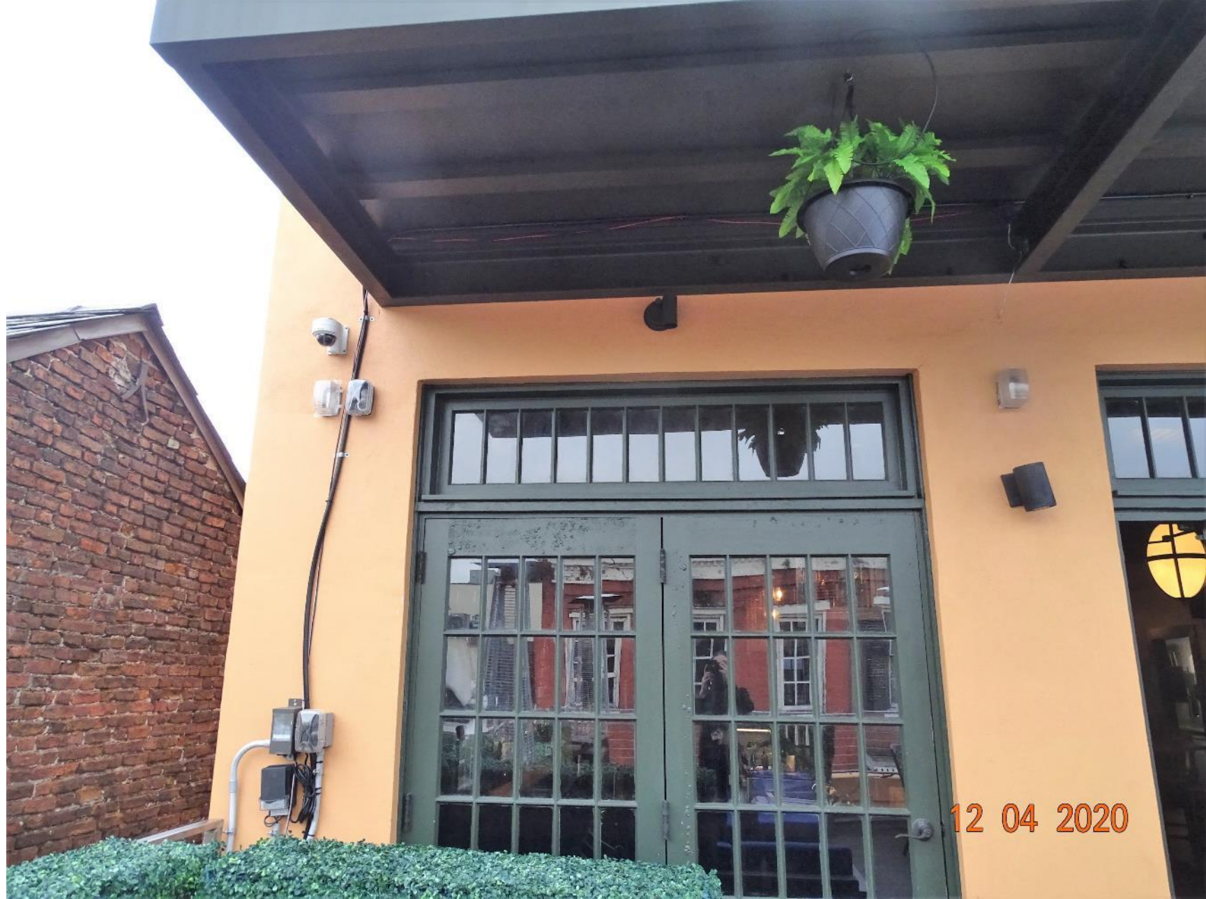
411 Bourbon – Roof Deck Awning – As Built
