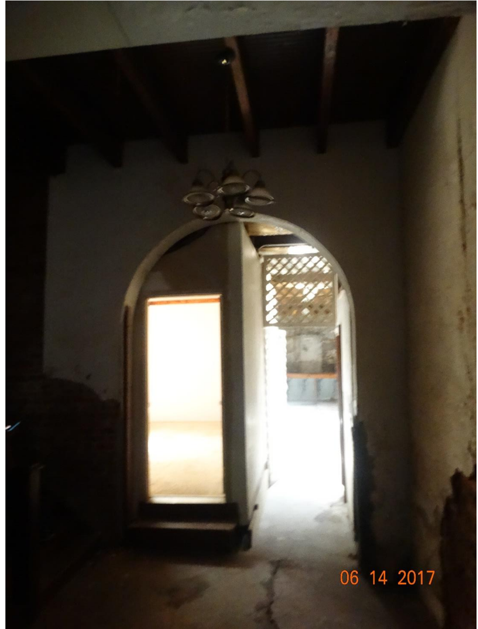
622 N Rampart – existing archway at rear of main building
