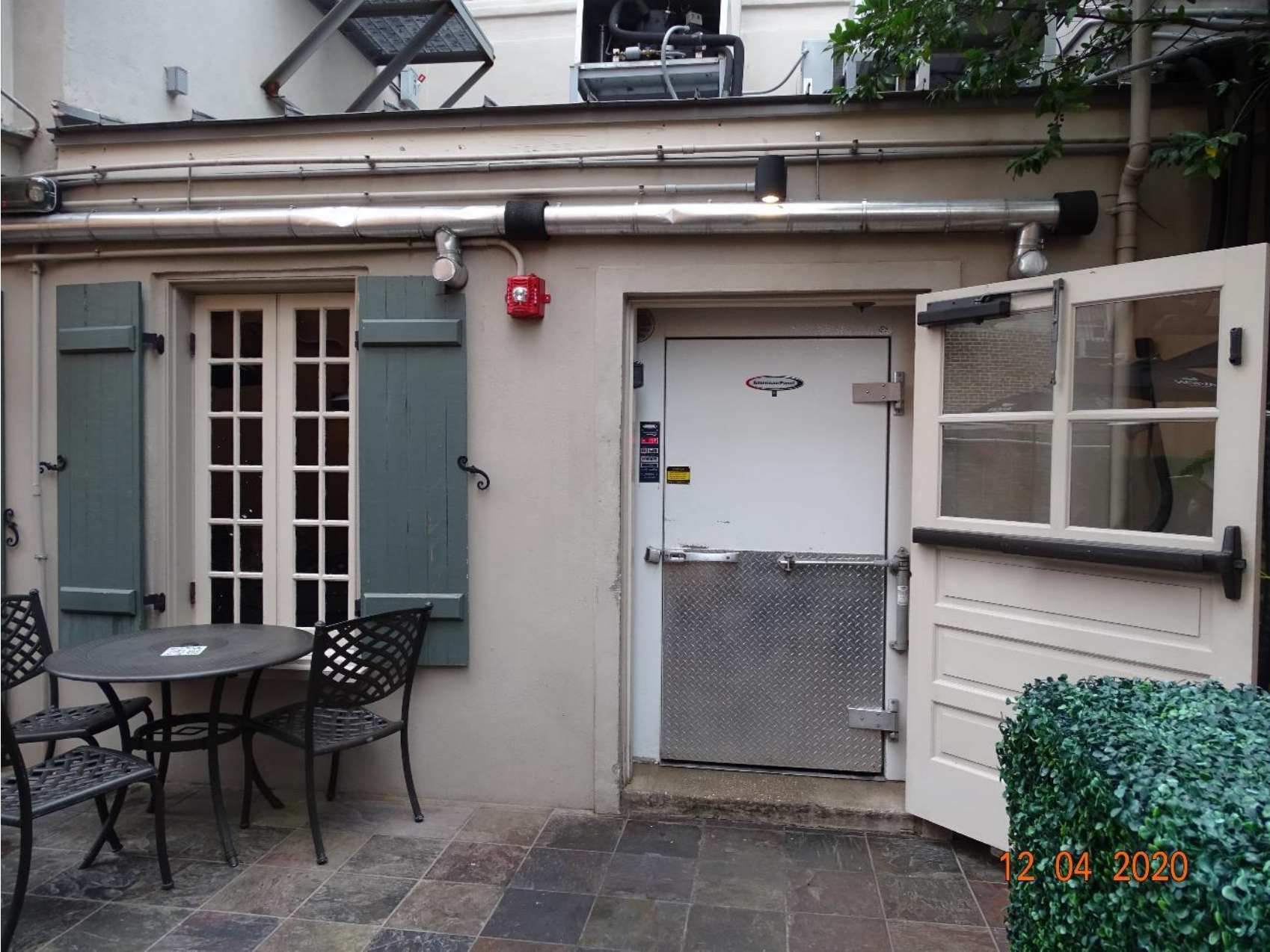
411 Bourbon – Walk-in Door – Rear Building – As Built
