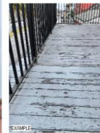
REPAIR BALCONY TO ADDRESS HAZARDOUS WALKING CONDITION
