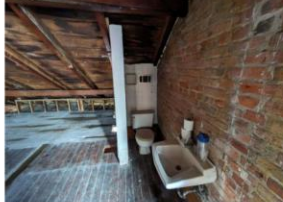
Existing plumbing fixtures to be demolished
