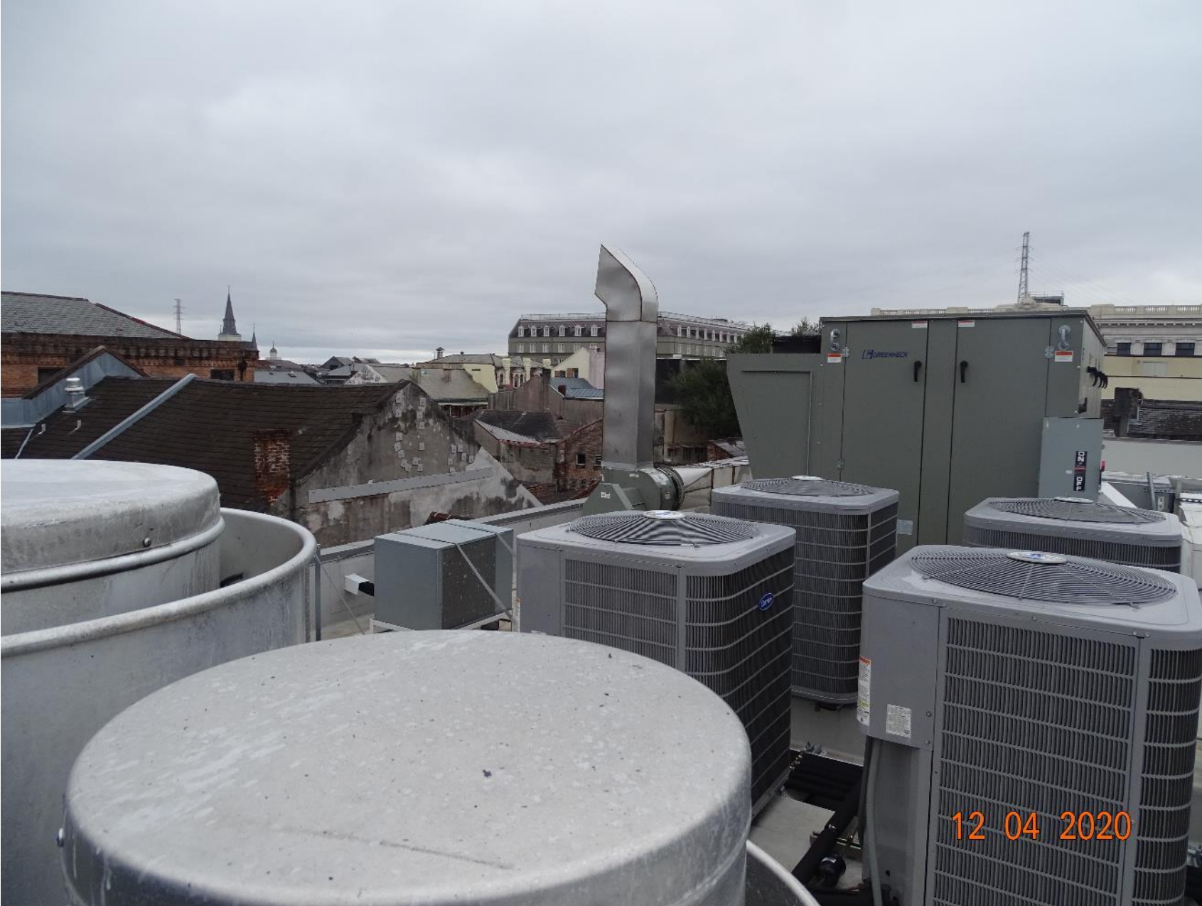
411 Bourbon – Mechanical Equipment – Main Building – As Built – Fourth Floor Roof
