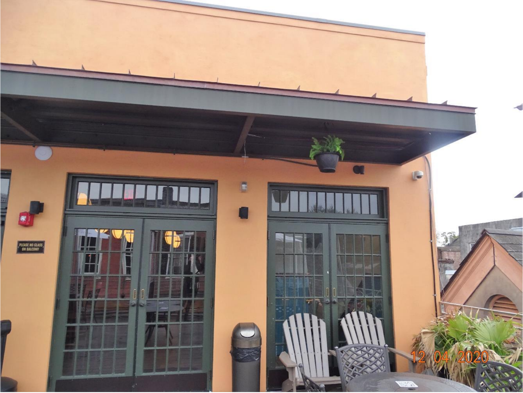
411 Bourbon – Roof Deck Awning – As Built
