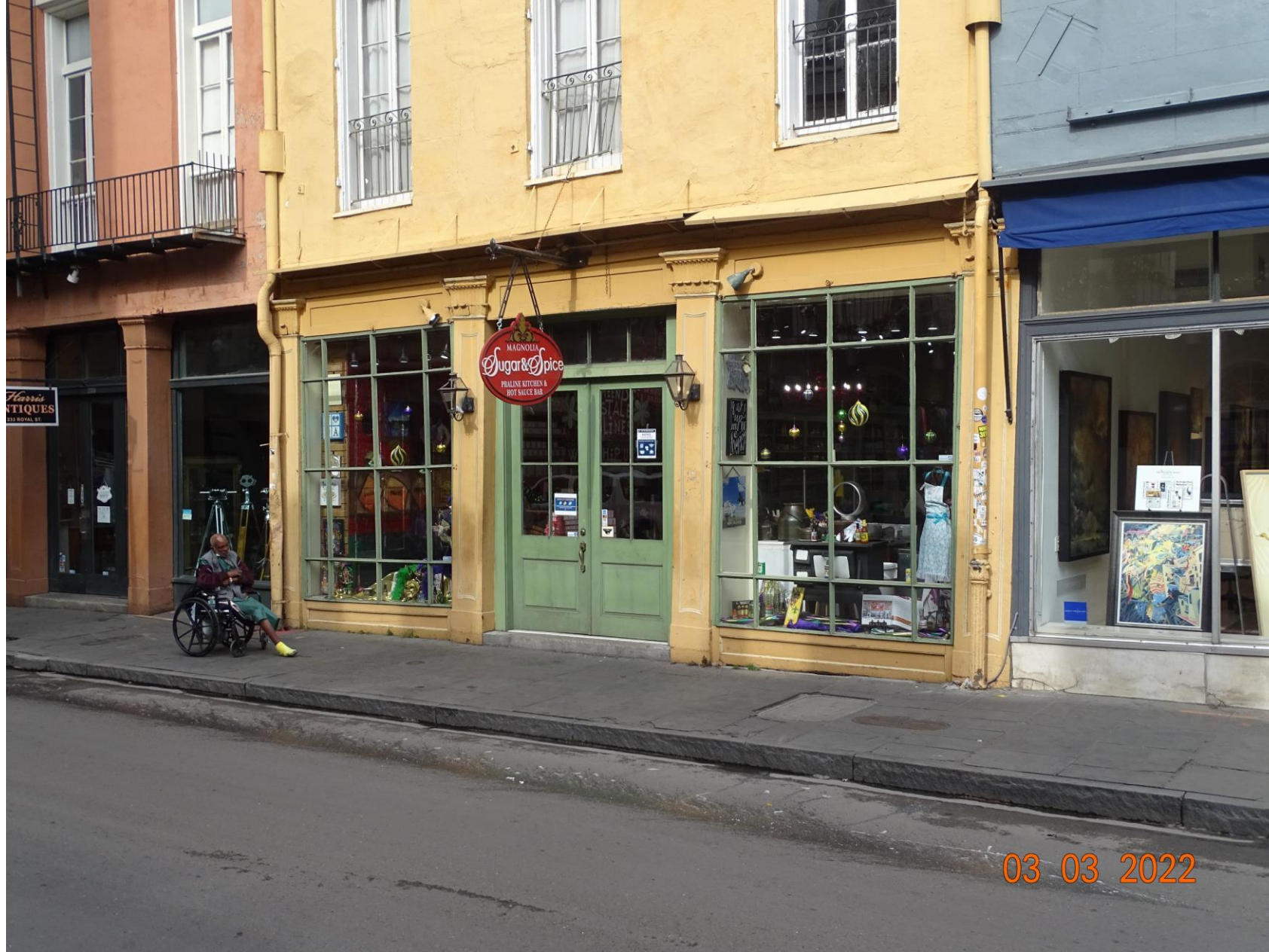
229 Royal – Neighboring Buildings
