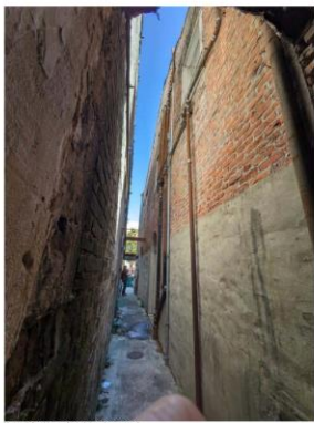
Unseal plumbing and conduit to be removed
