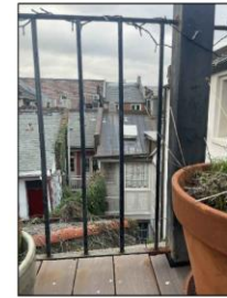
PHOTO of EXISTING RAIL
