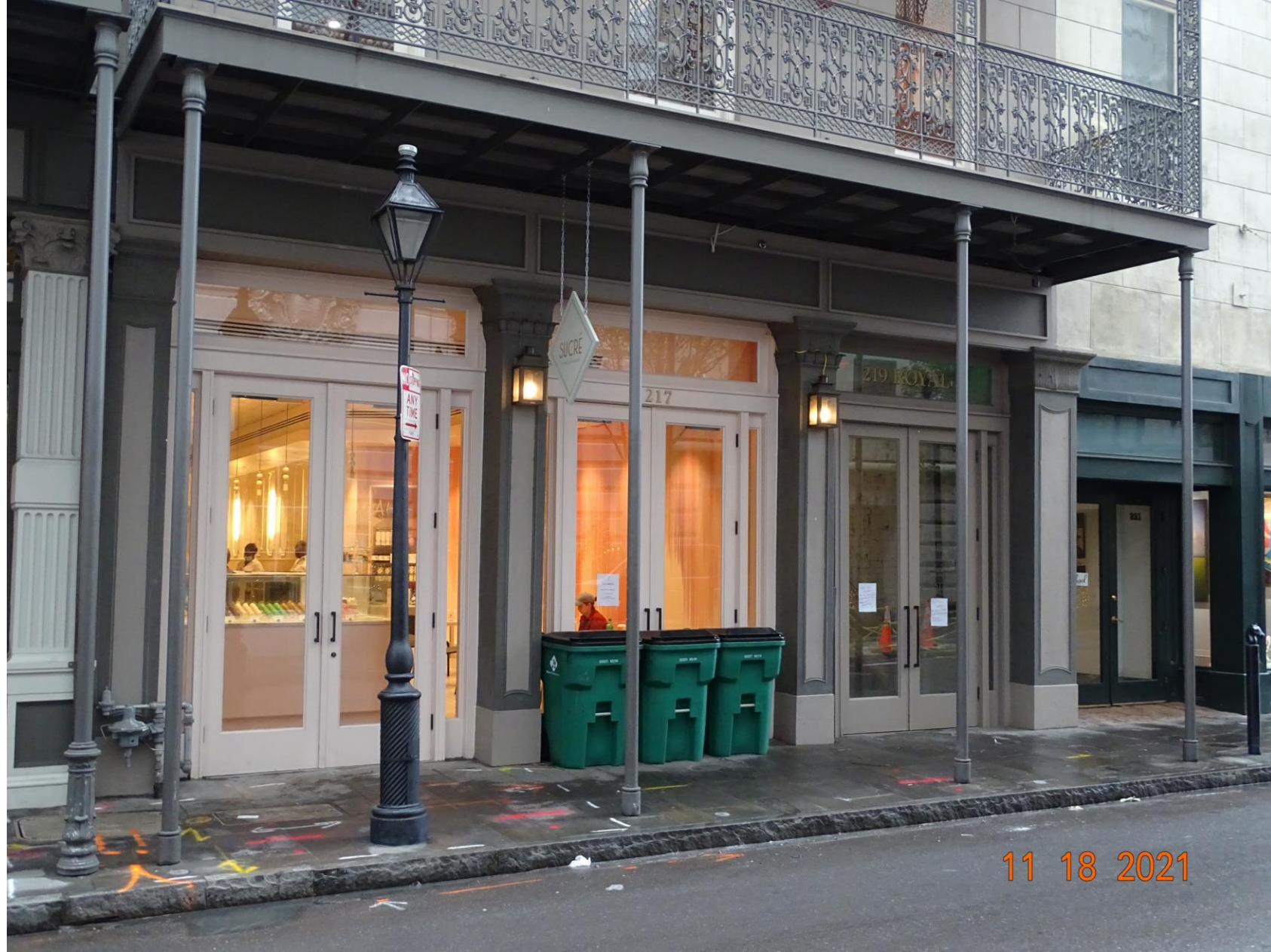
229 Royal – Neighboring Buildings
