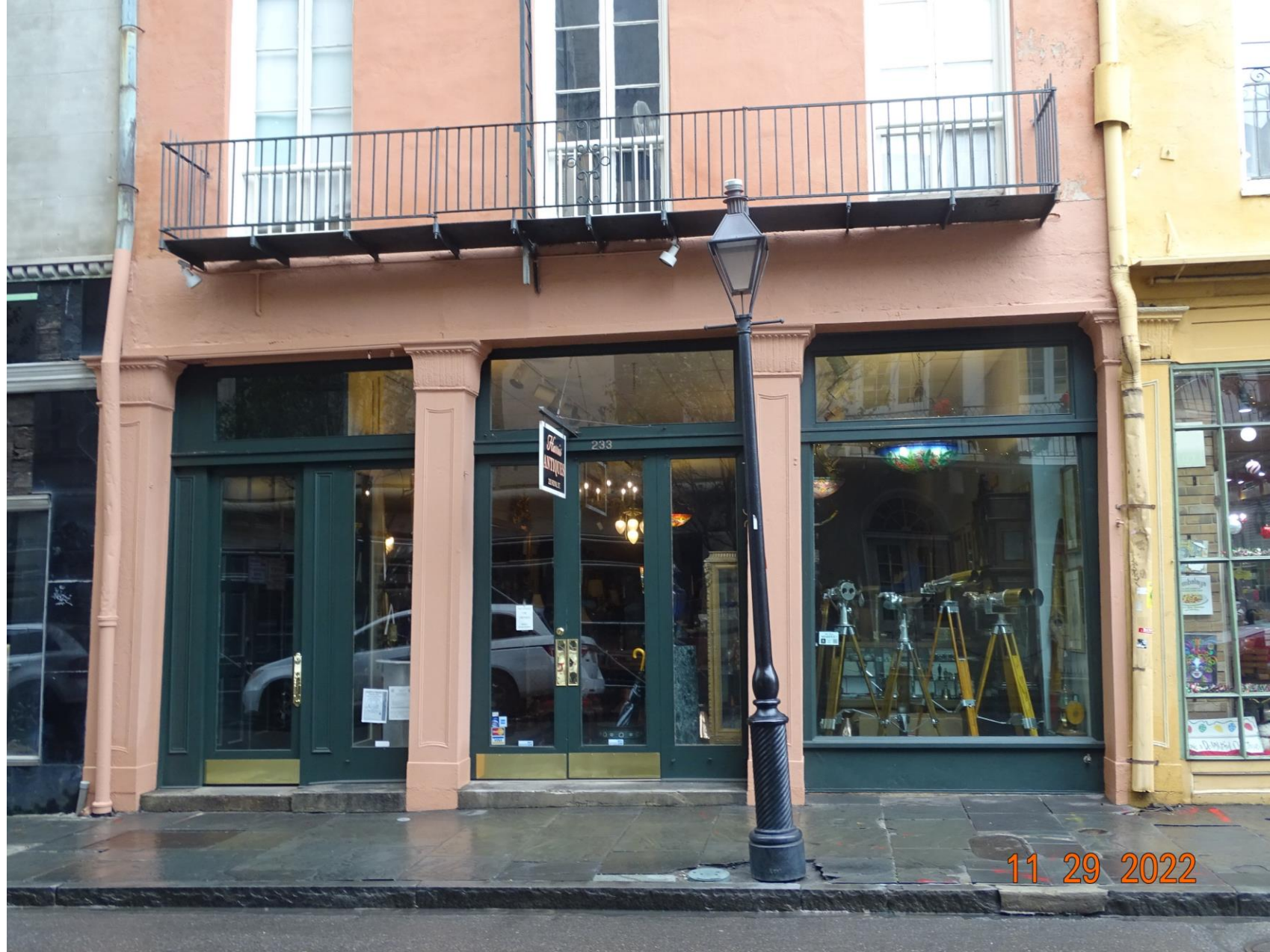
229 Royal – Neighboring Buildings
