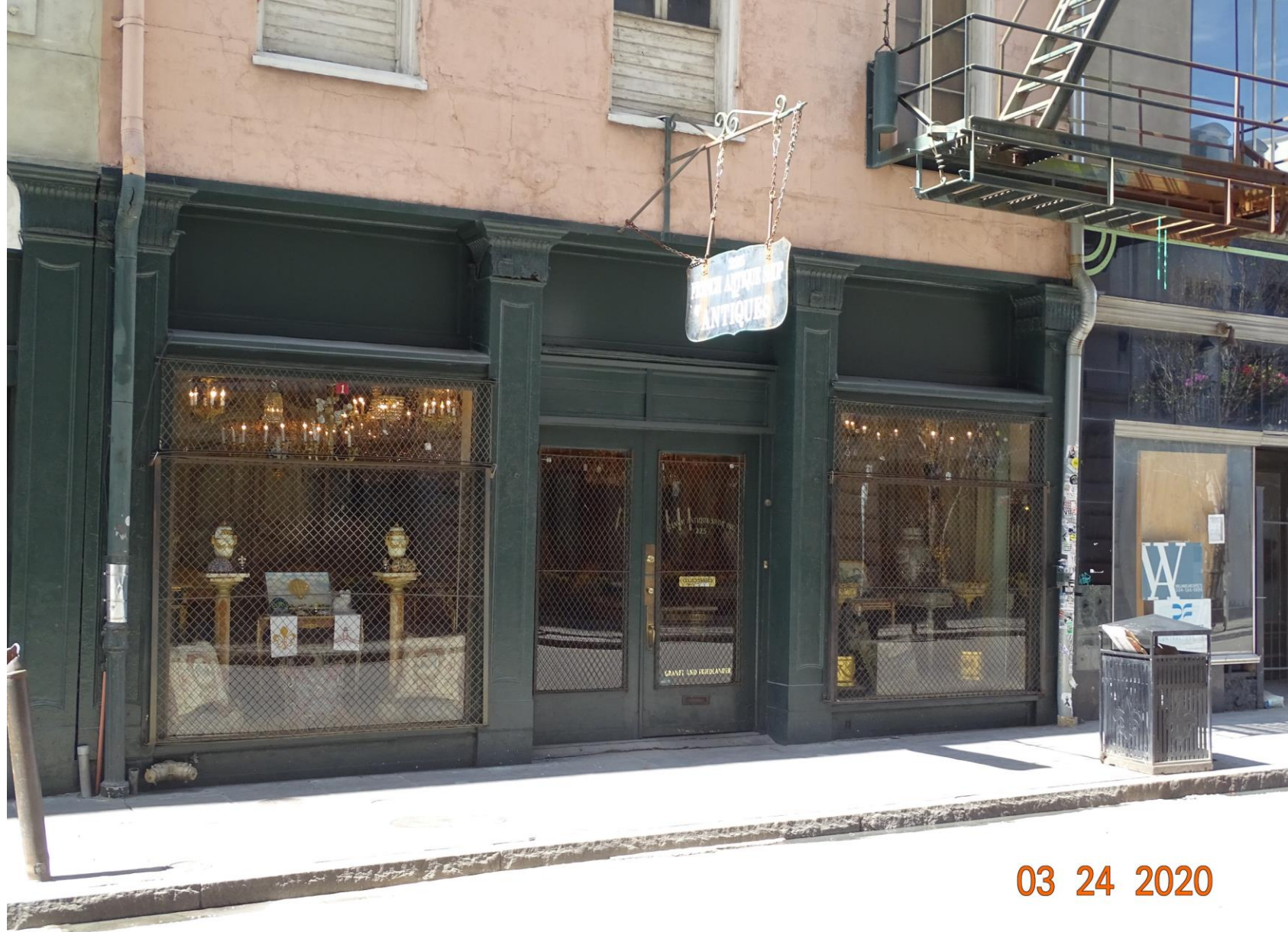
229 Royal – Neighboring Buildings
