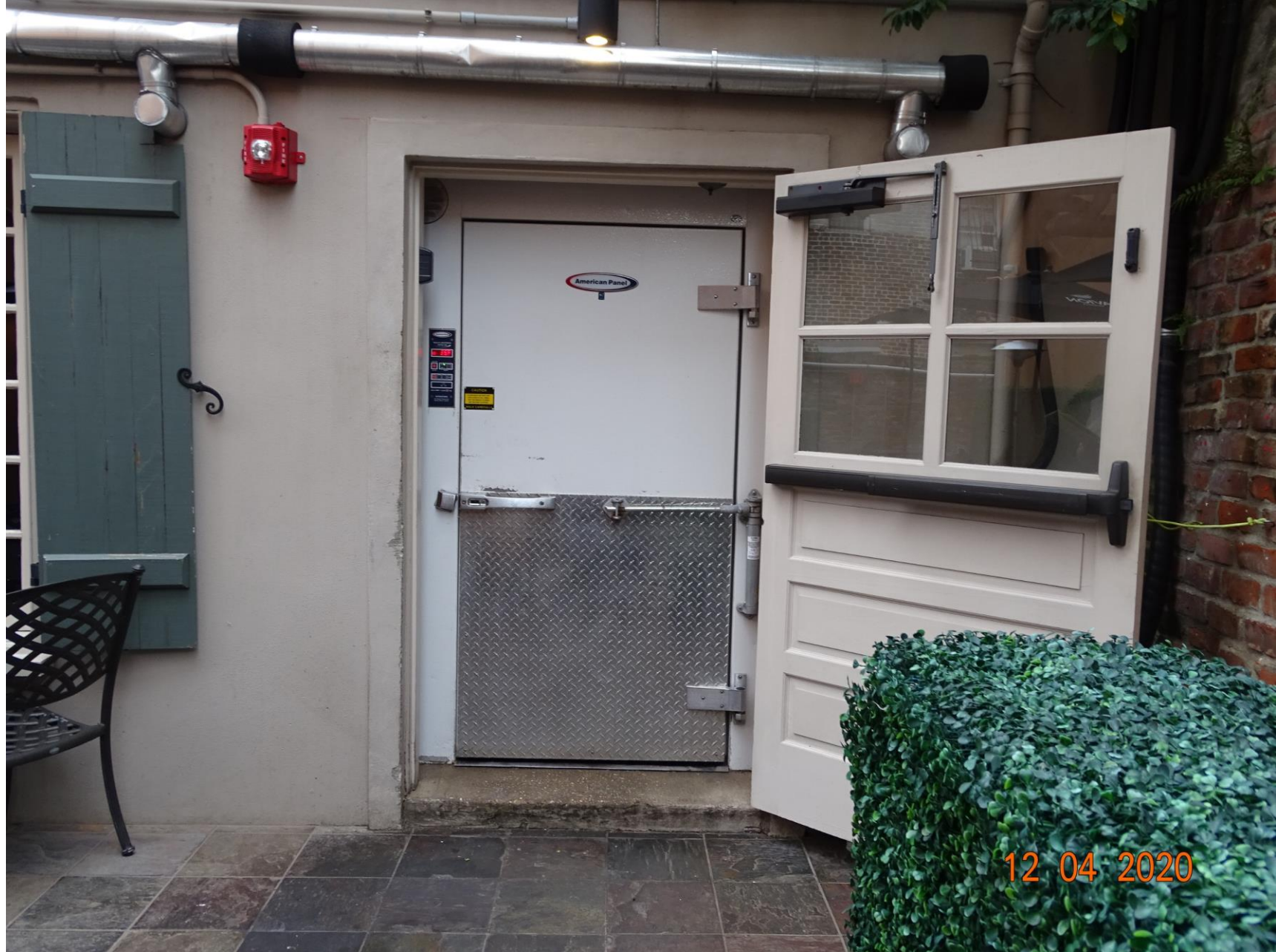
411 Bourbon – Walk-in Door – Rear Building – As Built
