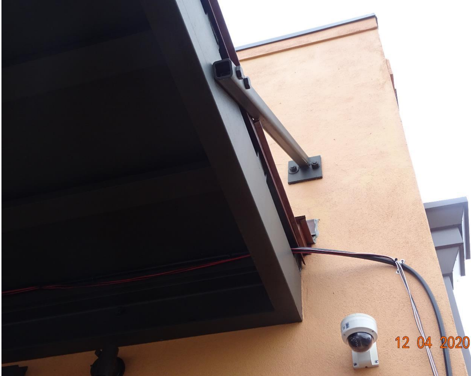
411 Bourbon – Roof Deck Awning – As Built
