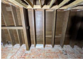
Beams to be demolished per plans. GC to provide all necessary temporary bracing
