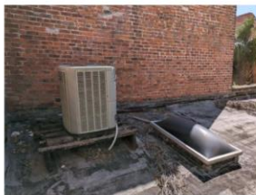
Existing condenser on roof. Roof to be demolished, condenser to relocate
