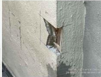
Showing Apex Construction Sample Area
