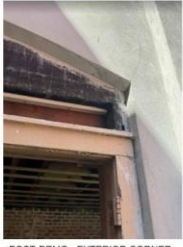
POST-DEMO - EXTERIOR CORNER
