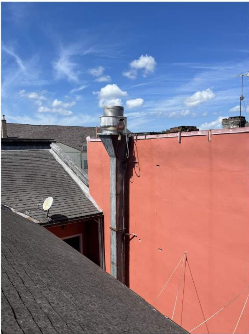
EXISTING HOOD TO BE REPLACED
