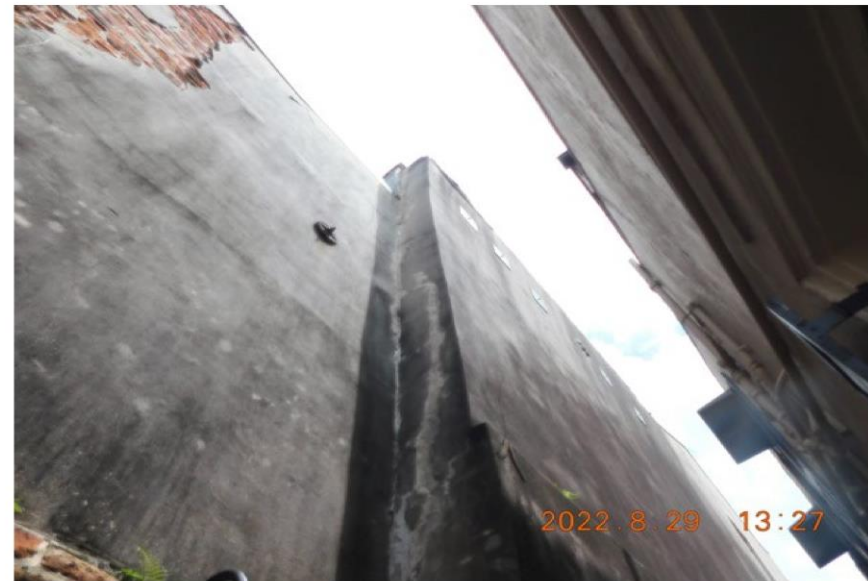
View of Exterior Wall from 1129 Burgundy Street
