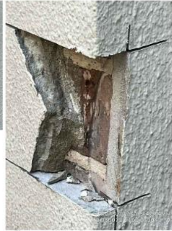
Close-up Apex Construction Sample
