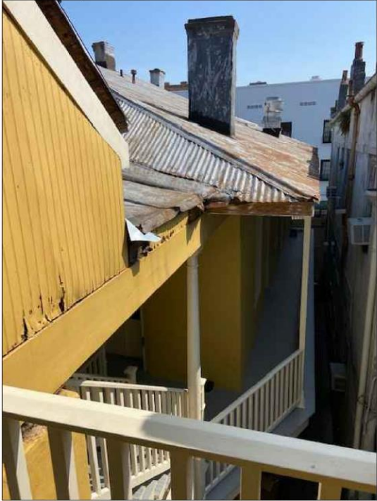
10 roof repair and replacement
