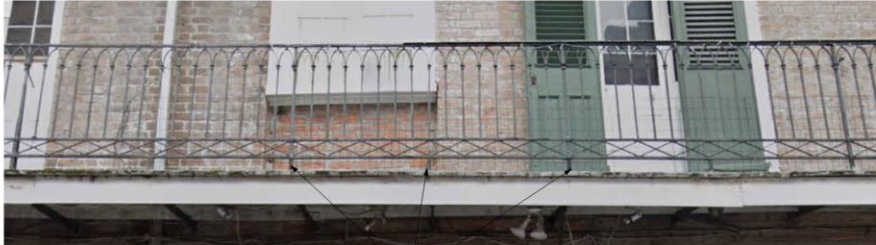
VERTICAL SUPPORT, ALIGN NEW GUARDRAIL VERTICAL SUPPORT IN-LINE, TYP. RAILING AT ST ANN ST.
