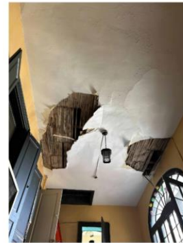
8 TYPICAL CEILING AT STAIRWELL
