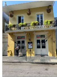
14 signage attached to building
