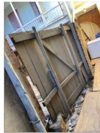
3 new vertical board fence
