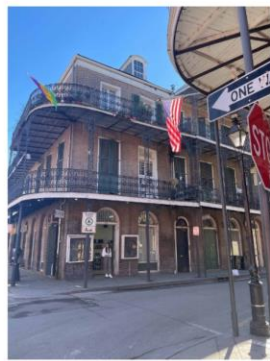
2 ROYAL ST & ST ANN CORNER FACADE
