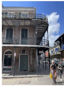
3A ST ANN CORNER FACADE
