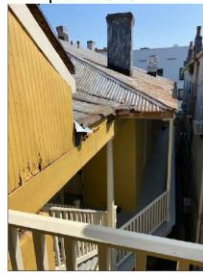
10 roof repair and replacement
