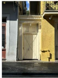
1 new metal gate
