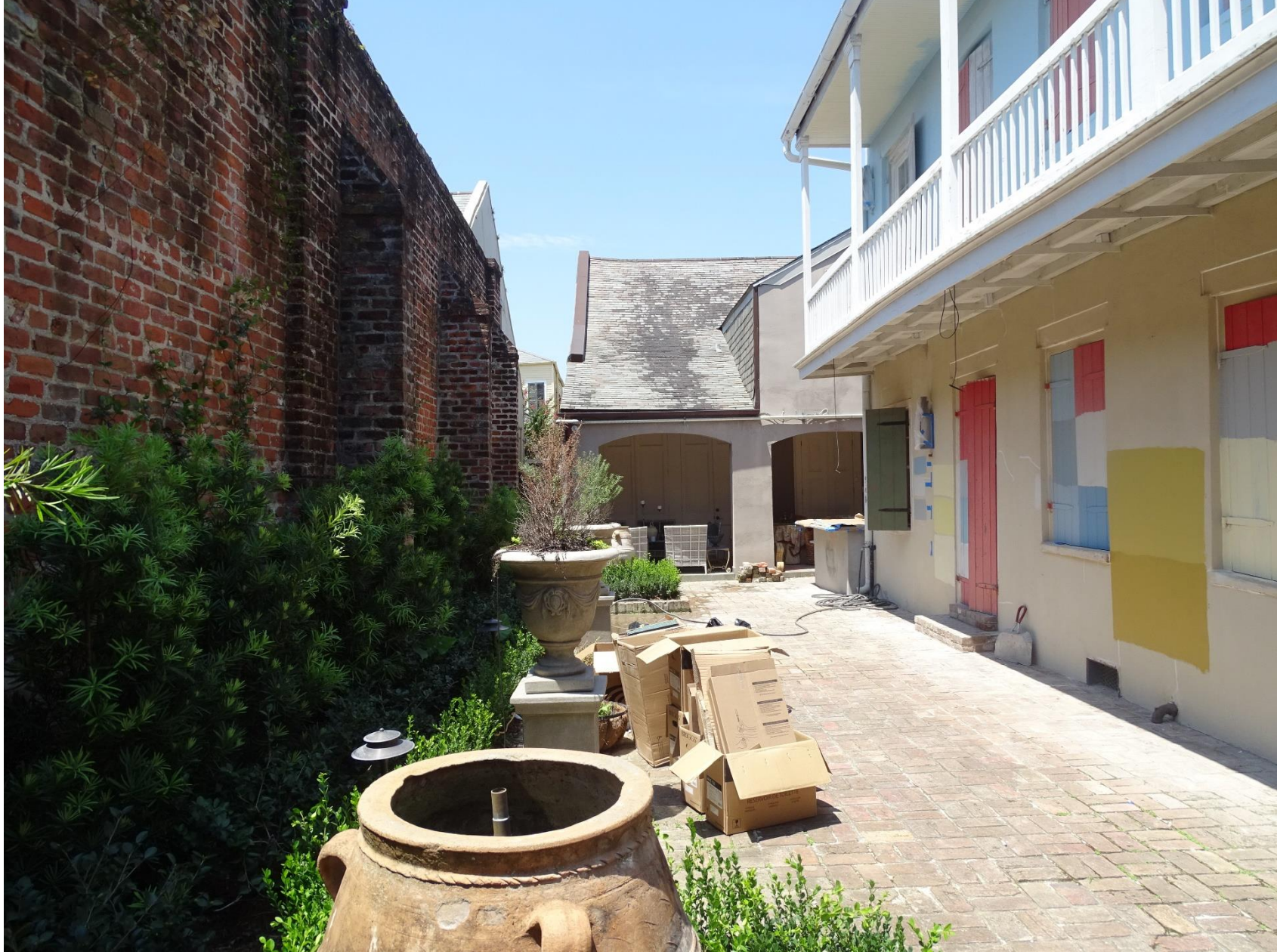
1118 Burgundy – unpermitted exterior kitchen
