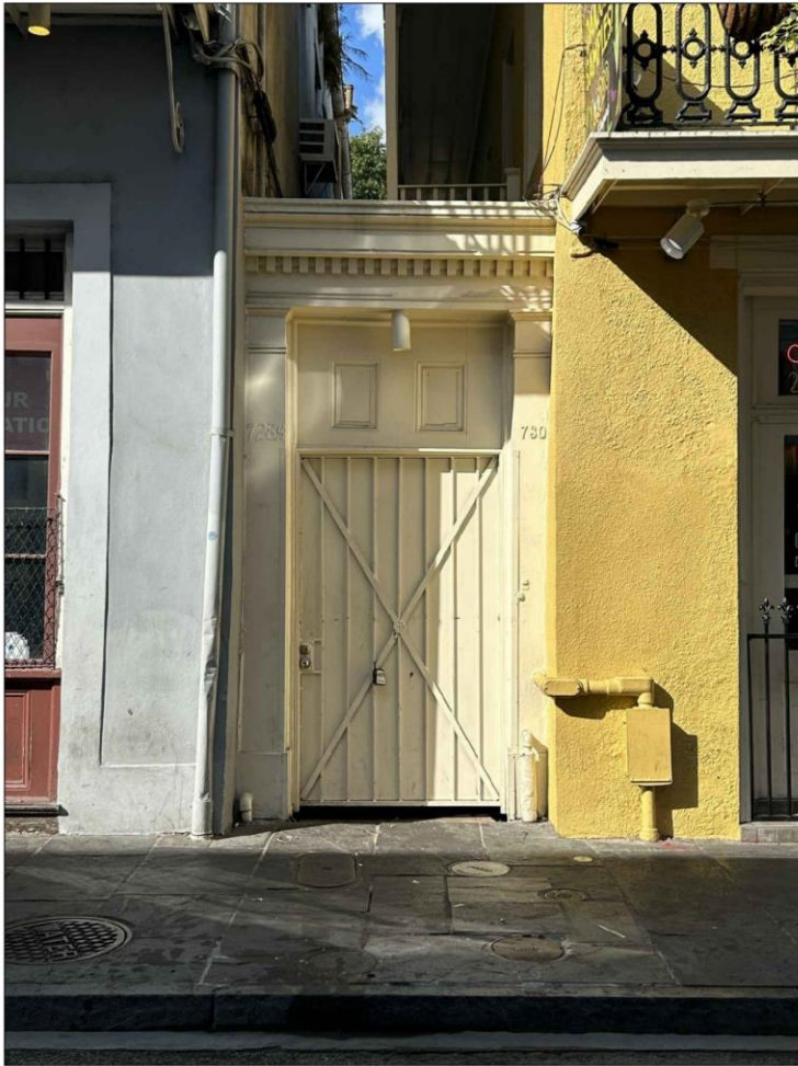
1 new metal gate
