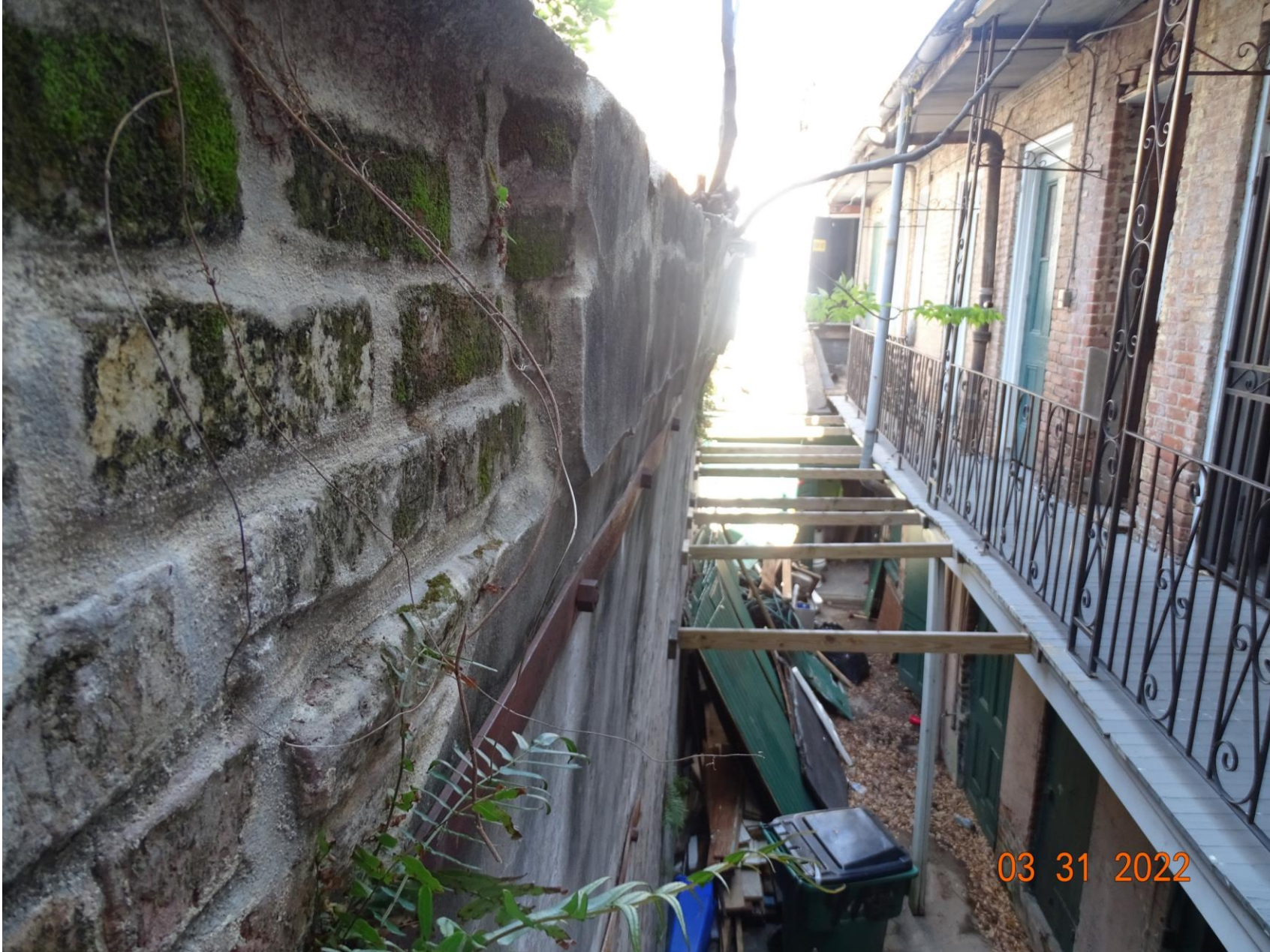
416 Bourbon – courtyard wall at 418 Bourbon
