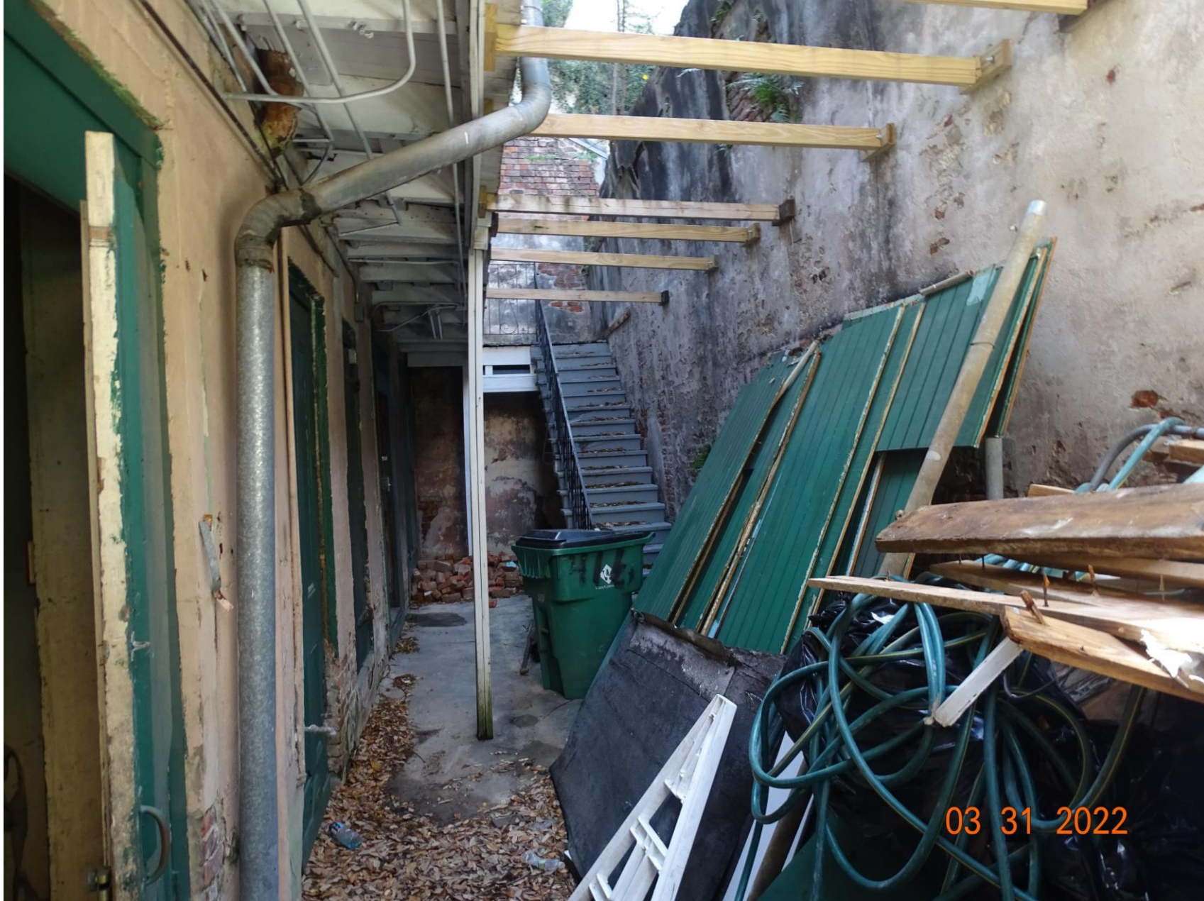
416 Bourbon – courtyard wall at 418 Bourbon
