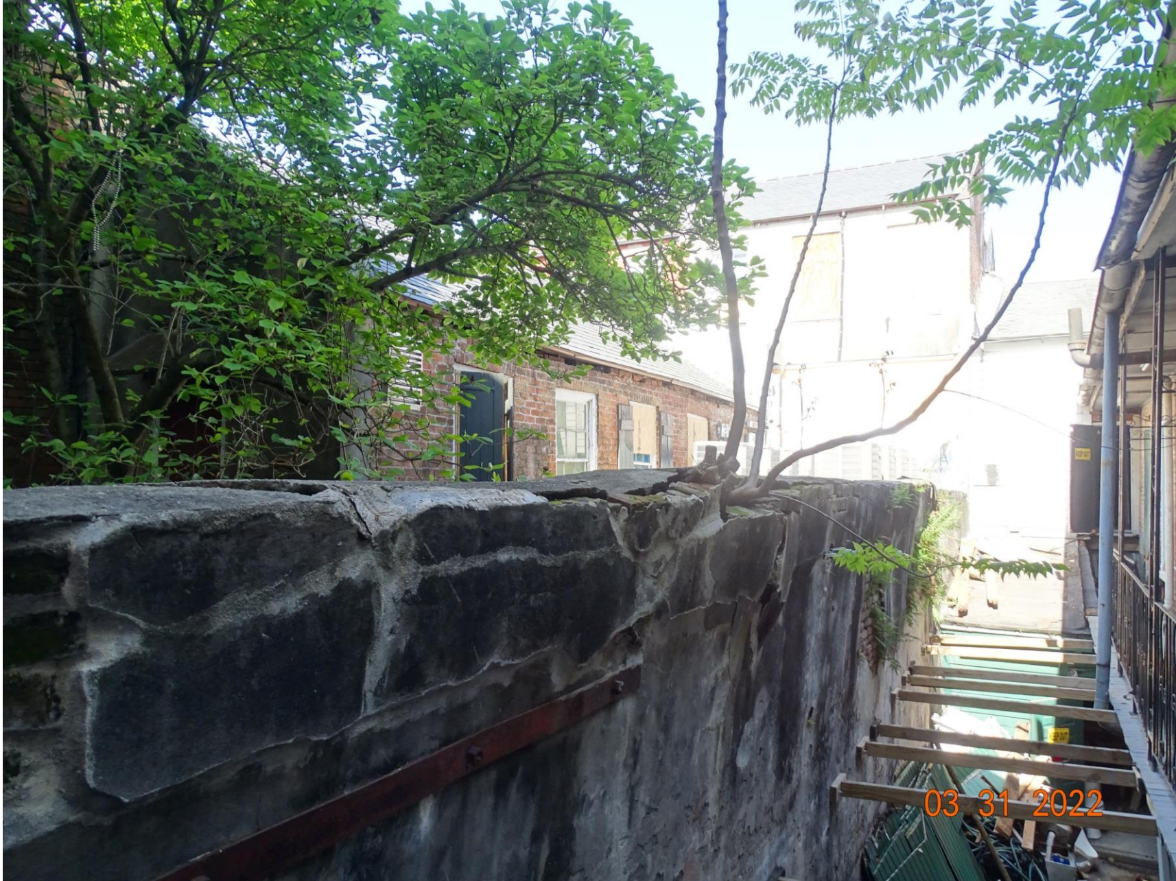
416 Bourbon – courtyard wall at 418 Bourbon
