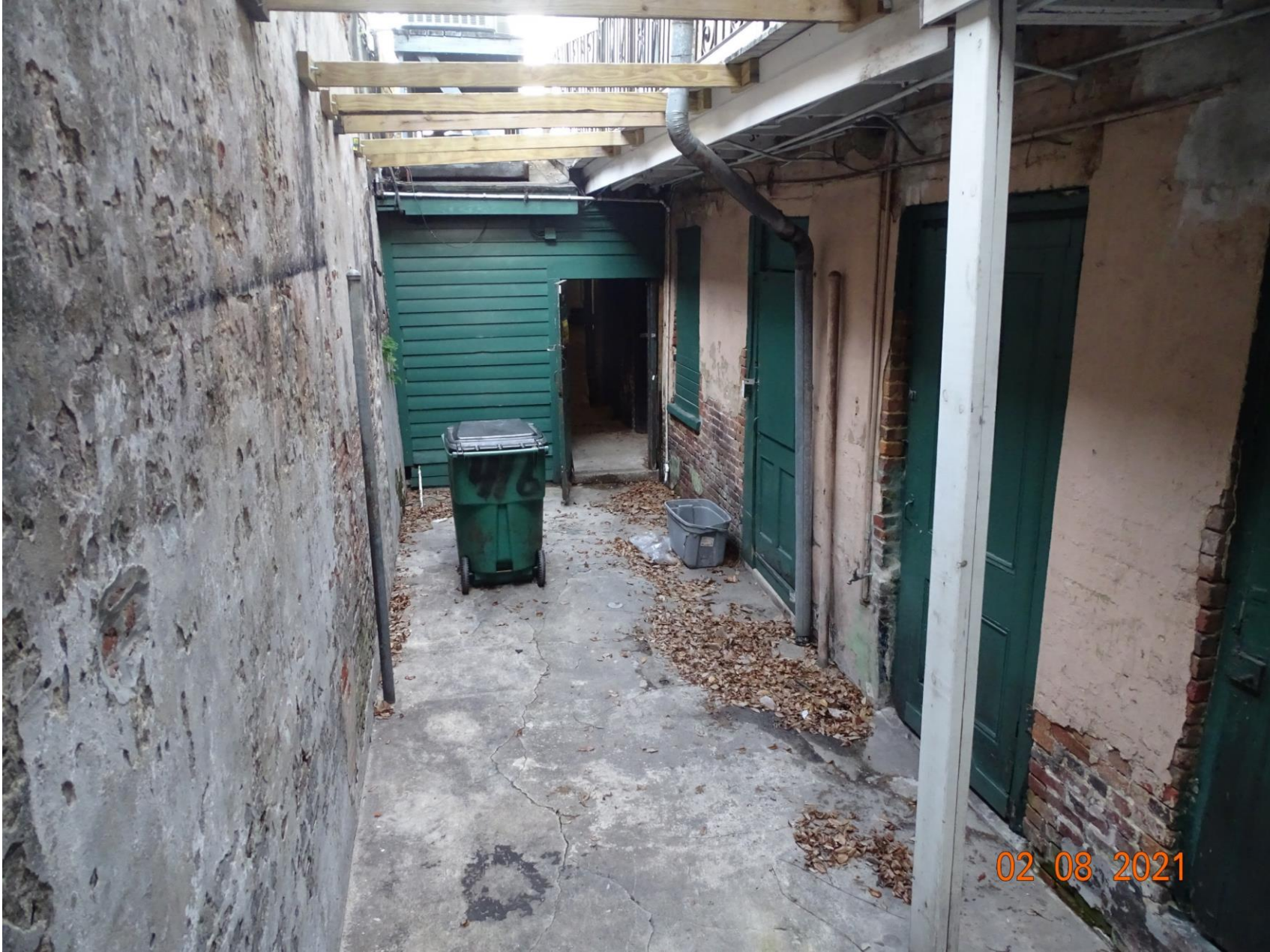
416 Bourbon – courtyard wall at 418 Bourbon
