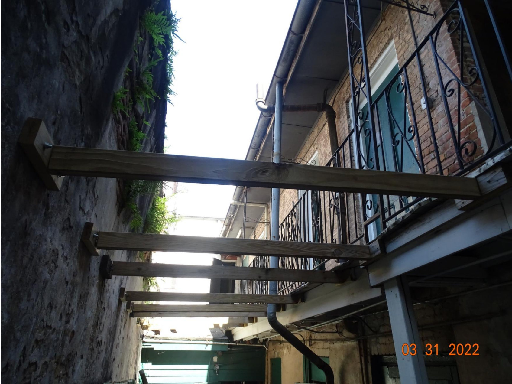
416 Bourbon – courtyard wall at 418 Bourbon
