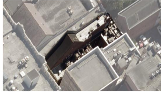
EXISTING CONDITION - ROOFTOP EQUIPMENT
