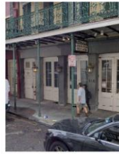
EXISTING CONDITION - FRONT FACADE
