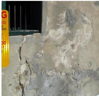
Rear of Service Building
