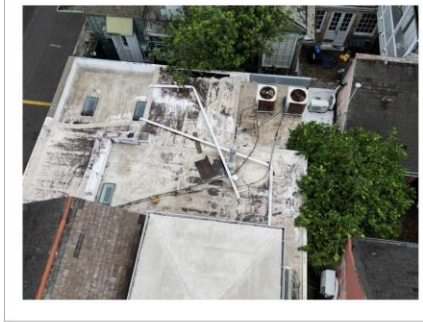
AERIAL VIEW OF EXISTING ROOF
