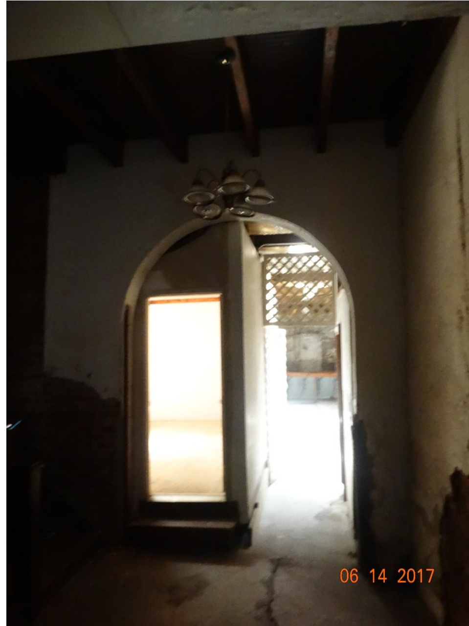
622 N Rampart – existing archway at rear of main building
