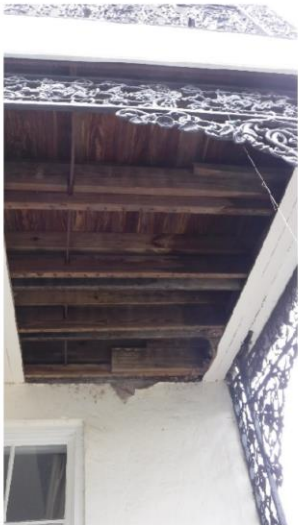
Photo 2: View at underside of 3rd floor
