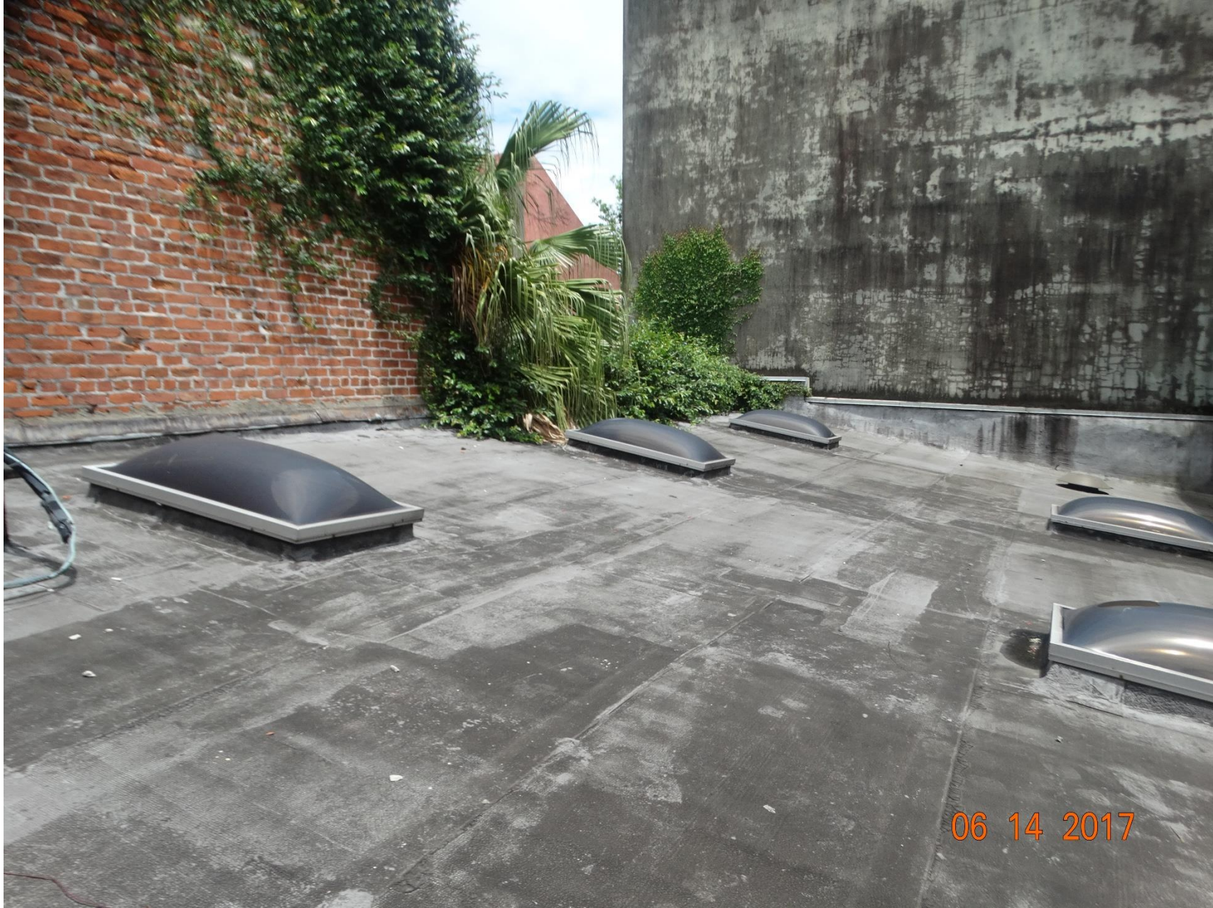
622 N Rampart – existing brown-rated roof
