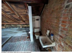
Existing plumbing fixtures to be demolished
