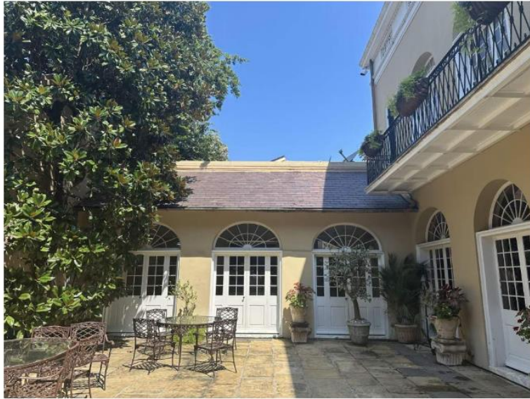
VIEW FROM RIVER-SIDE COURTYARD
