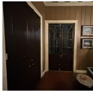
INTERIOR PHOTO OF EXISTING DOOR
