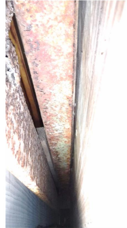
Photo 5: Steel channel along front of balcony
