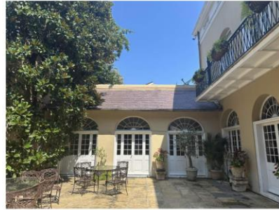
VIEW FROM RIVER-SIDE COURTYARD
