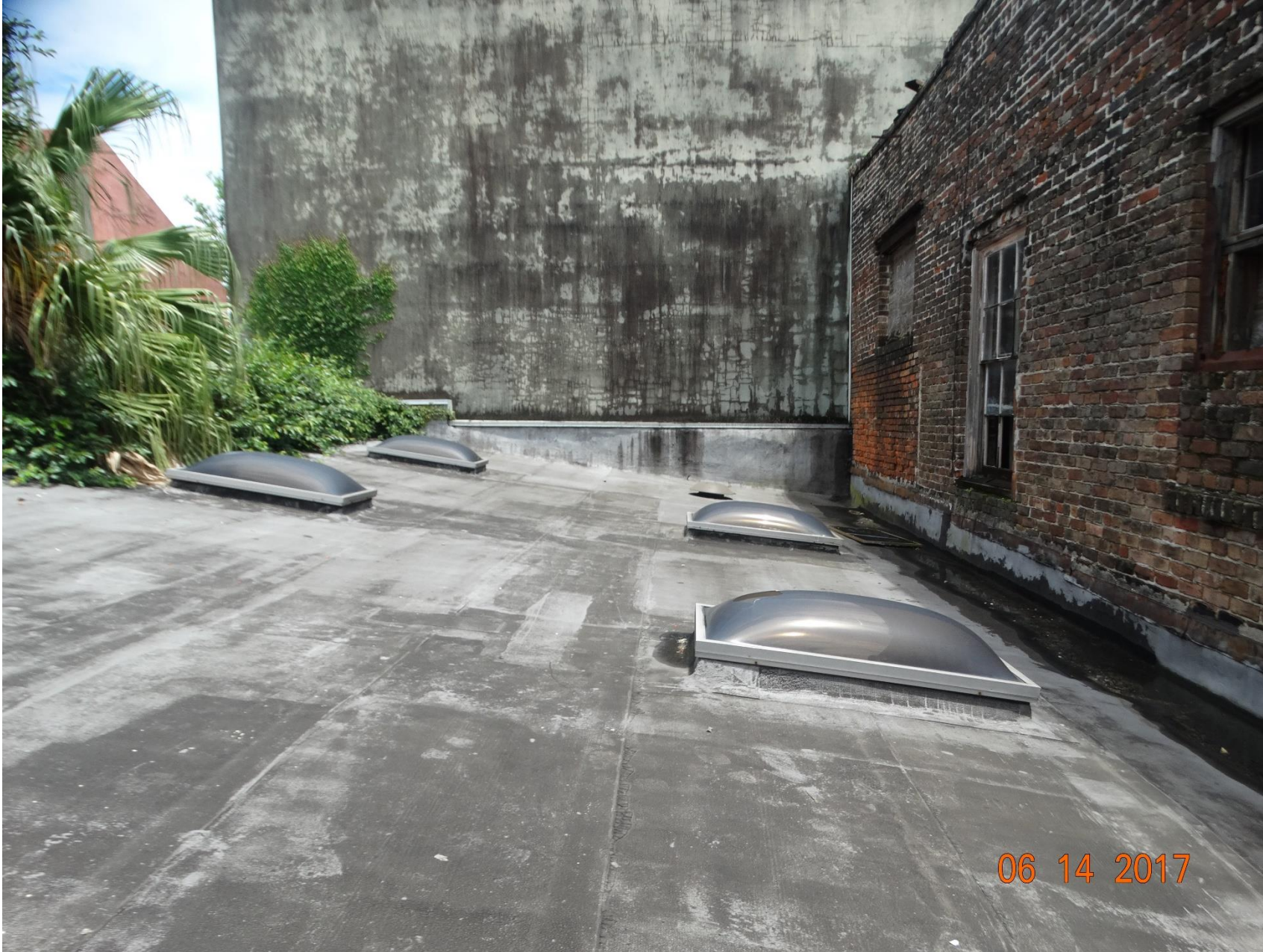
622 N Rampart – existing brown-rated roof
