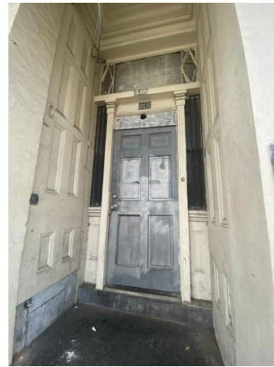
PHOTO OF DOOR ALONG RAMPART STREET
