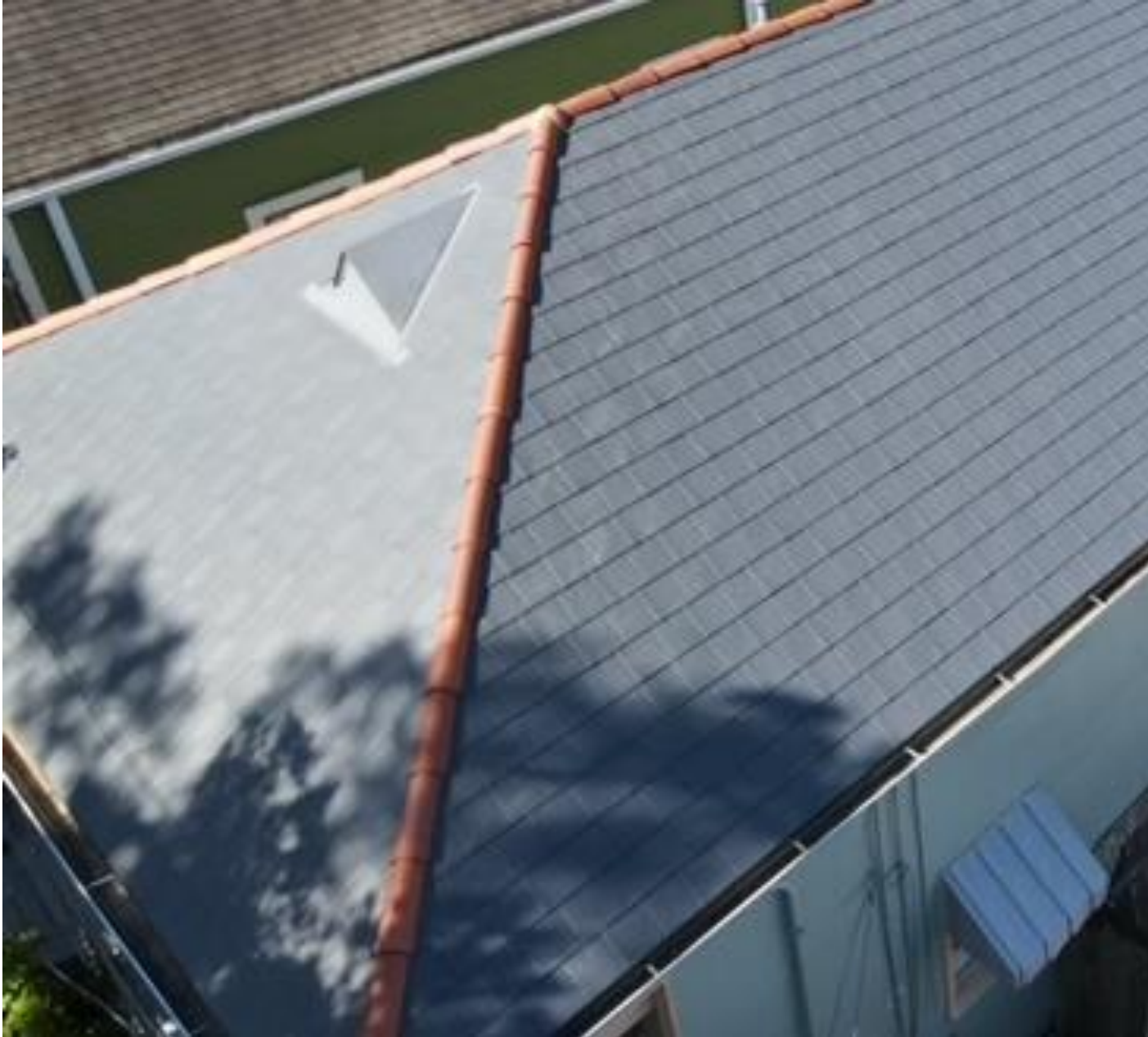
910 Bourbon – Same material on a roof at 509 Olivier
