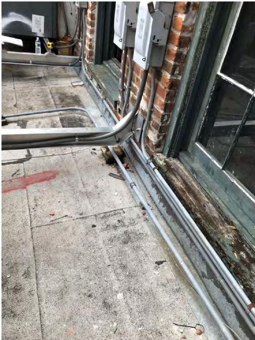
typical support beam at wall of main building
