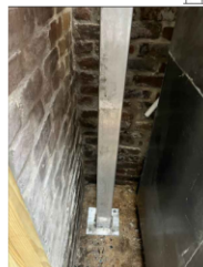
Existing Column Base
