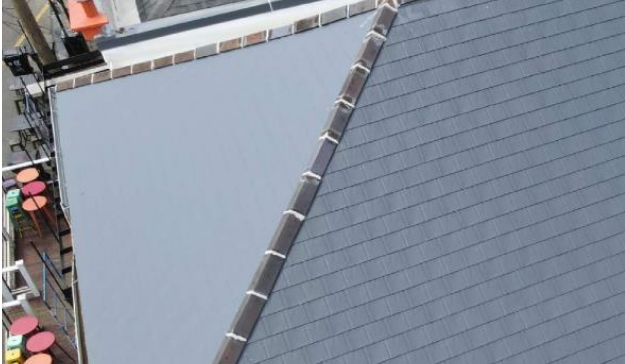
910 Bourbon – Same material on a roof in the Marigny
