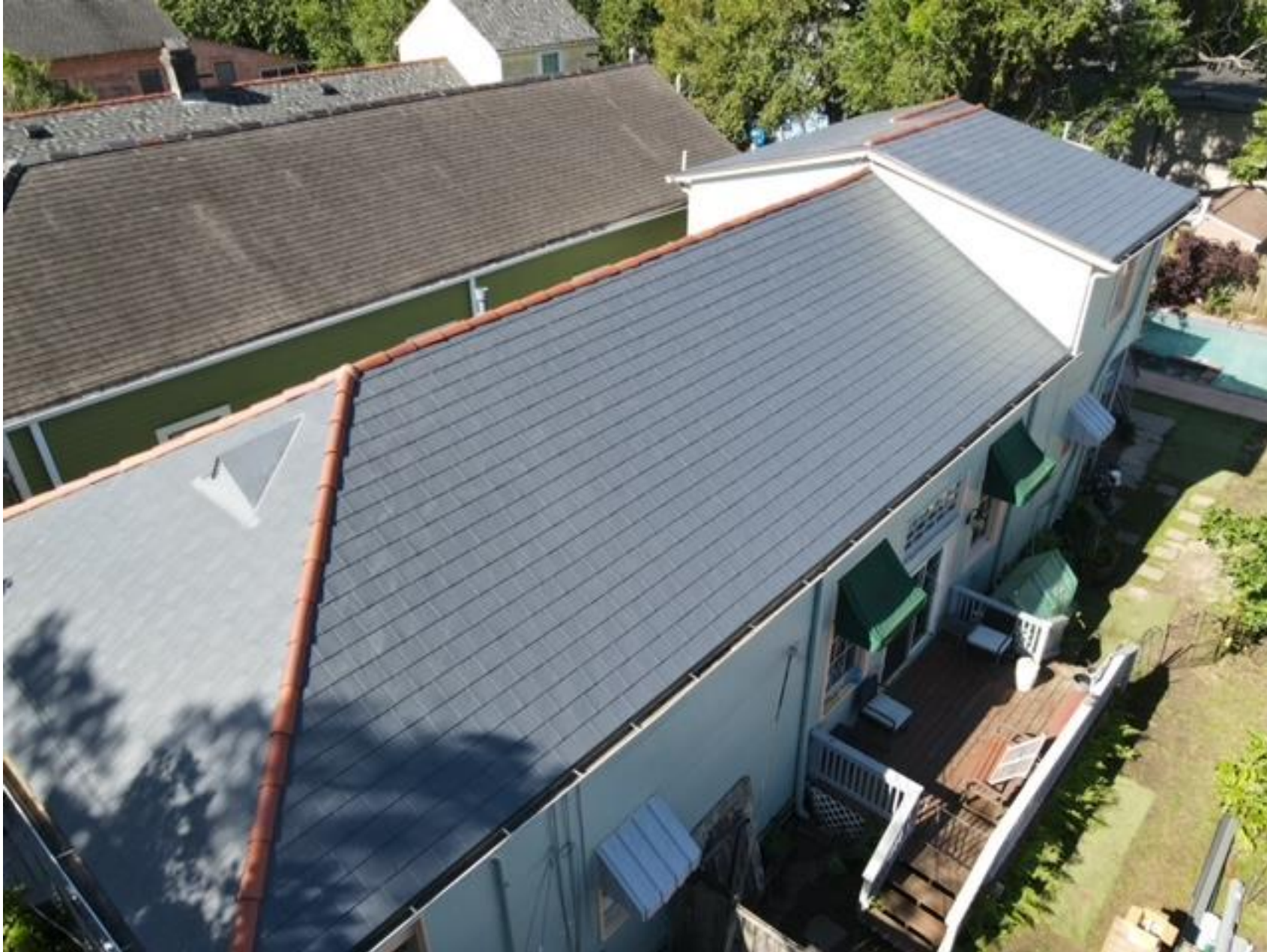
910 Bourbon – Same material on a roof at 509 Olivier
