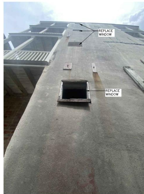
PHOTO OF REAR WALL
