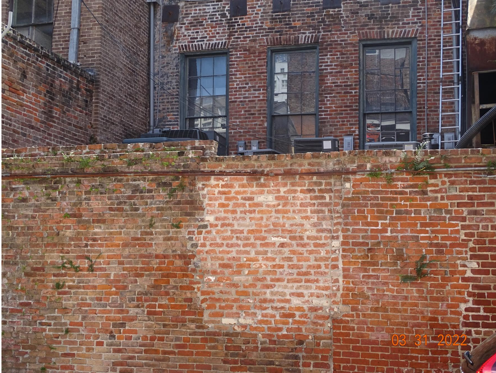
209 Decatur – previous conditions
