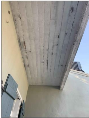
4 REPAIR & REPAINT SOFFIT OVER REAR BALCONY
