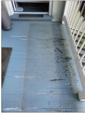
3 REPLACE ROTTEN DECKING AT REAR BALCONY
