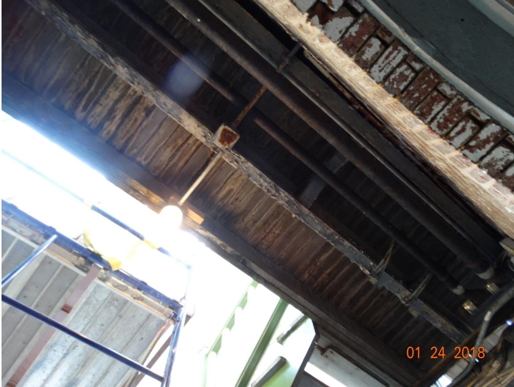
828 Bourbon – Underside of Rear Balcony
