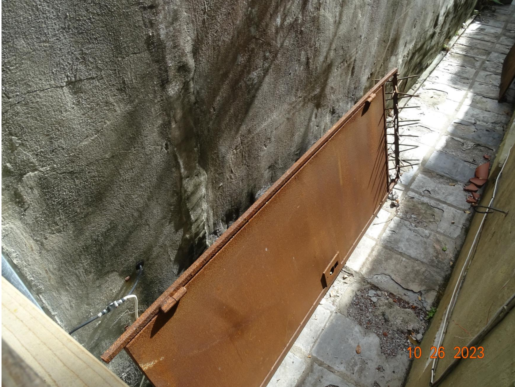
1030 St Philip – previous gate
