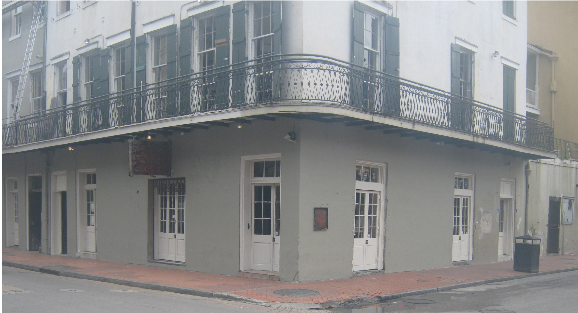
235-41 Bourbon – 2010 Repairs in Progress
