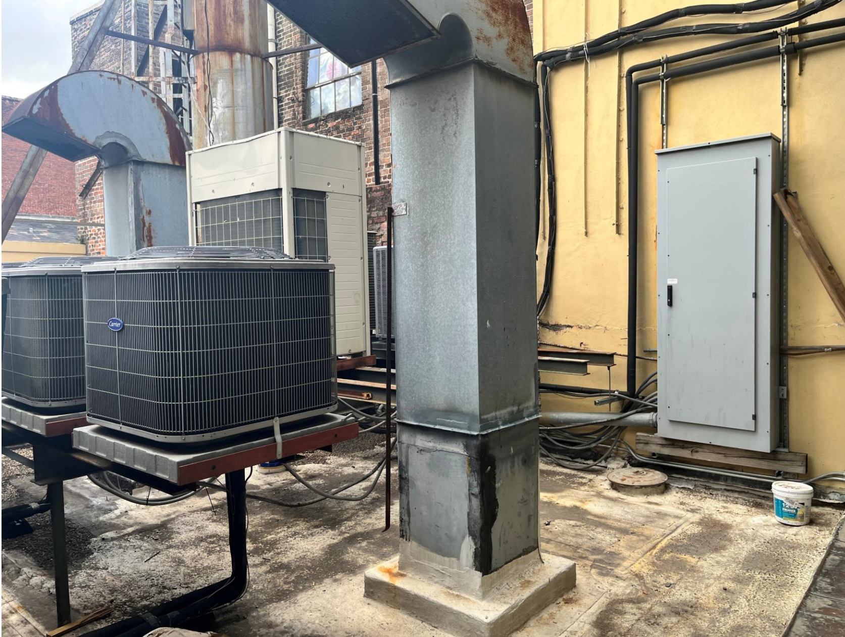
719 St. Louis – Area in need of rail
