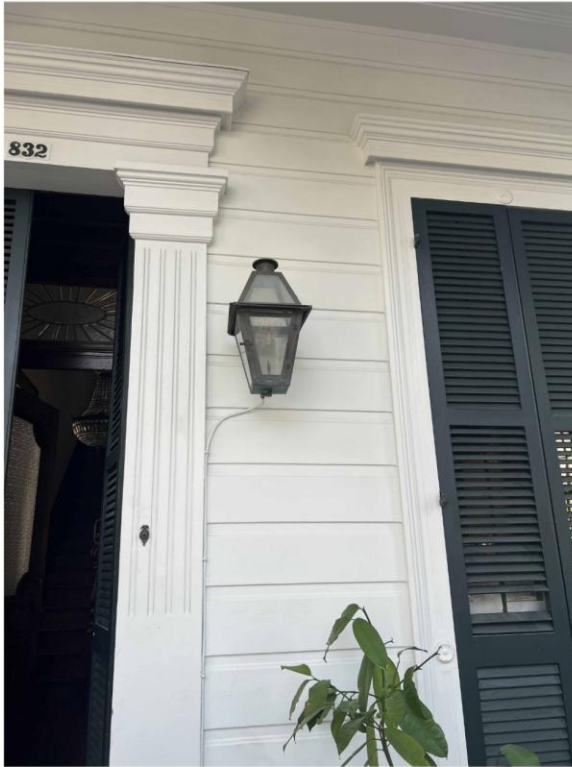
PHOTO A (EXISTING GAS LANTERN)
