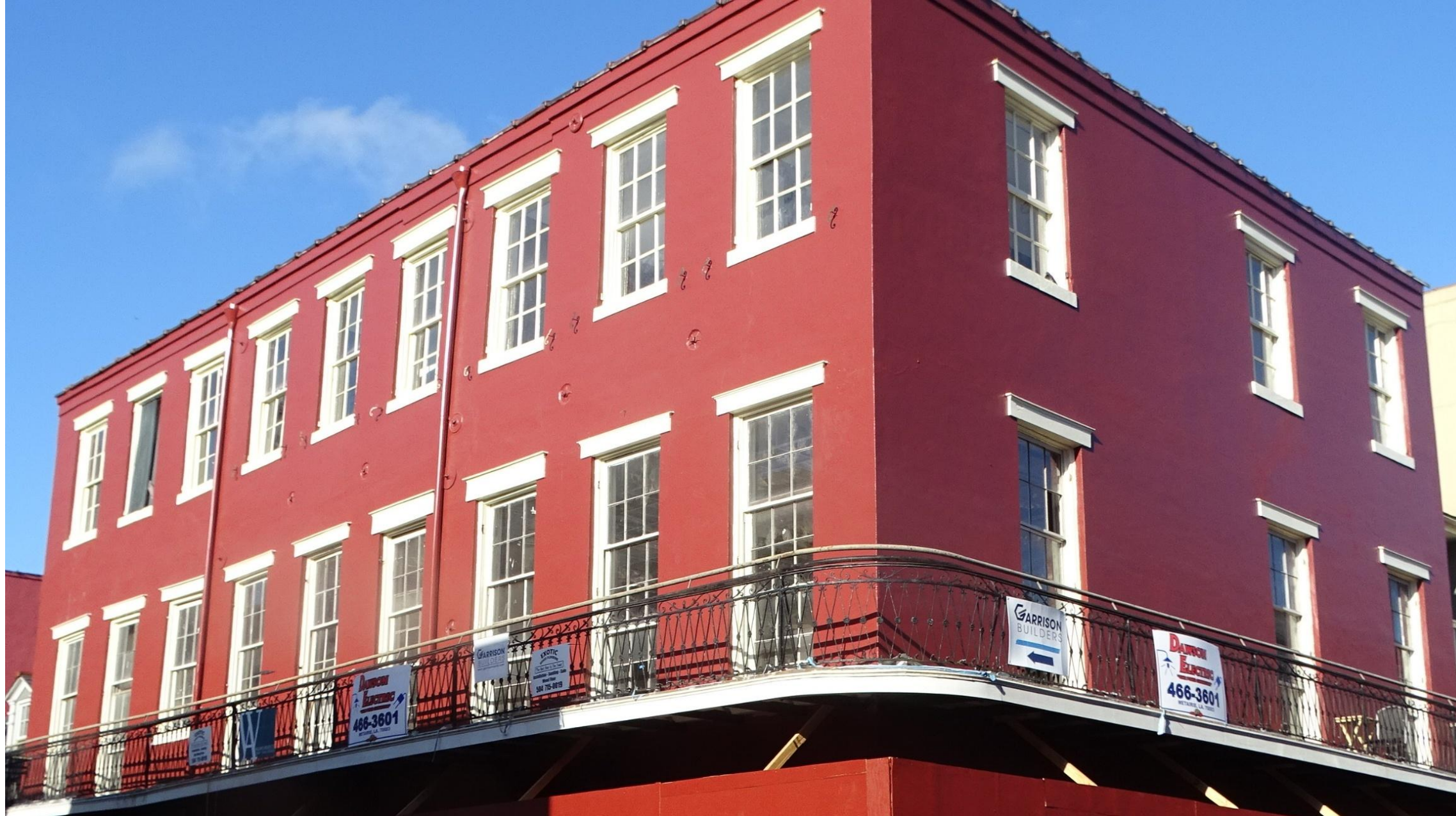
235-41 Bourbon – Prior to Window Replacement
