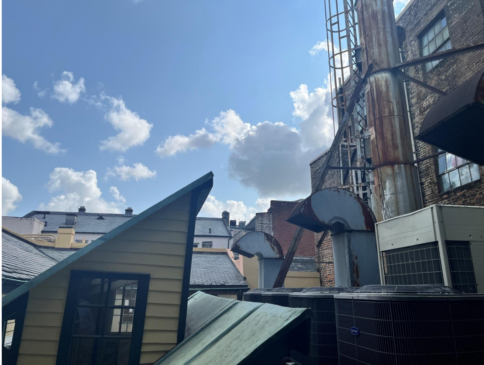
719 St. Louis – Area in need of rail
