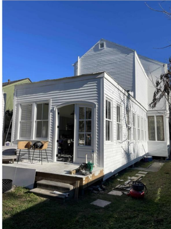
PHOTO B (EXISTING REAR ADDITION)
