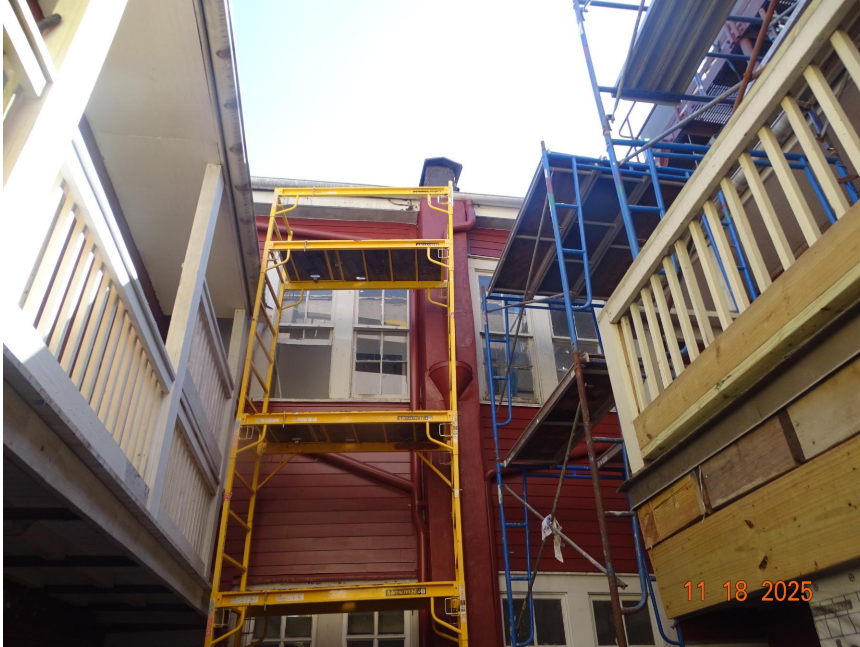
235-41 Bourbon – Courtyard Wall rebuilt and windows replaced
