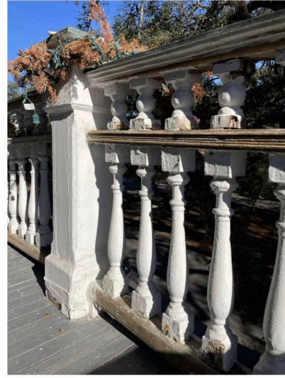
PHOTO C (EXISTING FRONT BALCONY RAIL)
