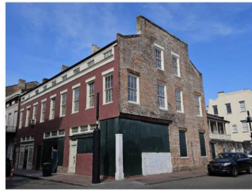
EXTERIOR PHOTO AT DAUPHINE & CONTI
