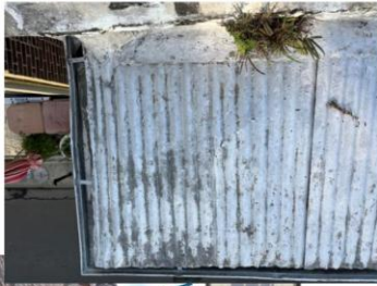
Existing awning roof (river side corner) from above.
