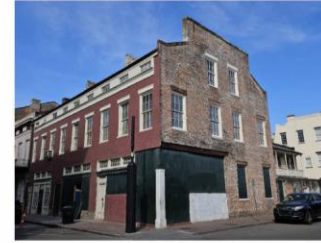
EXTERIOR PHOTO AT DAUPHINE & CONTI
