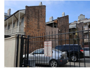
EXTERIOR PHOTO AT REAR
