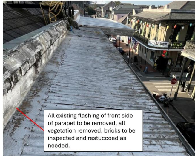
Replace existing corrugated metal porch roof to match existing. Roof dimension=32ft. X 4ft. Use 24 ga. Galvalume standing seam metal roof.
