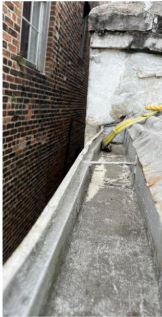
River side corner of awning gutter and partial downspout.
