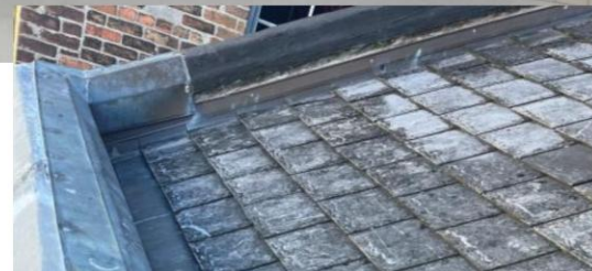
Profile of roof parapet showing location of flashing.
