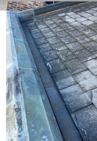
Profile of roof parapet showing location of flashing.
