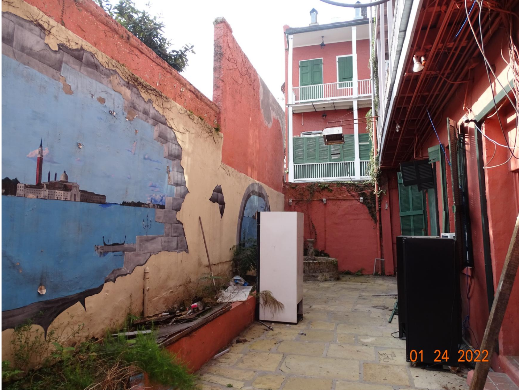
730-732 St Peter – previous conditions
