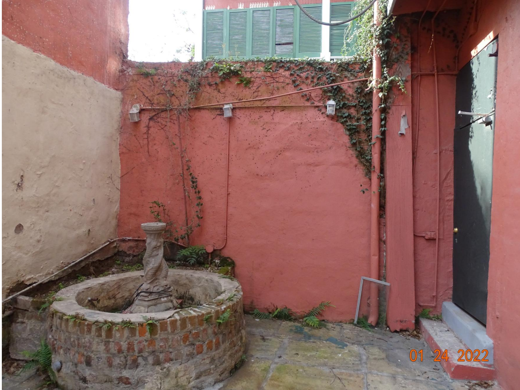
730-732 St Peter – previous conditions
