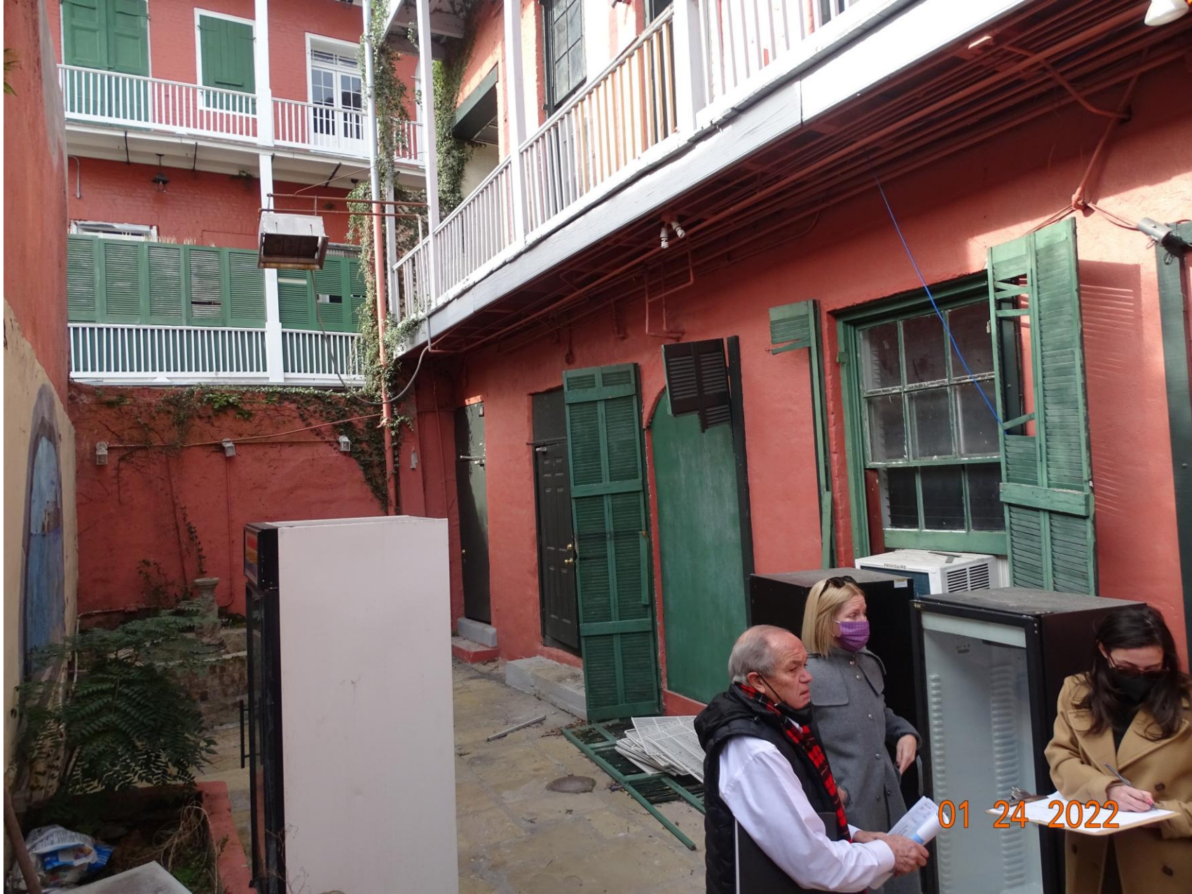
730-732 St Peter – previous conditions
