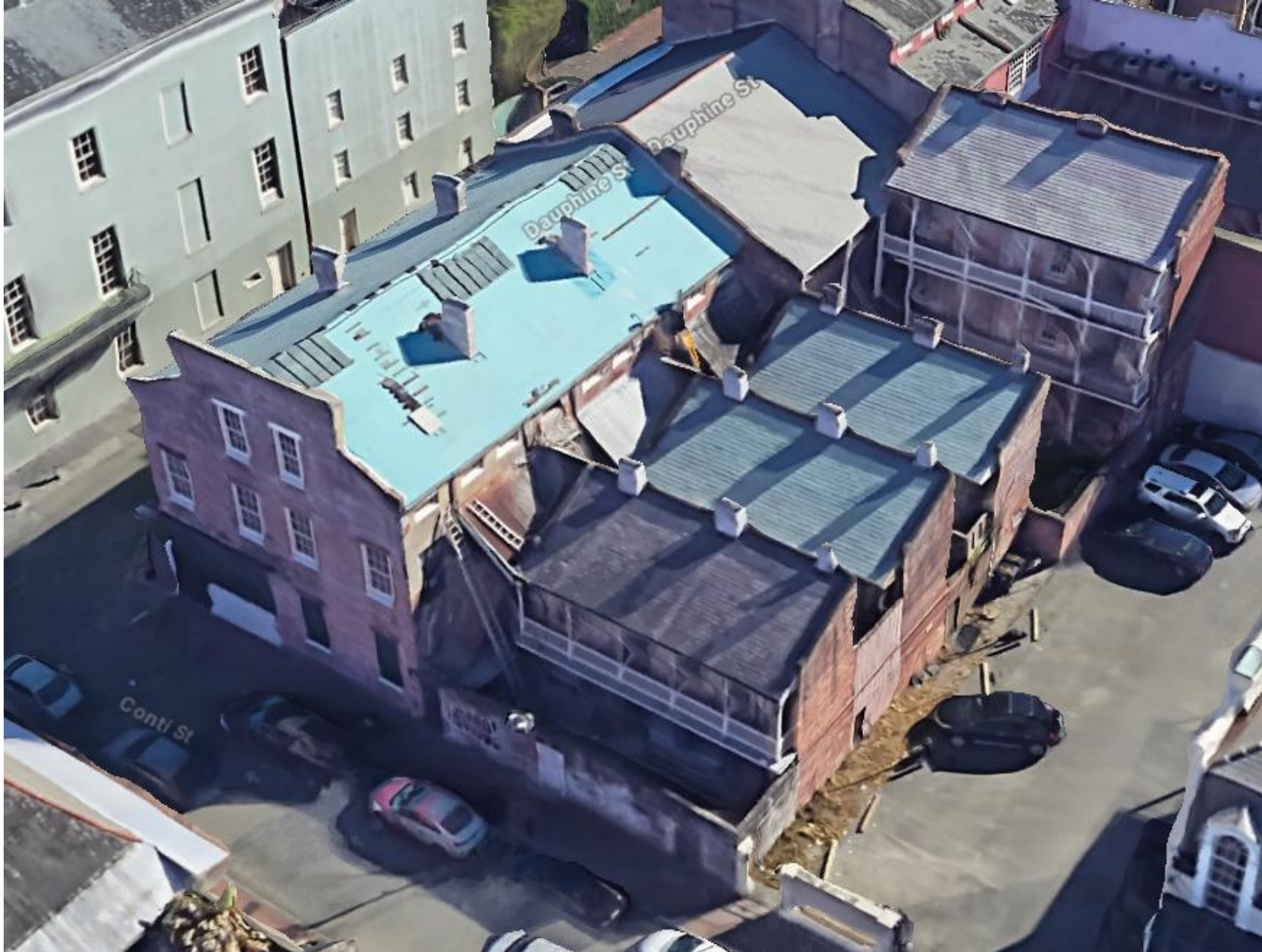
335 Dauphine – Rear Property Line Wall
