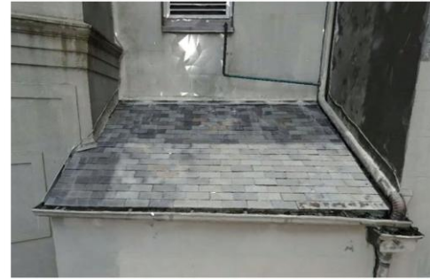
39 NE CHAPEL ROOF
