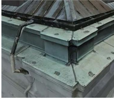
35 MAIN STEEPLE - GUTTER
