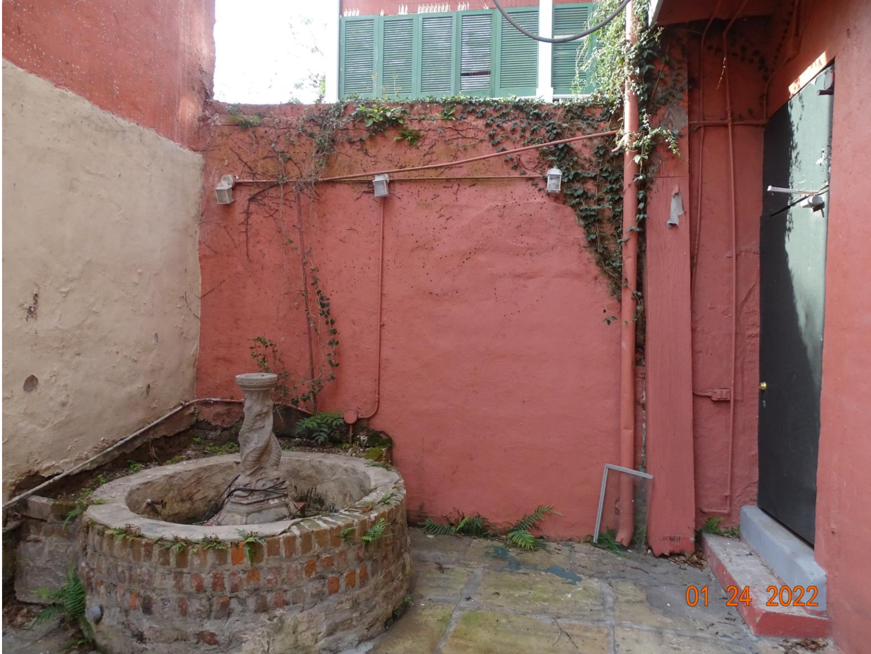
730-732 St Peter – previous conditions
