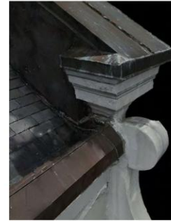
37 MAIN ROOF - GUTTER
