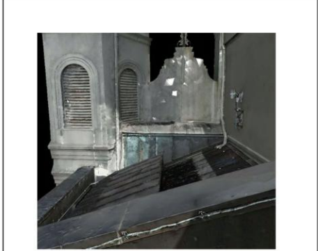
32 COOLING TOWER ROOF (N)
