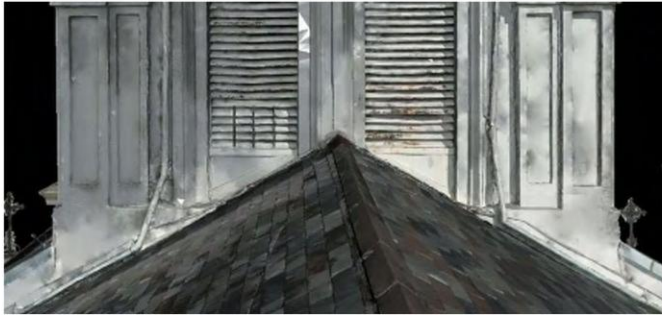
38 MAIN ROOF - STEEPLE BASE (W)
