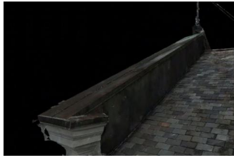
41 MAIN ROOF - PARAPET (W)
