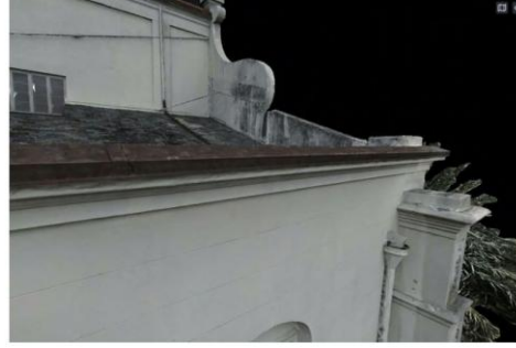
36 EXISTING REAR SIDE PARAPET
