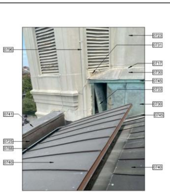
28 CHILLER ROOF - ACCESS PANEL HEAD
